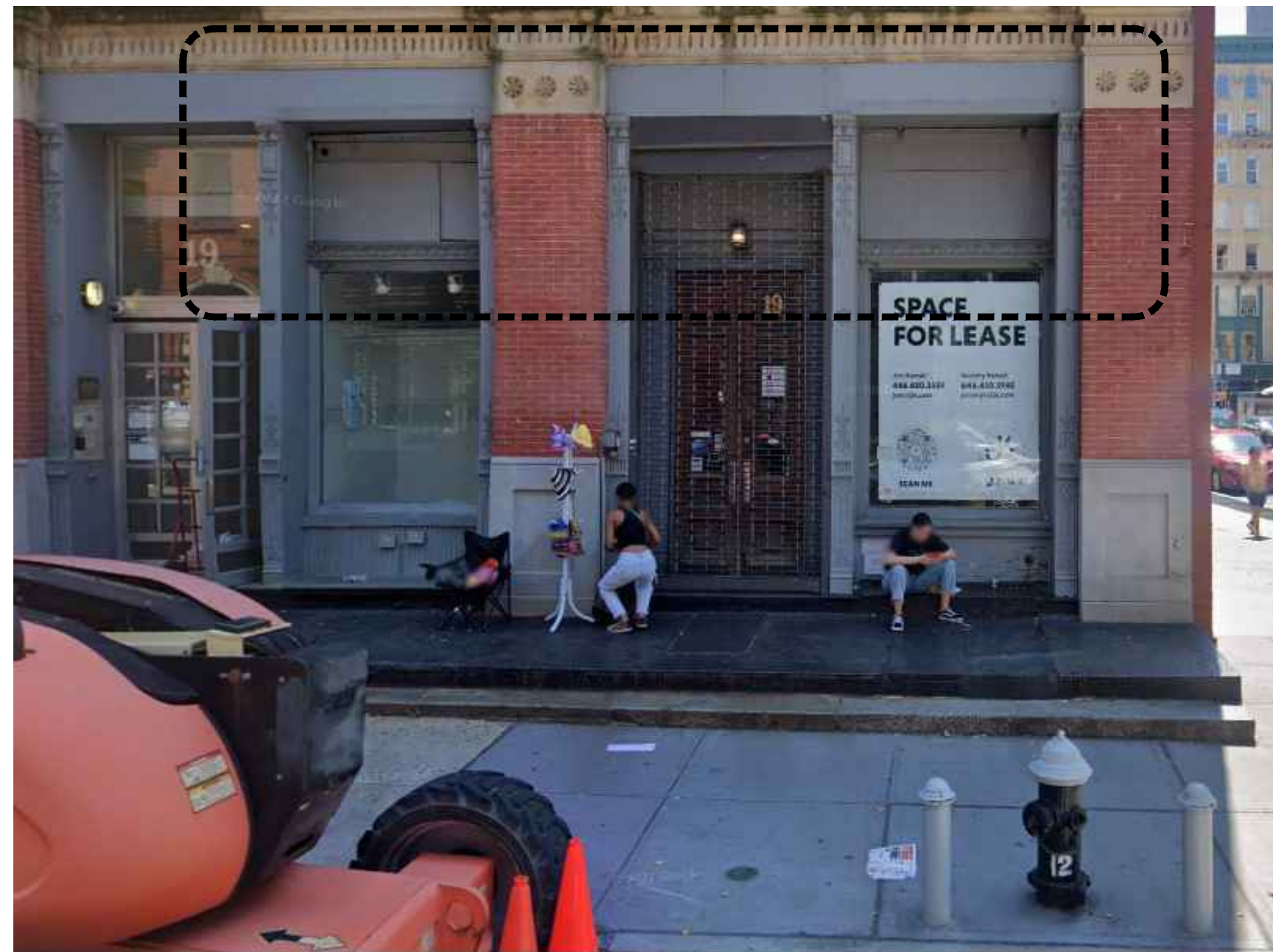
2 LOCATION #1 : VIOLATION - 160322 REMOVED A-005 SCALE: N/A
