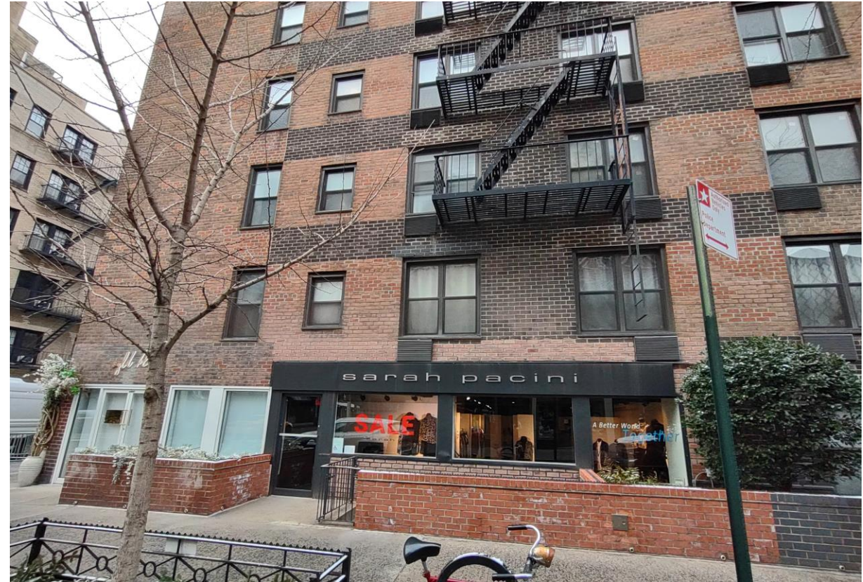
Partial Bleecker Street elevation. Storefronts at the southern end of the façade.
