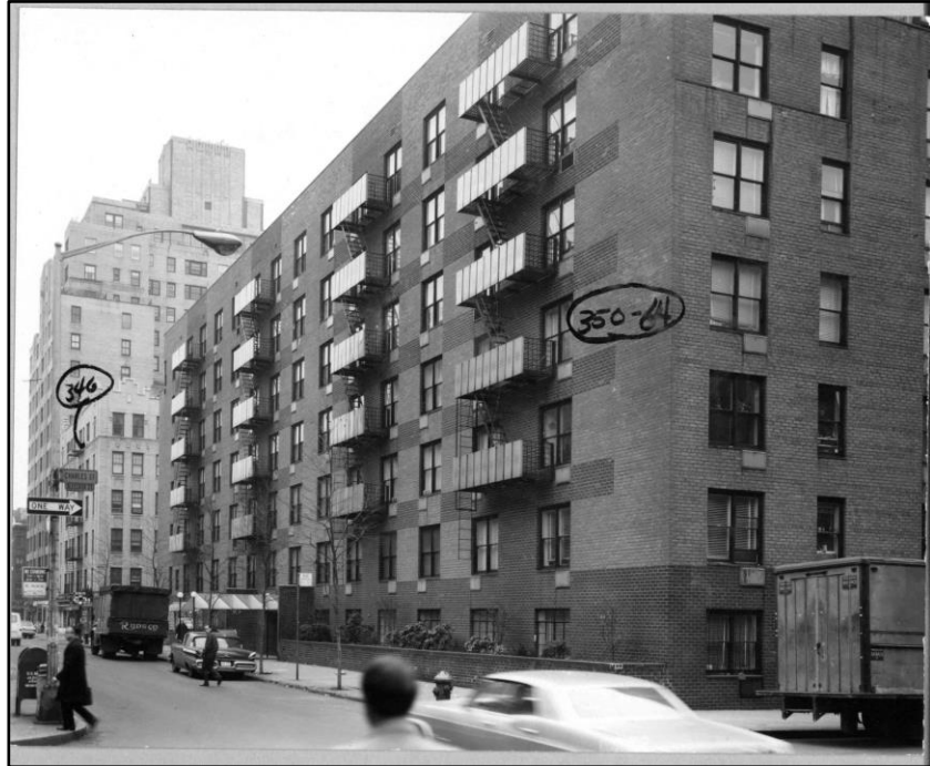
1969 Designation Photo, looking south on Bleecker Street from Charles Street. (NYC LPC)
