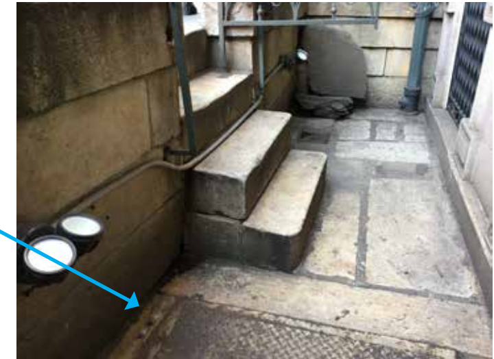
Areaway Looking West
