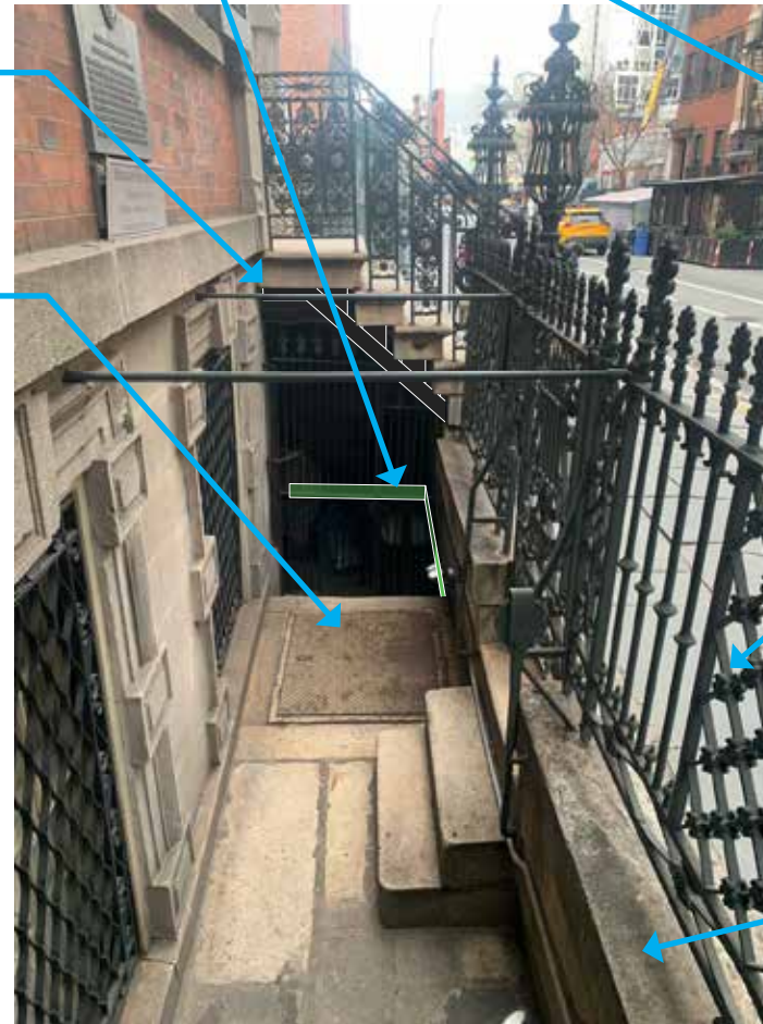
Areaway Looking East
