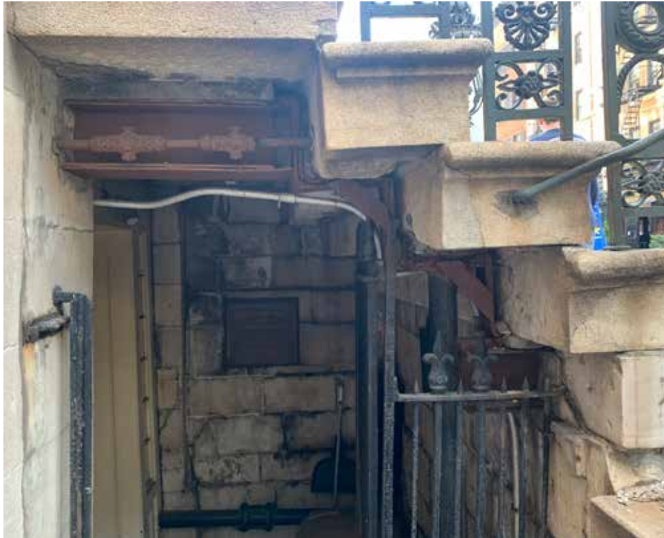
10 - Existing Stair Support Looking East
