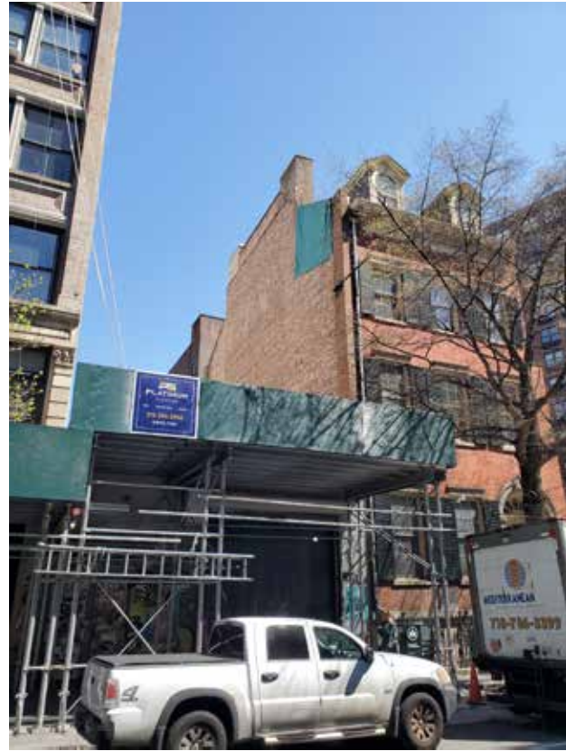
West and South Facades
