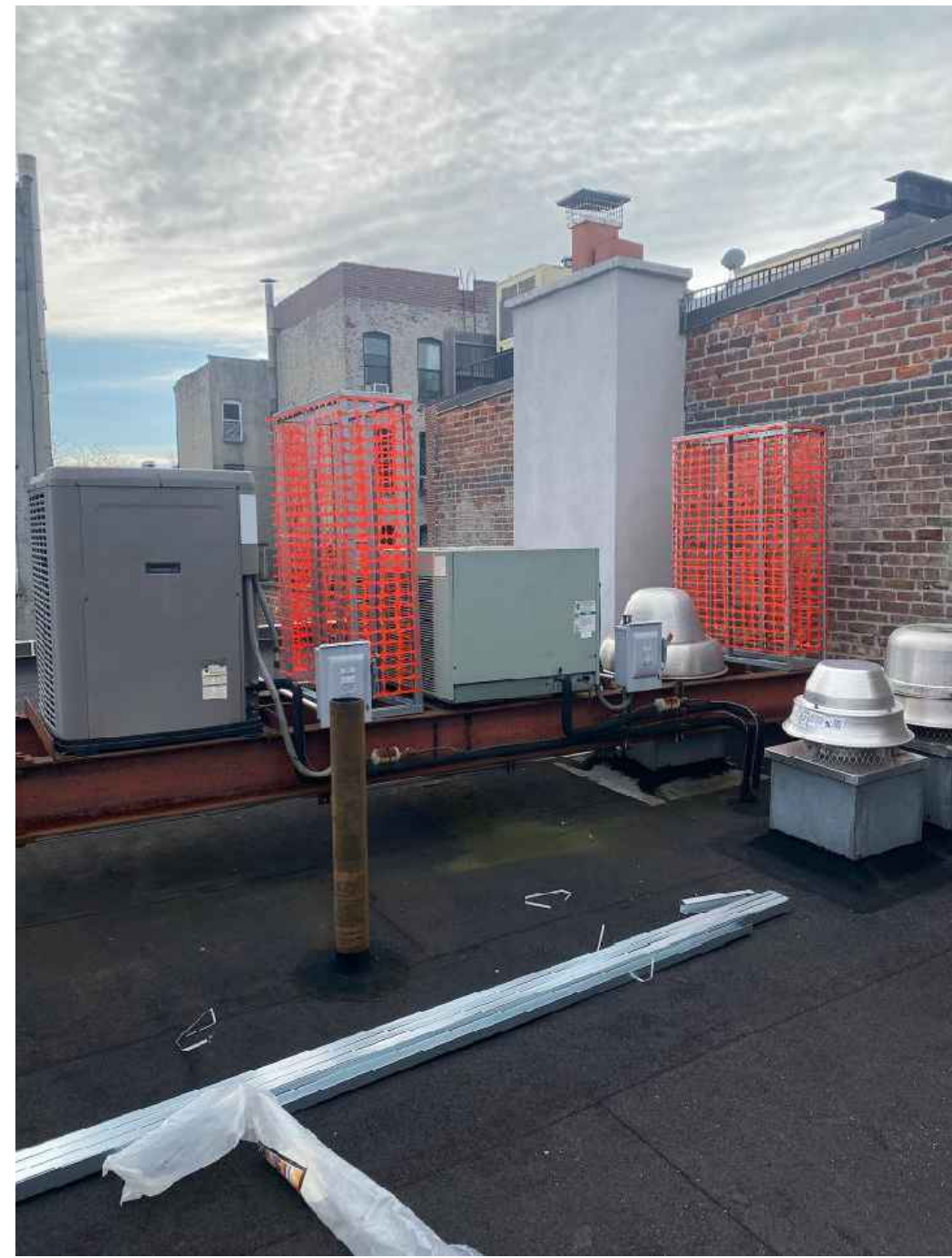
3- VIEW SOUTH ON ROOF
