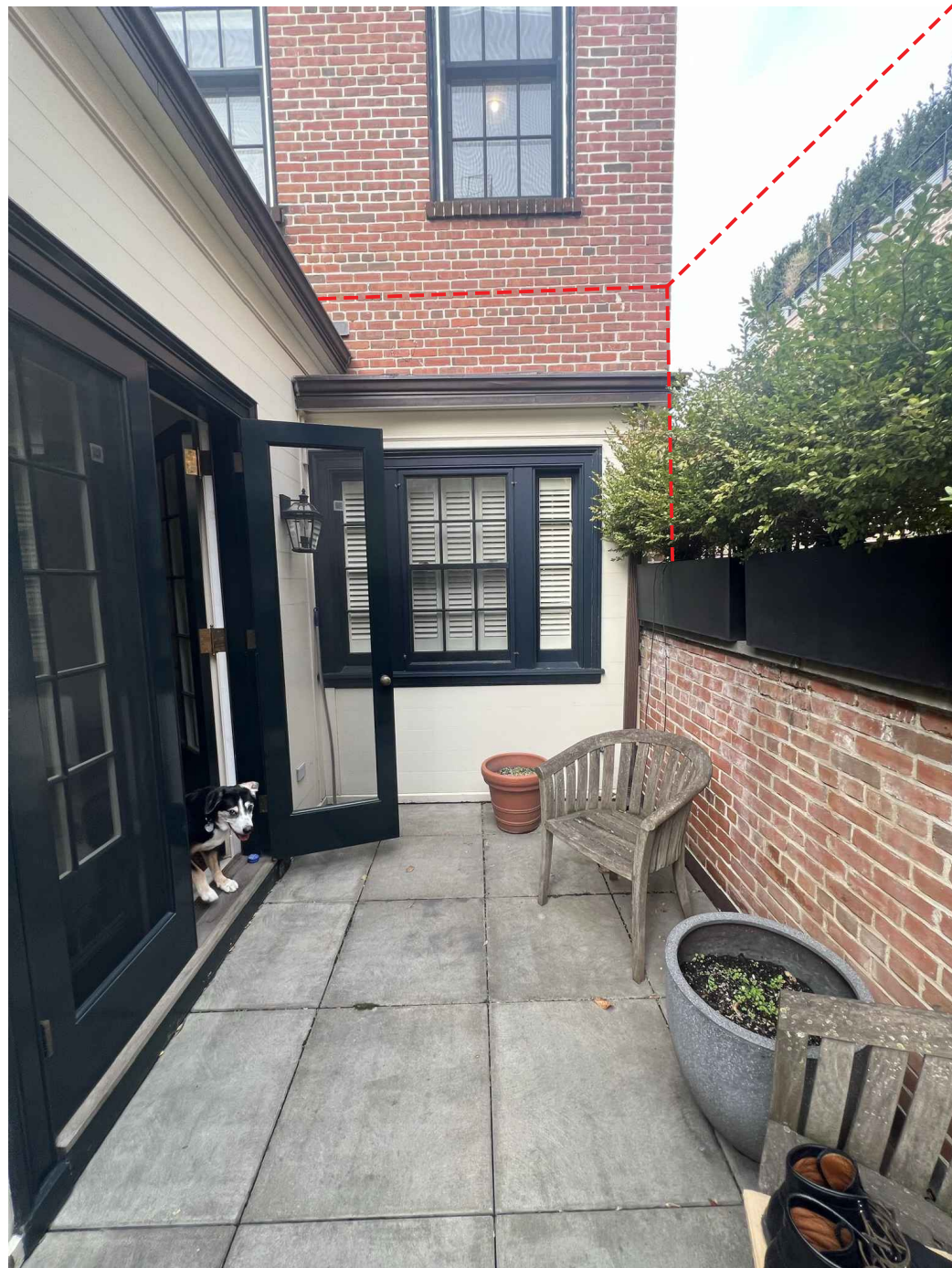
1- VIEW NORTH AT 2ND FLOOR TERRACE
