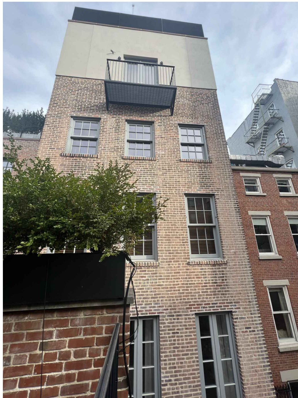
2- VIEW EAST AT 2ND FLOOR TERRACE
