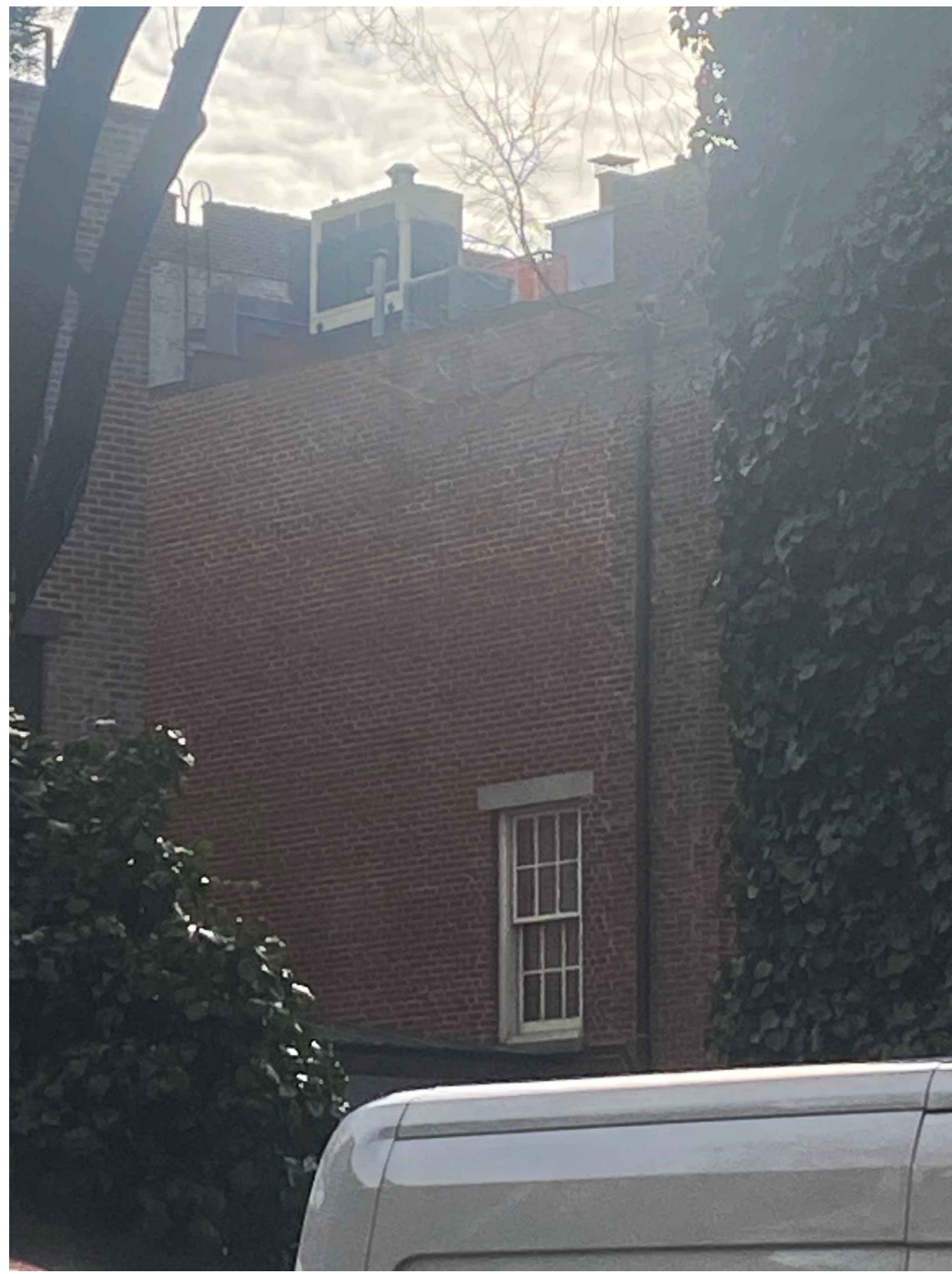
2- VIEW FROM W11TH STREET
