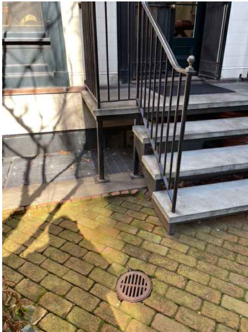
1- STAIR TO YARD
