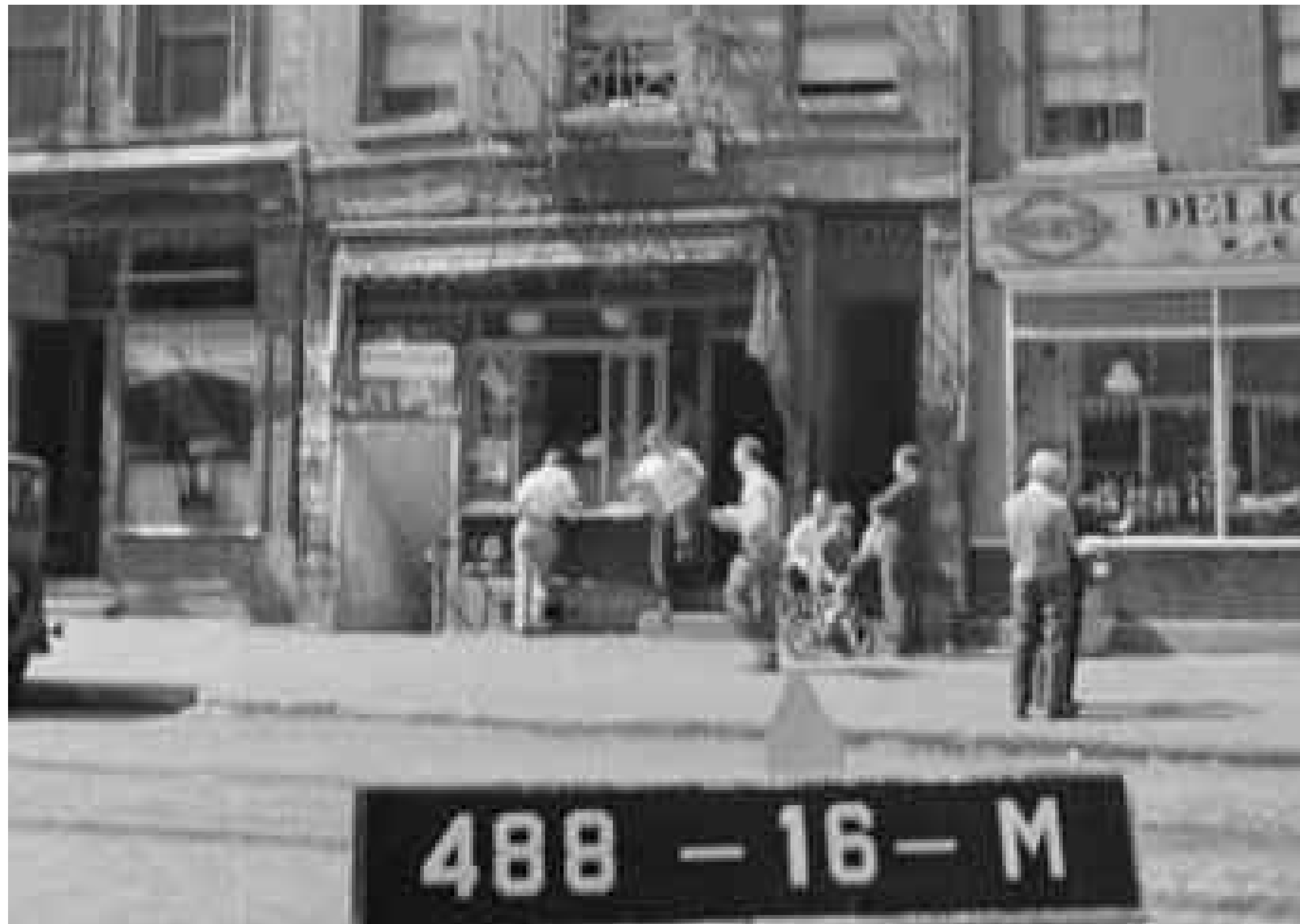
EXISTING CONDITION OF STOREFRONT
