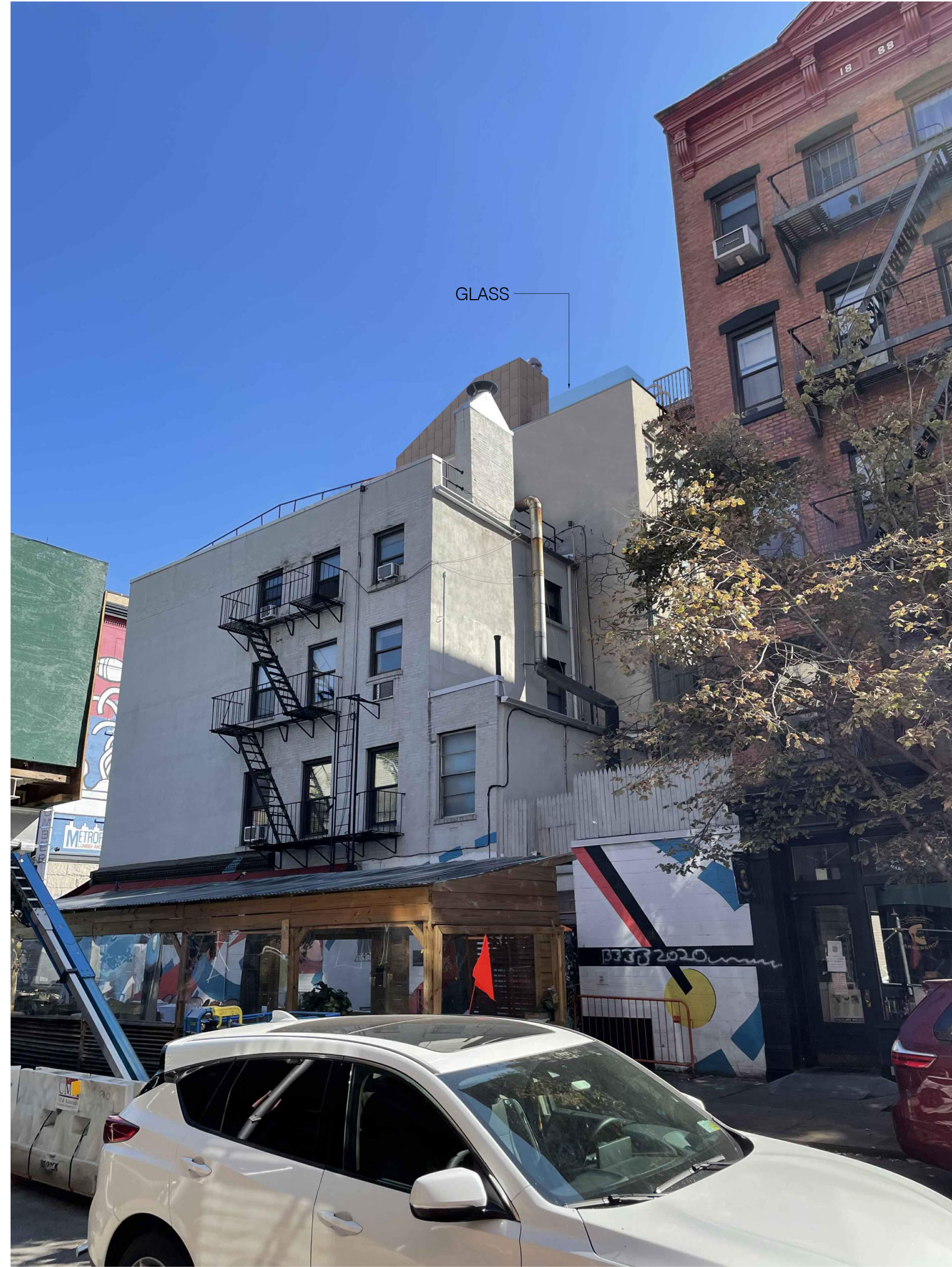
02 SIDE & REAR FACADE PHOTO MONTAGE N.T.S.
