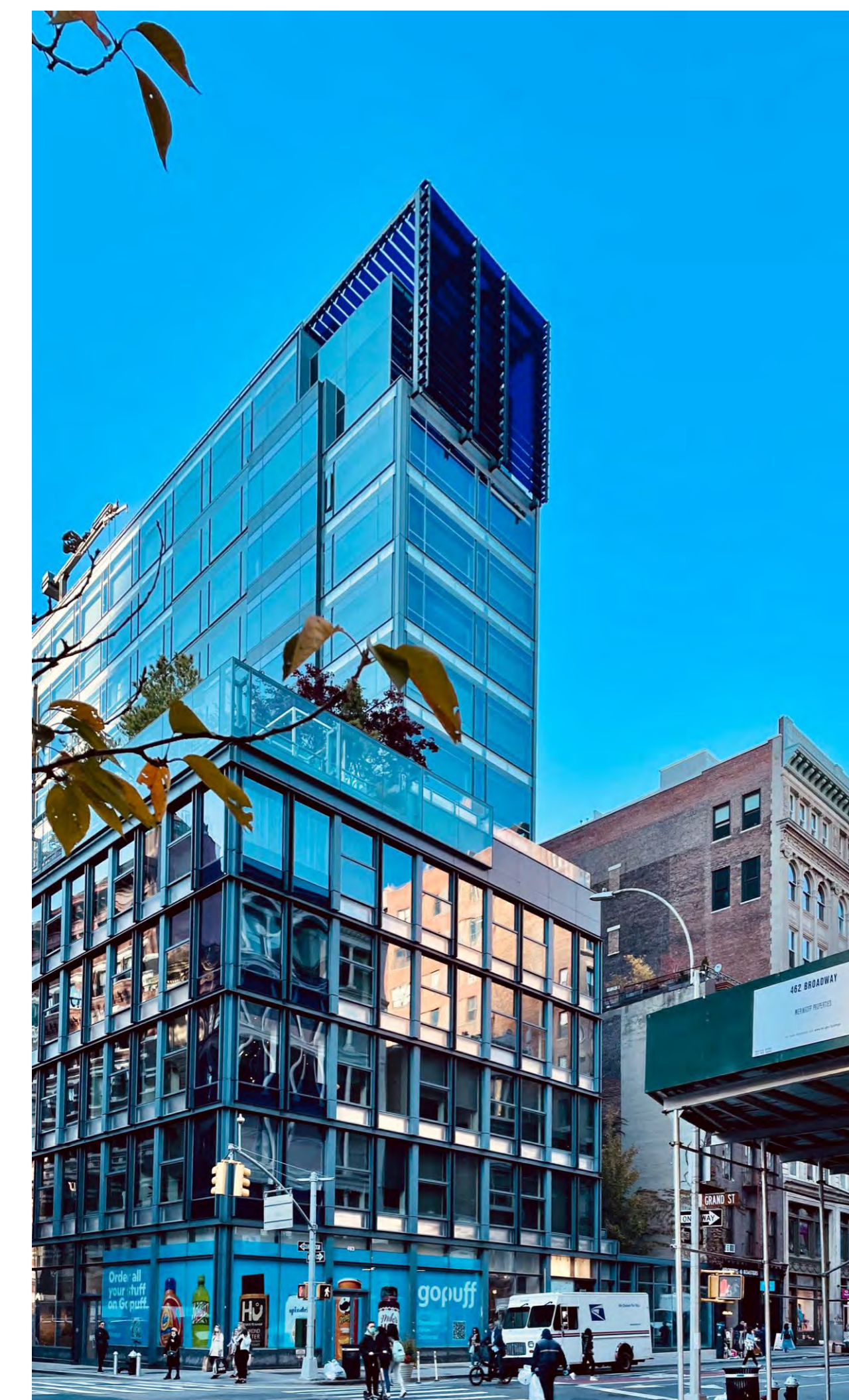
2. VIEW FROM GRAND STREET
