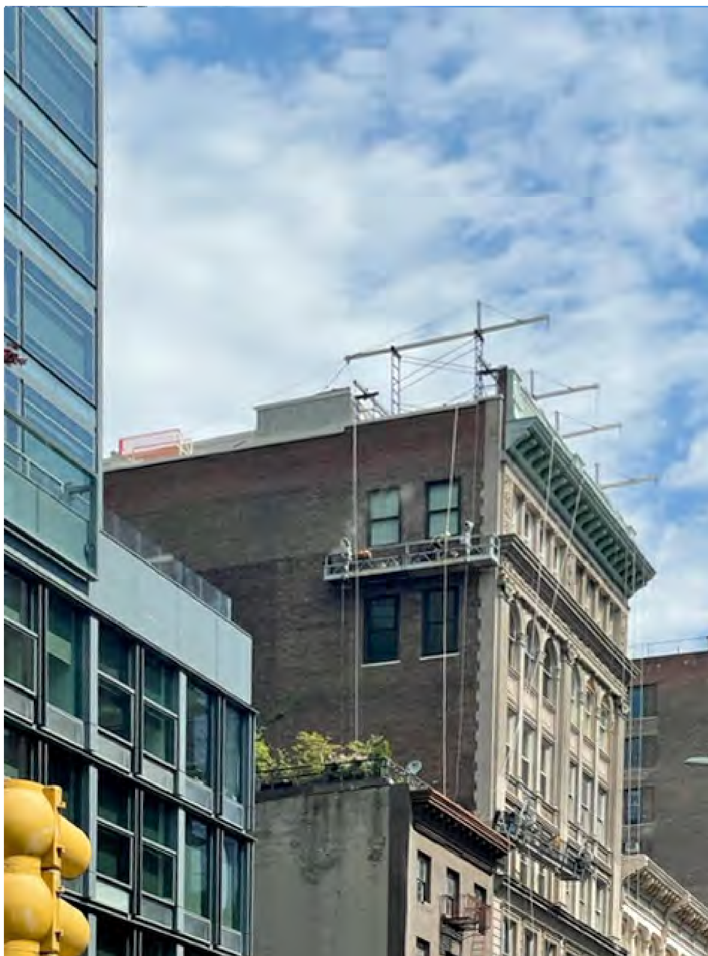
VIEW 2, MOCK-UP OF NEW EXHAUST ENCLOSURE
