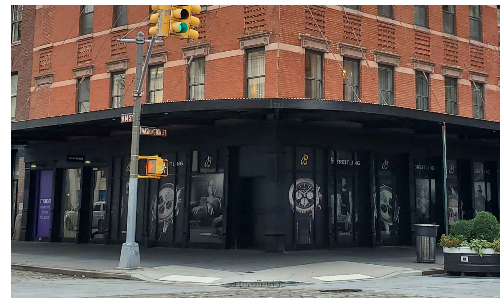
2 NORTH-WEST CORNER - STREET VIEW NTS
