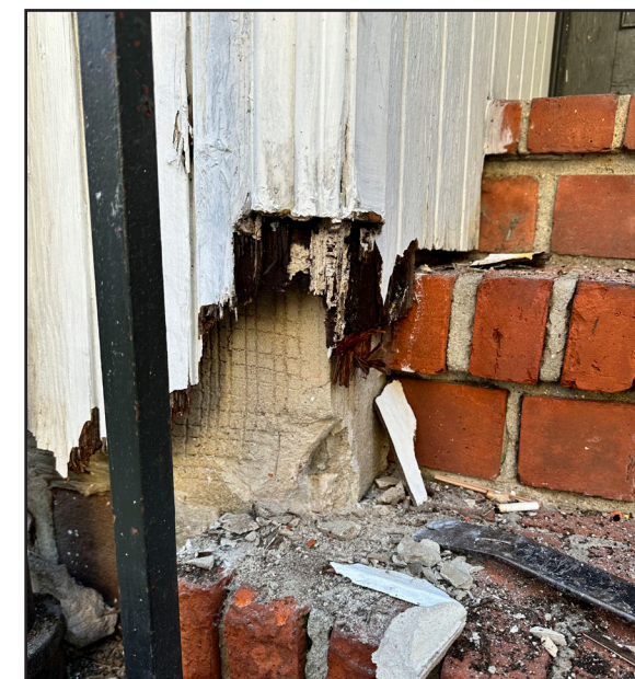
WOOD CLADDING PROBE REVEALING CEMENT INFILL
