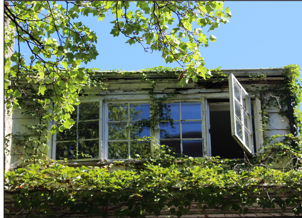
ATTIC DORMER AND CASEMENT WINDOWS
