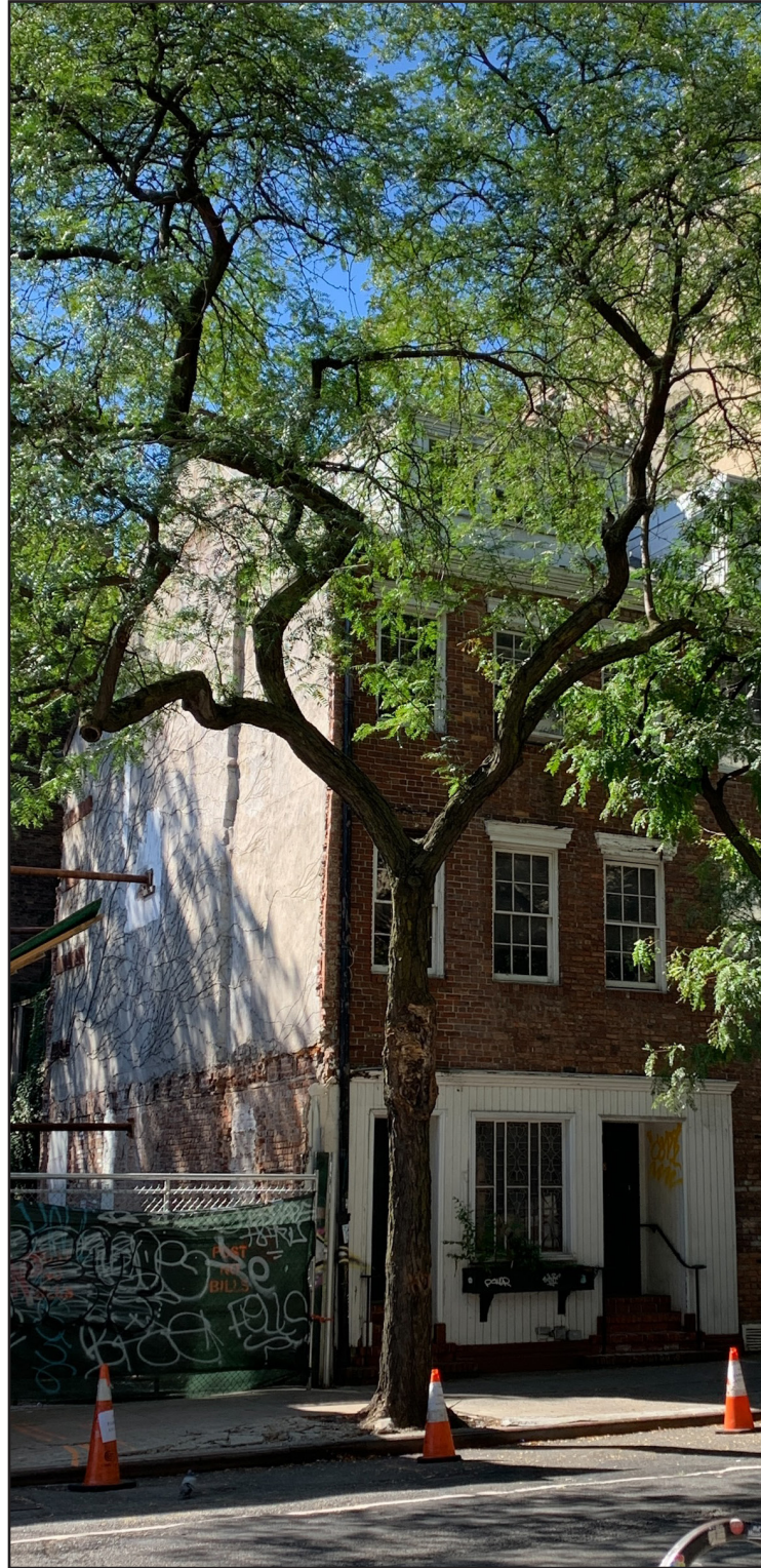
PHOTO 1 FRONT VIEW LOOKING SOUTHWEST
