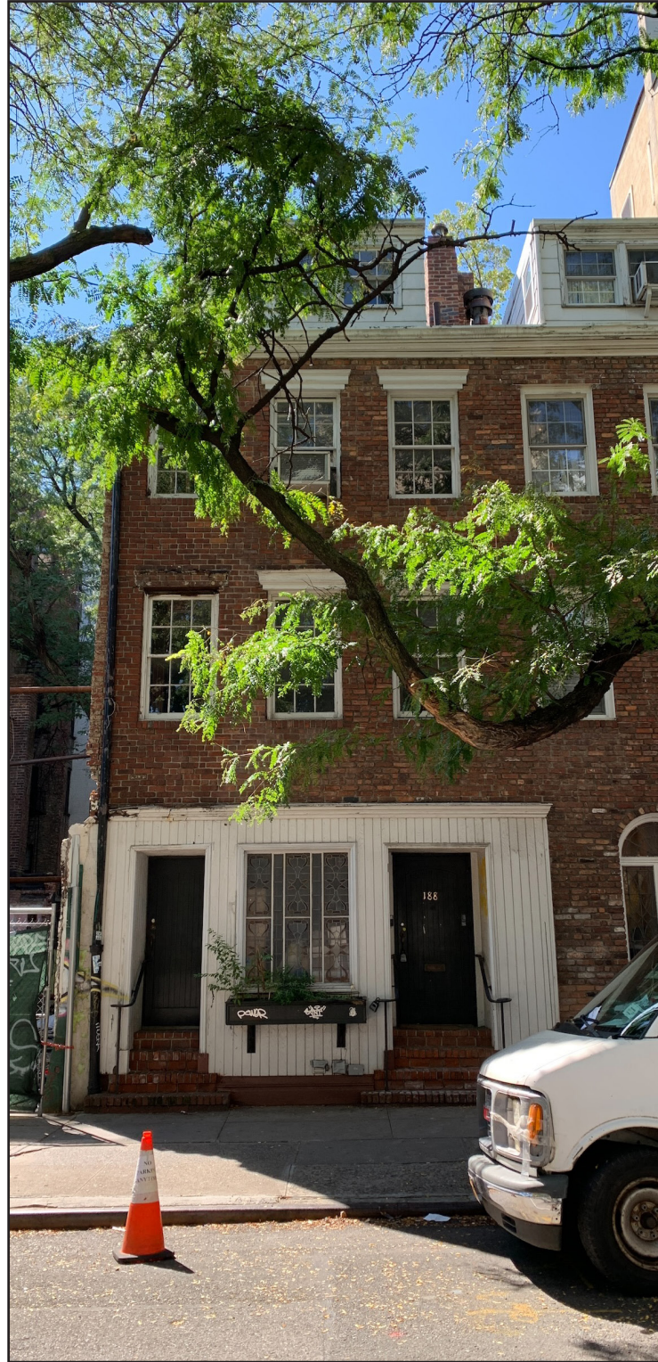
PHOTO 2 FRONT VIEW LOOKING SOUTH
