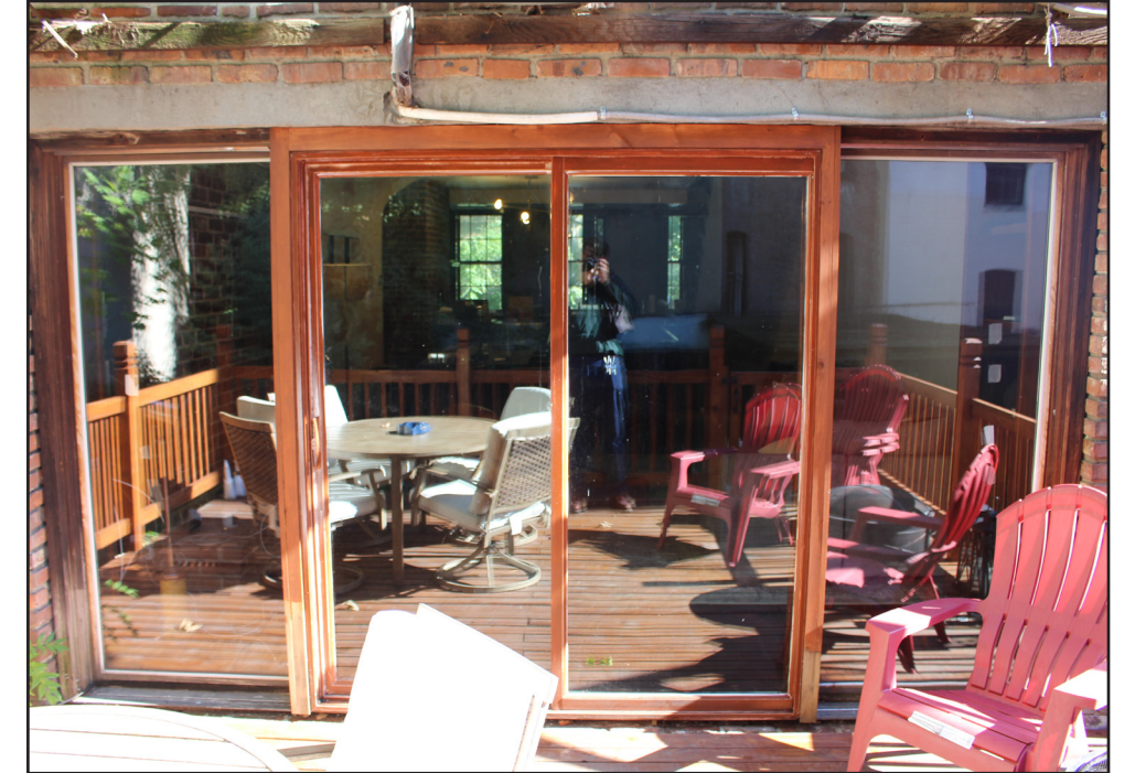
SECOND FLOOR GLAZING
