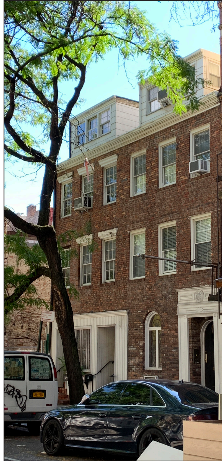
PHOTO 3 FRONT VIEW LOOKING SOUTHEAST
