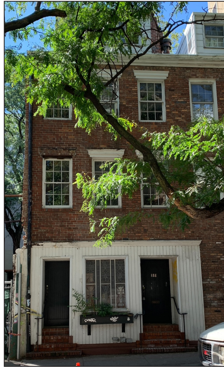
188 SPRING ST EXISTING FRONT FACADE
