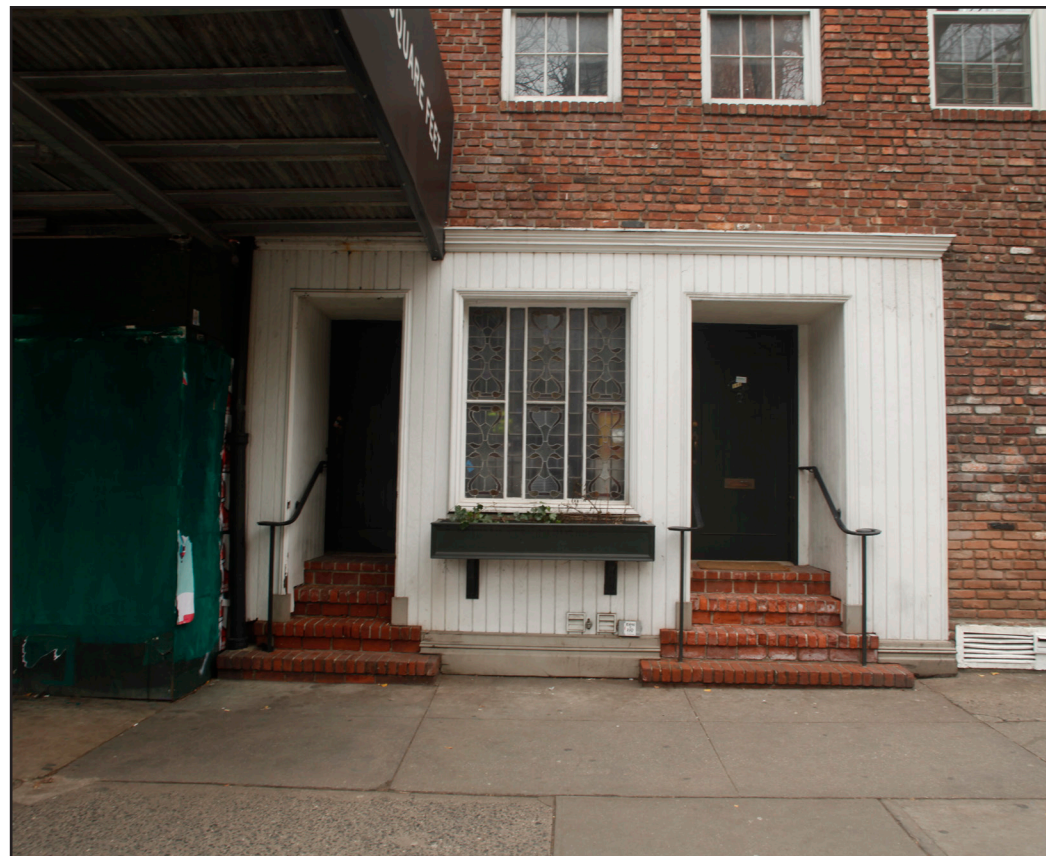
LPC - DESIGNATION PHOTO
