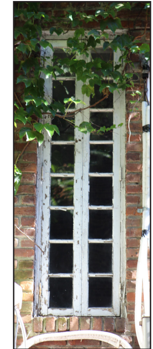
THIRD FLOOR DOUBLE CASEMENT WINDOWS
