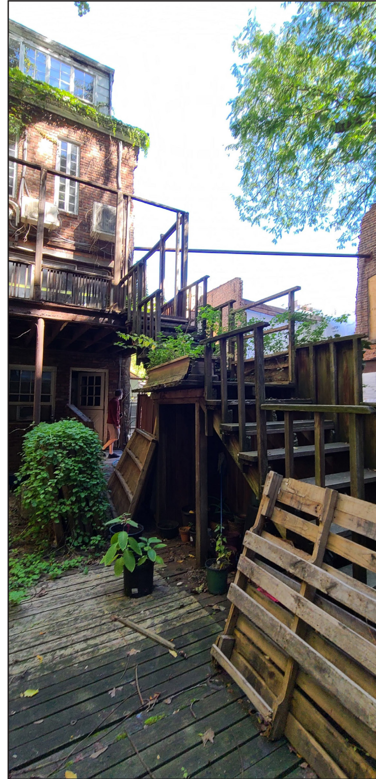
PHOTO 3 REAR VIEW LOOKING NORTHEAST
