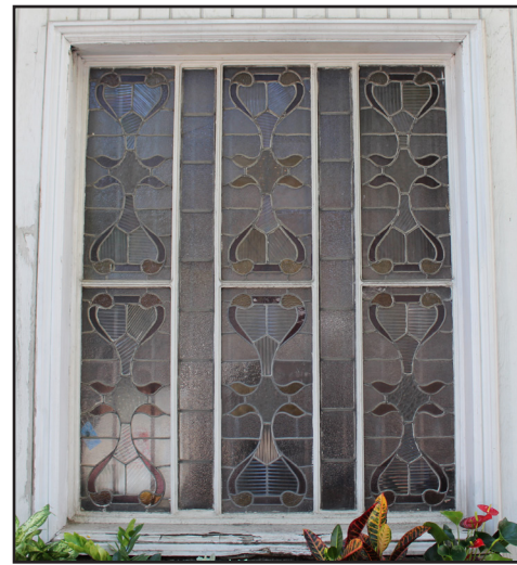
1960s FIRST FLOOR FIXED STAINED GLASS WINDOW
