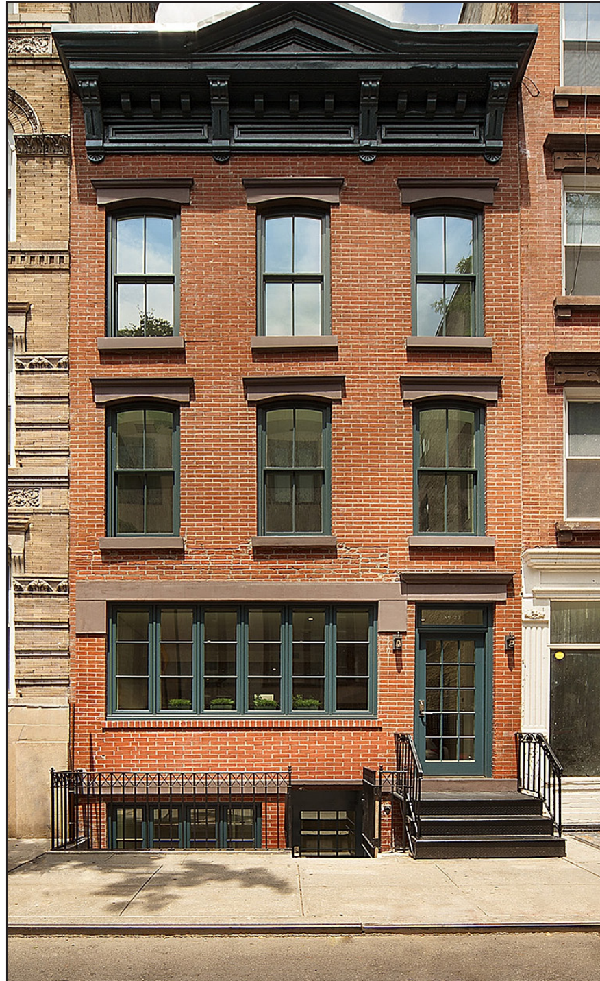
23 DOWNING ST | LPC 12-6737 ALTERED RENAISSANCE REVIVAL
