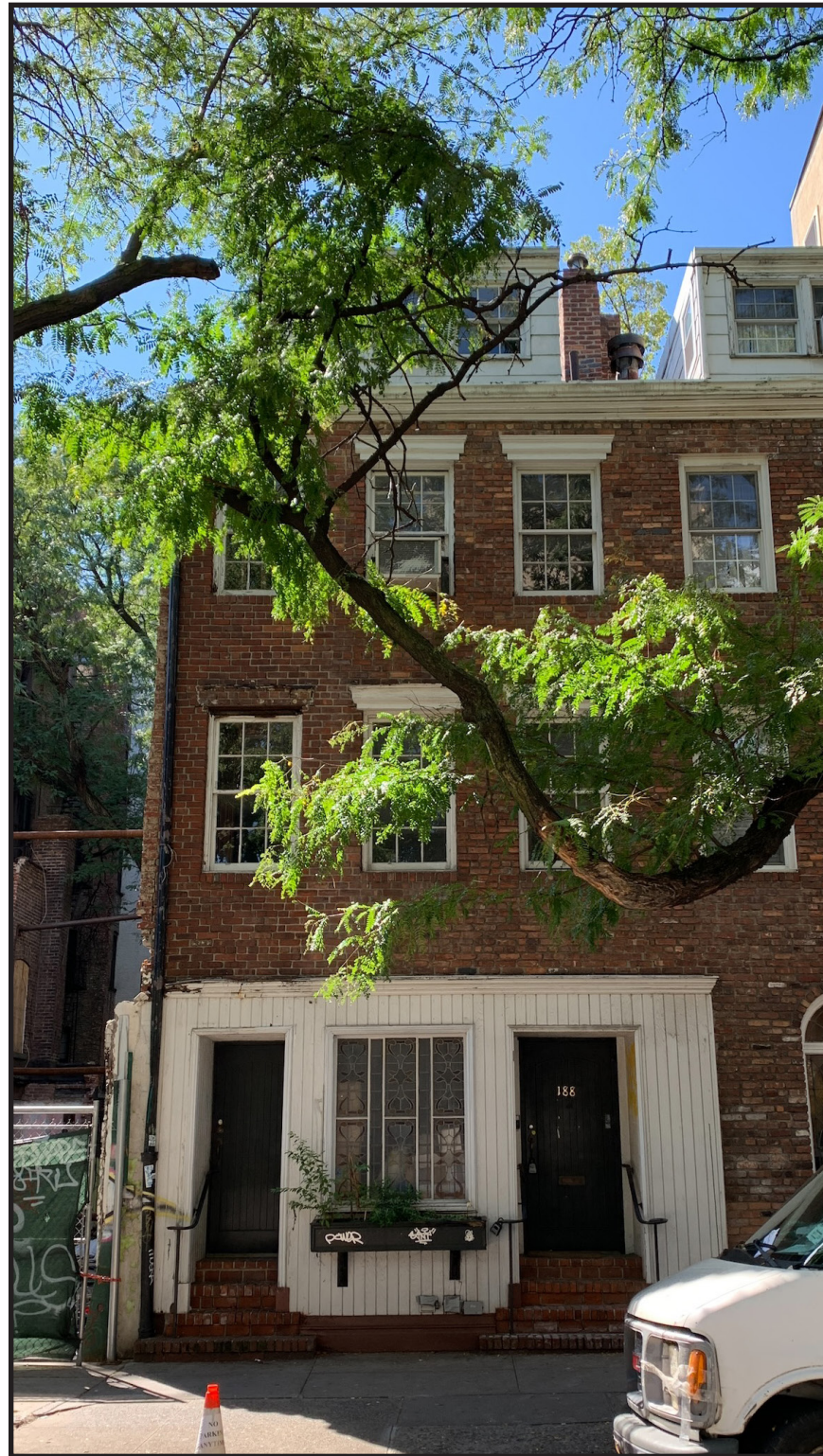
EXISTING FRONT FACADE
