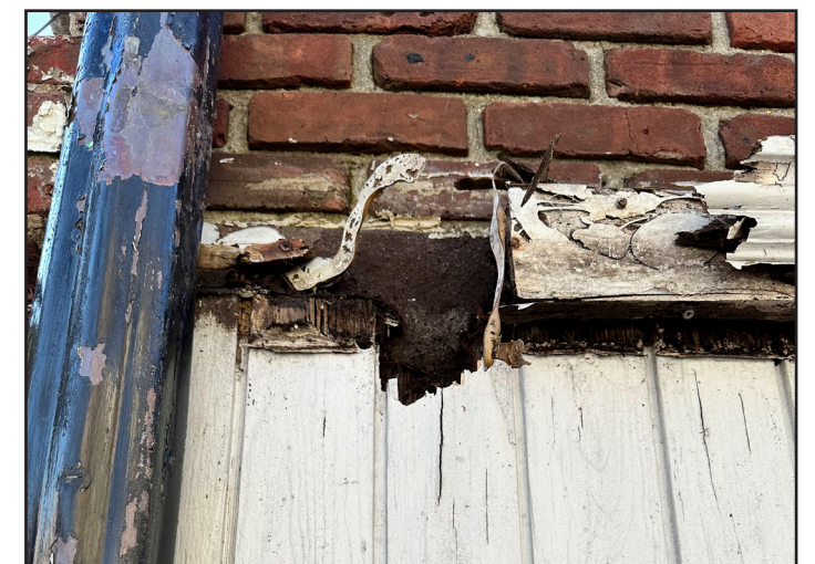
WOOD CLADDING PROBE REVEALING ORIGINAL BROWNSTONE LINTEL
