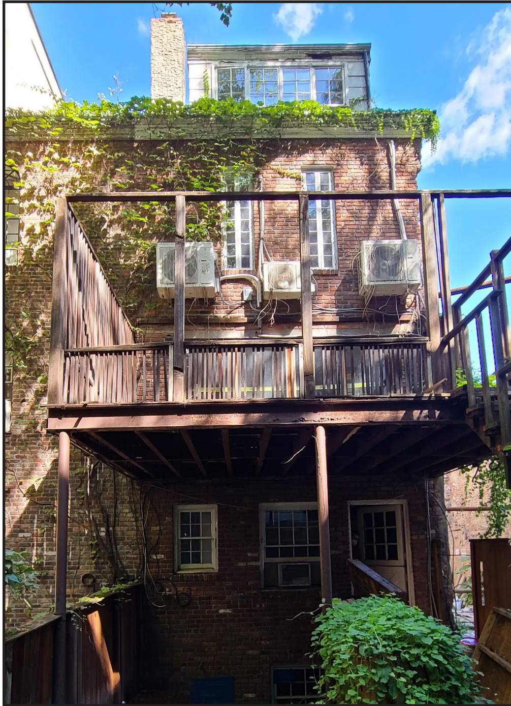
188 SPRING ST EXISTING REAR FACADE ALTERED FEDERAL STYLE
