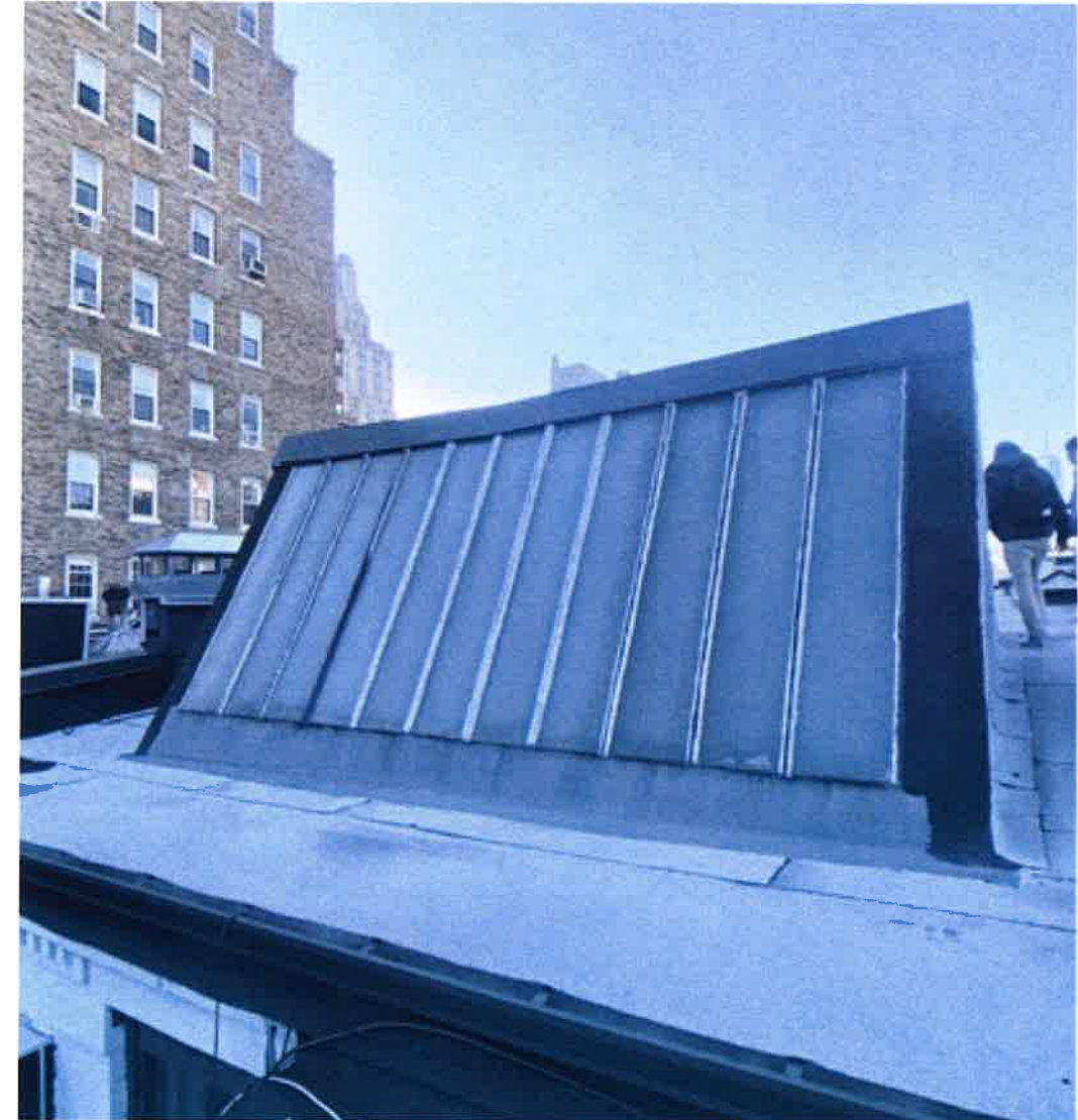
Skylight View Looking South
