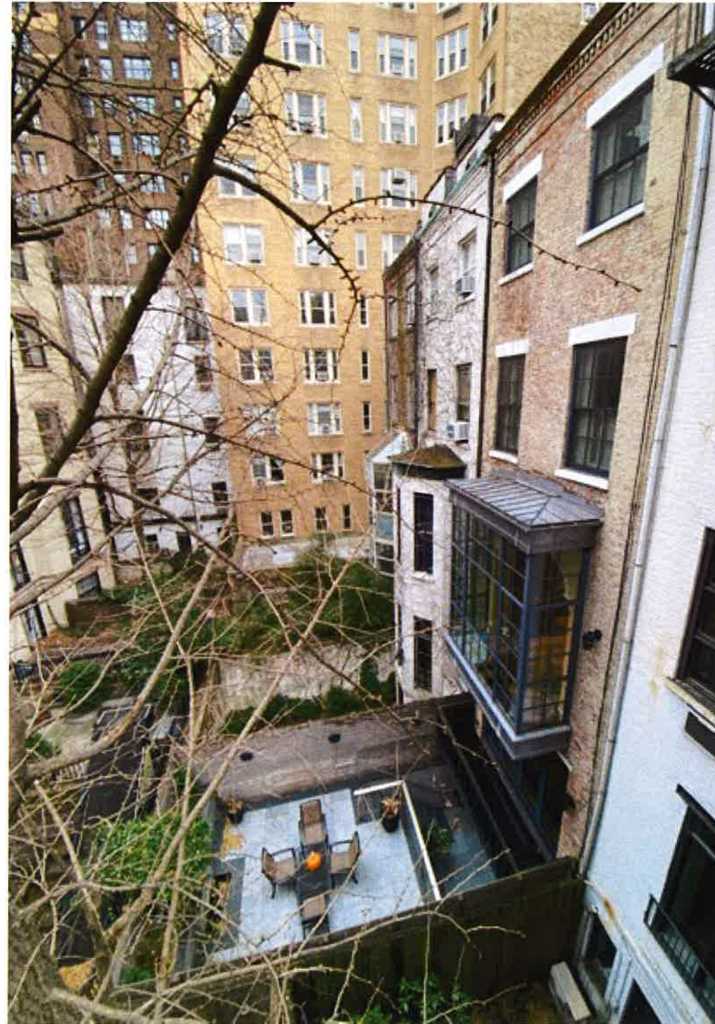
Context: Rear Yard Looking West
