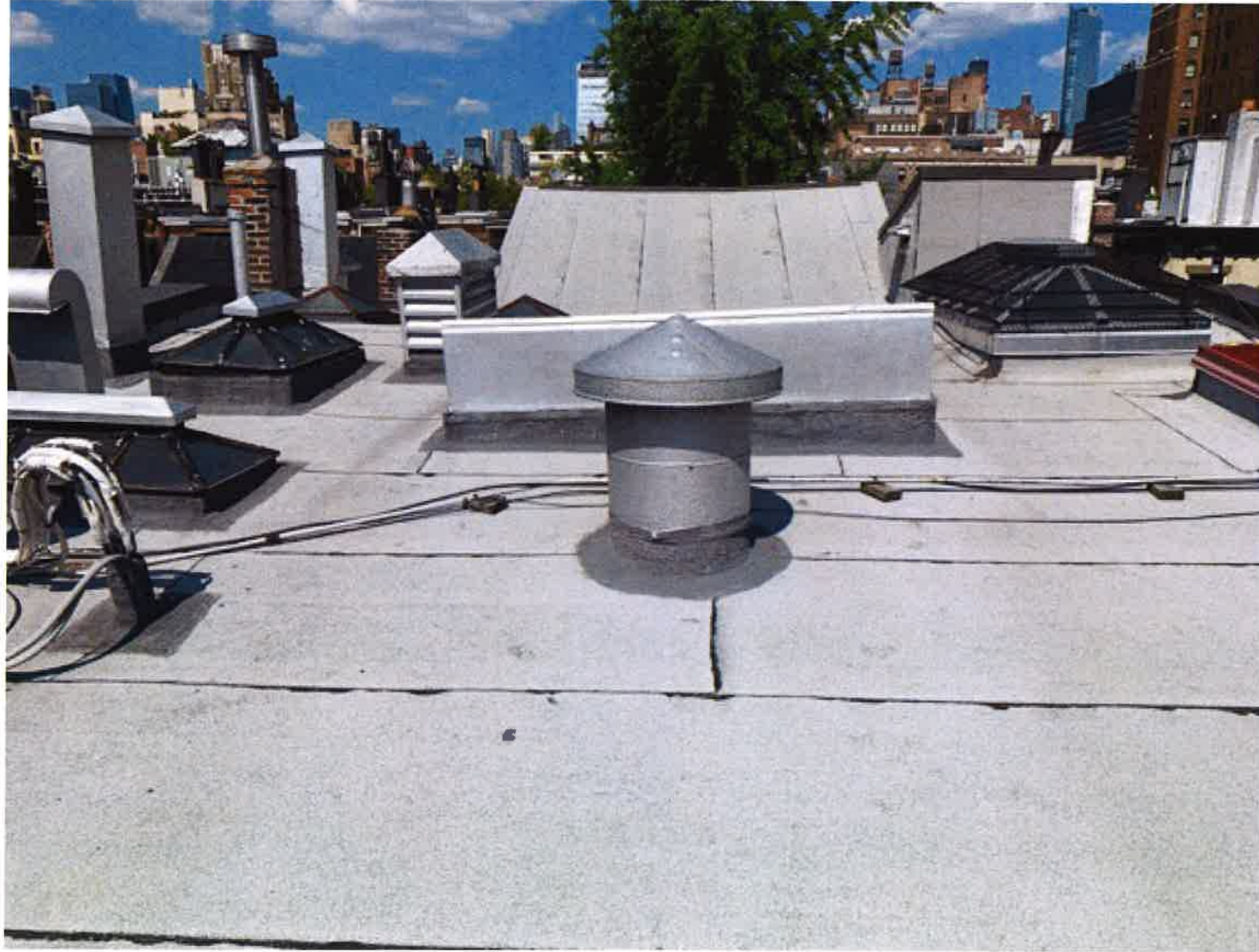
Skylight View Looking North
