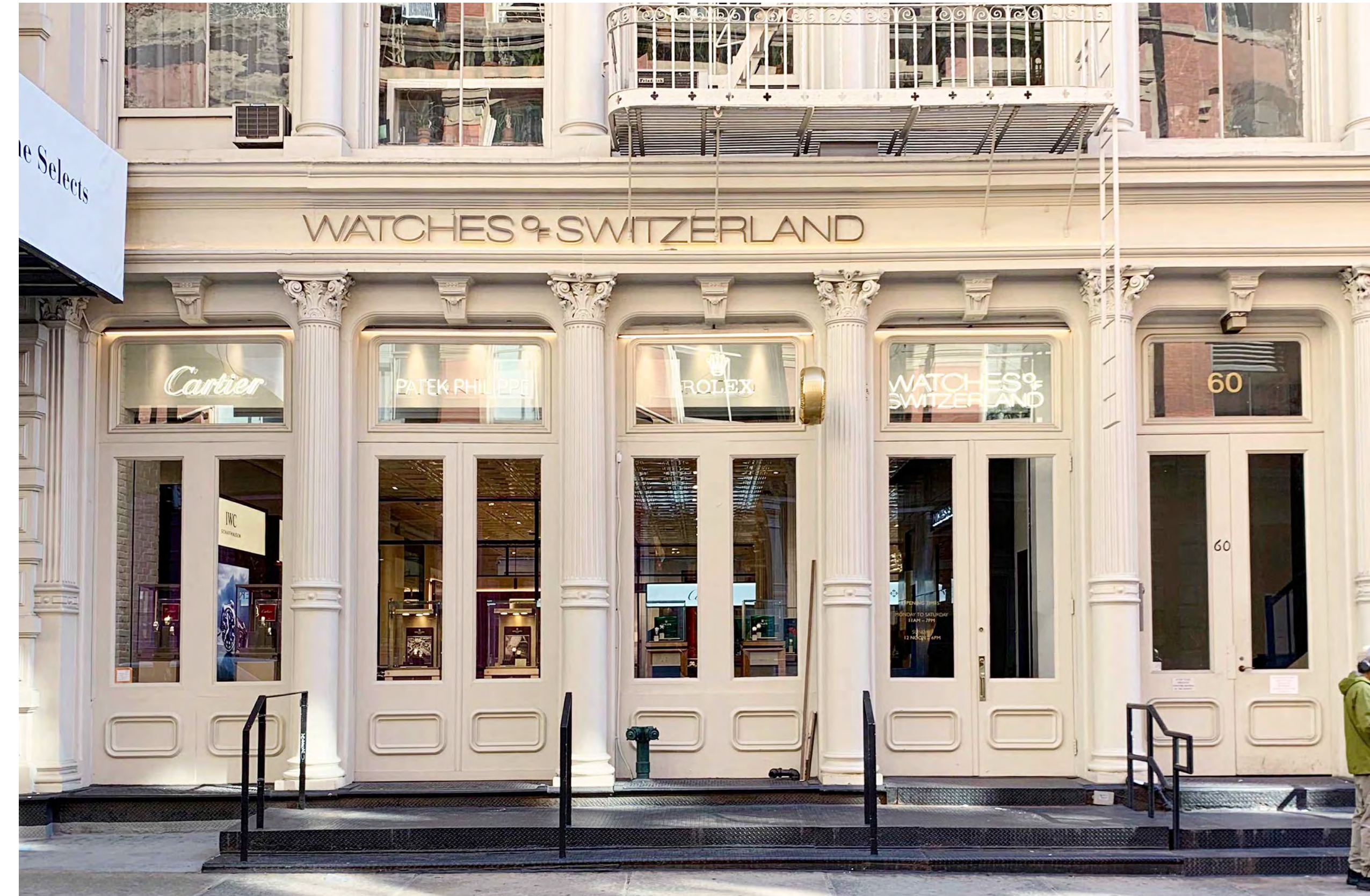
BAY 01 ORIGINAL CAST IRON BASE BAY 02 FIXED WOOD DOORS BAY 03 ORIGINAL CAST IRON BASE BAY 04 WOOD ENTRY DOORS (RETAIL) BAY 05 WOOD ENTRY DOORS (RESIDENT)
