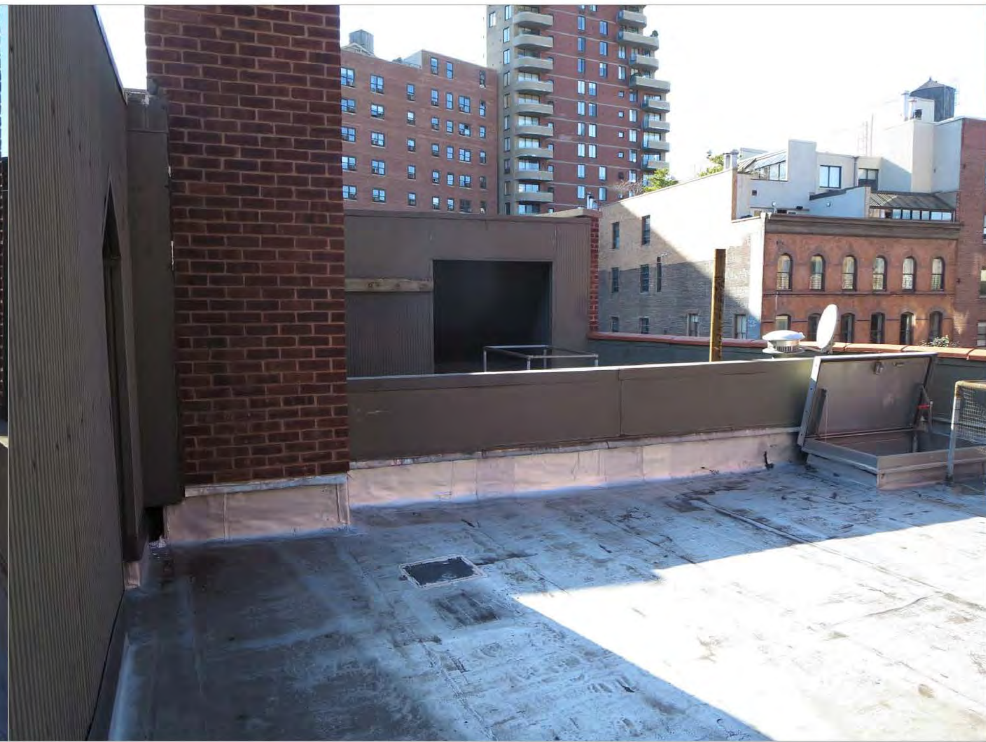
2 ROOF LOOKING WEST Scale: NTS
