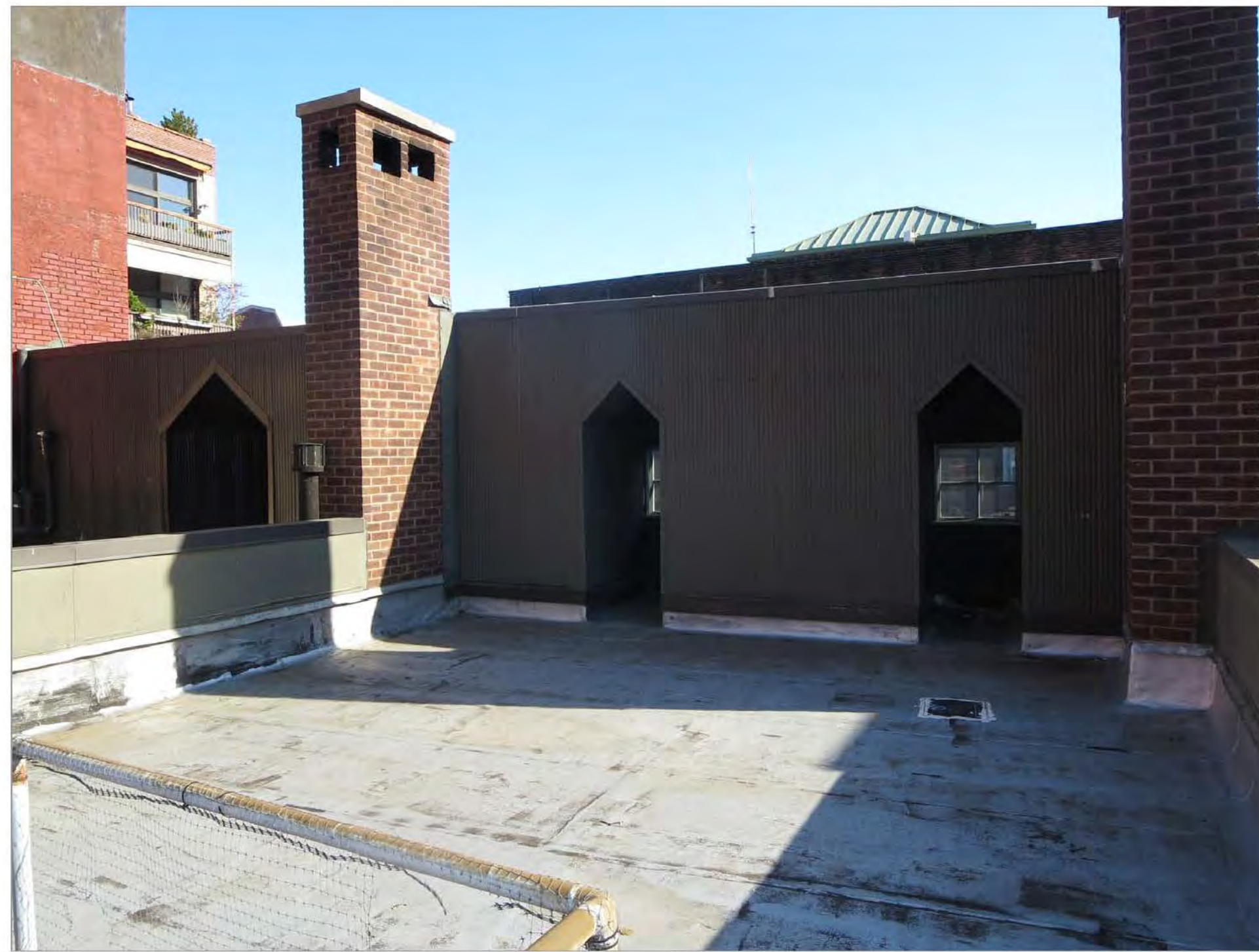
1 ROOF LOOKING SOUTH Scale: NTS
