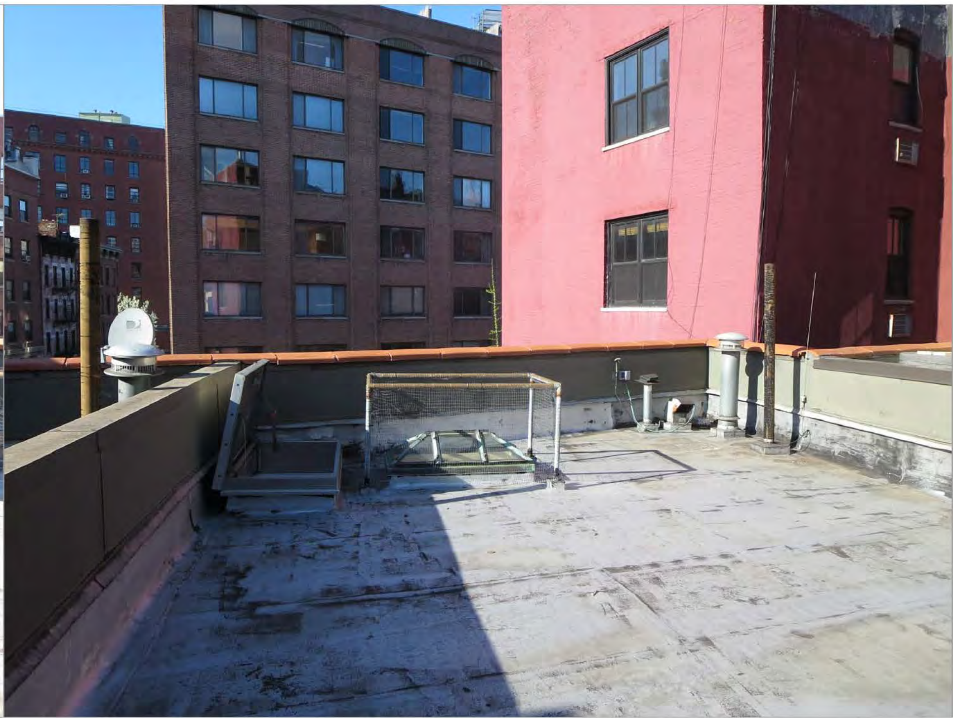
3 ROOF LOOKING NORTH Scale: NTS
