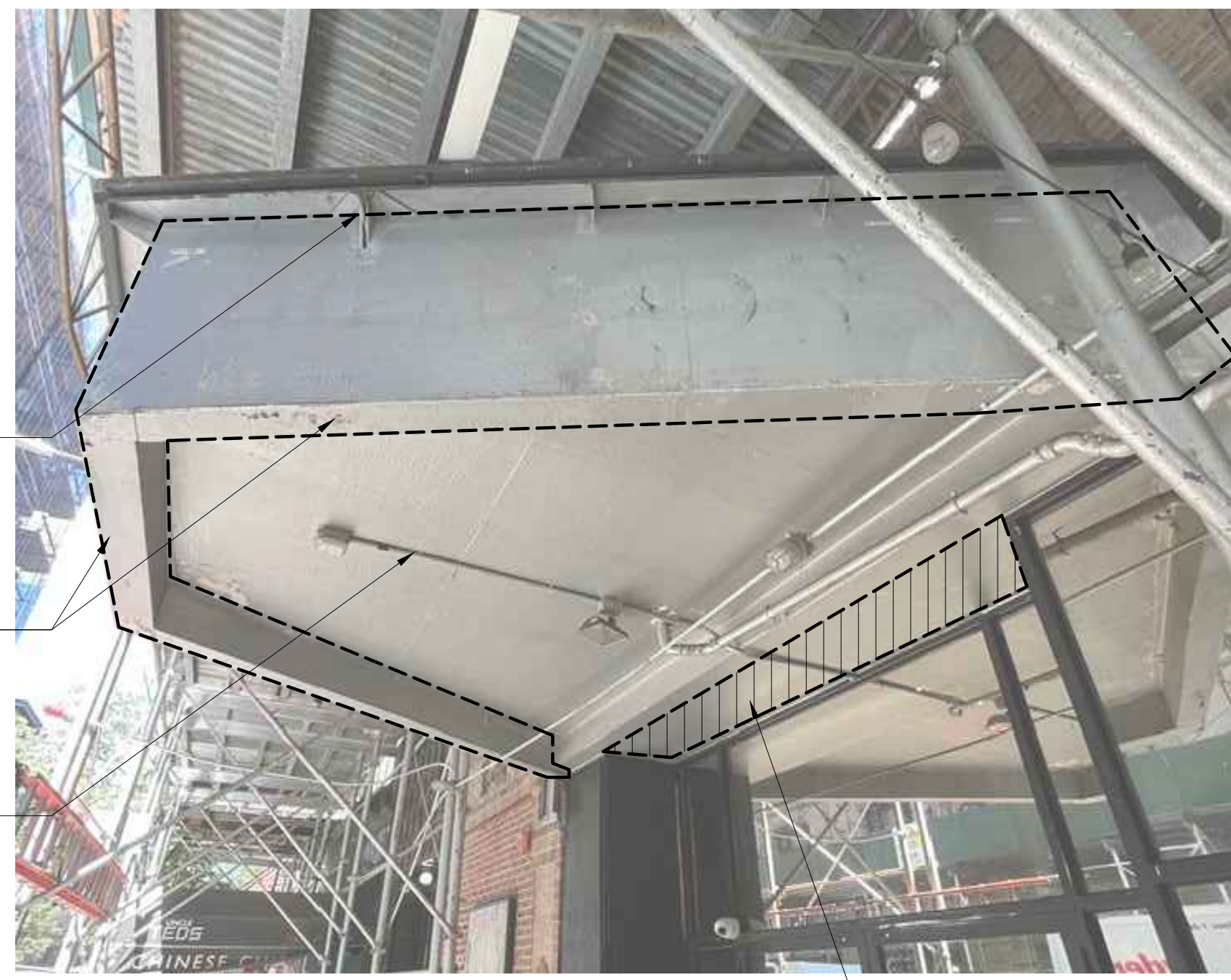
01 EXISTING MARQUEE CONDITION SCALE: N/A
