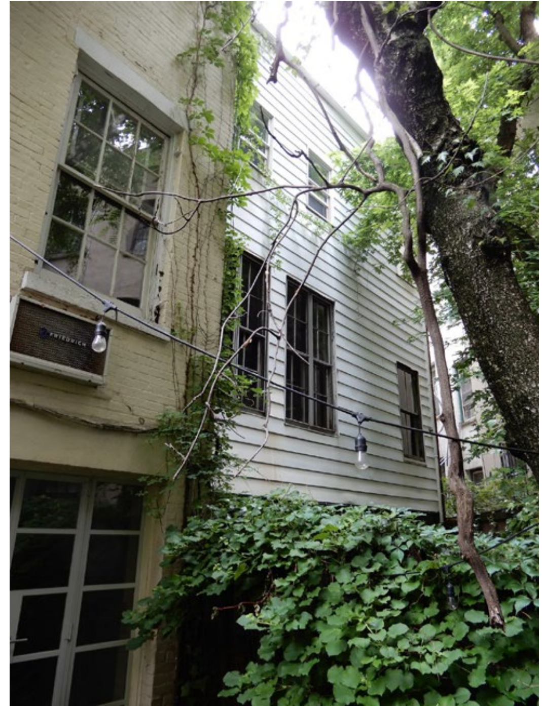
Context: Rear Yard Looking East
