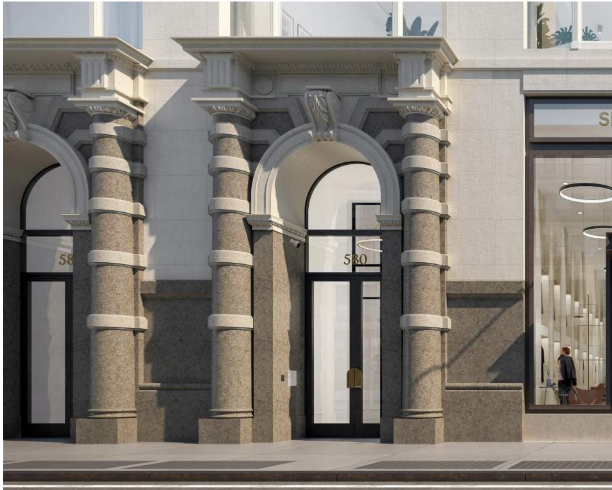
Broadway Entry Door Replacement
