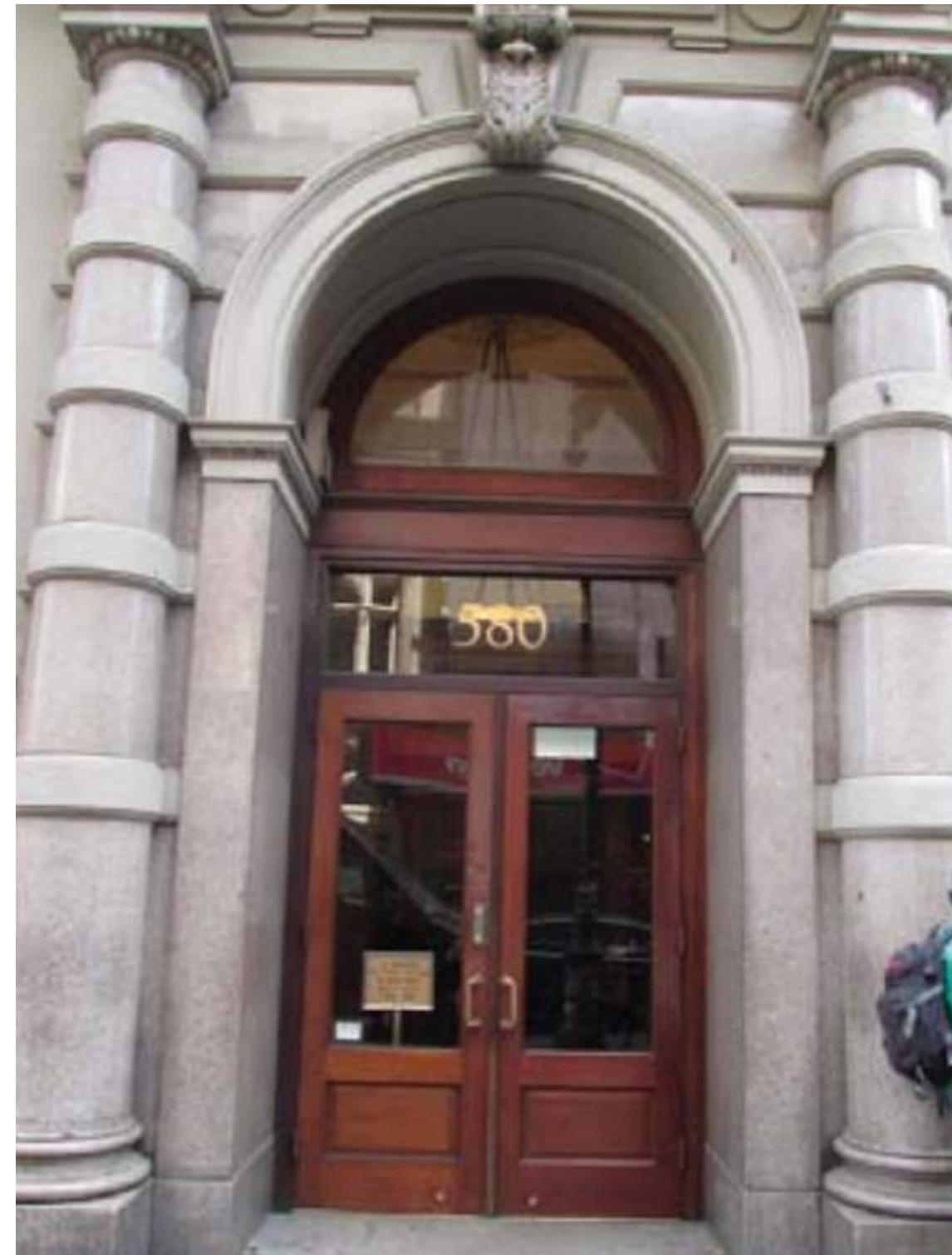
Existing Condition at 580 Broadway
