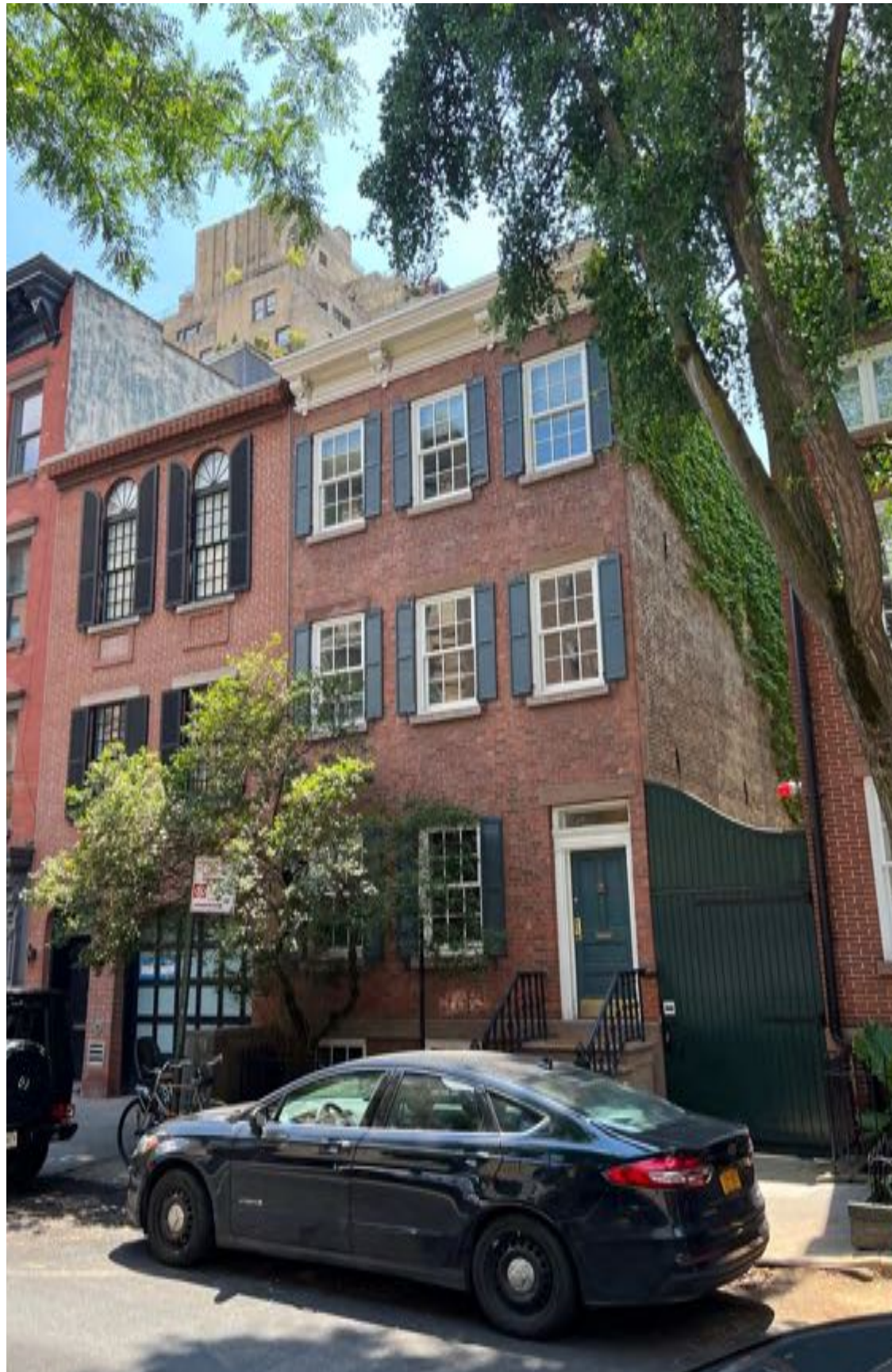
North Facade - Existing
