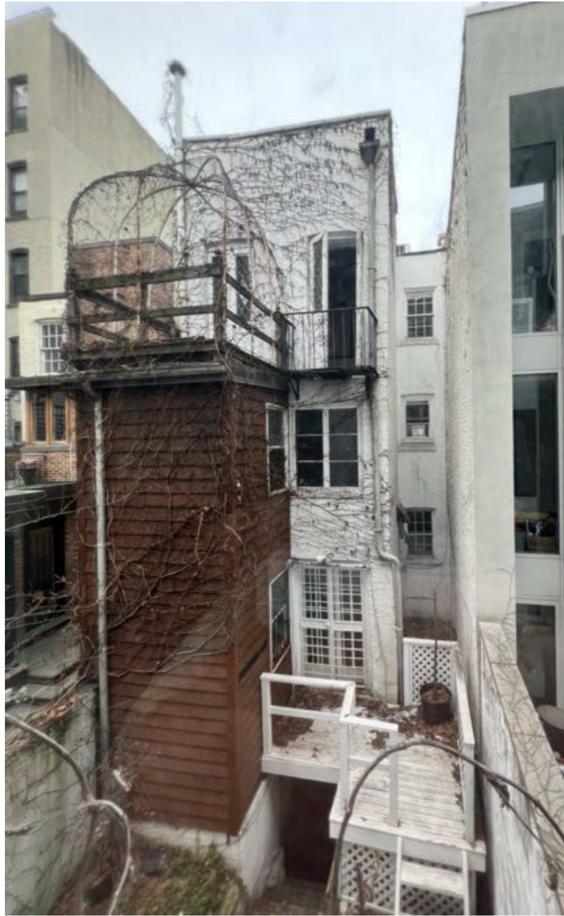
South Facade - Existing
