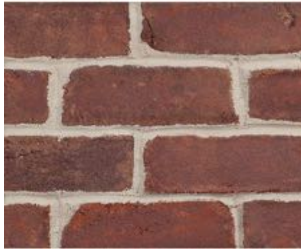
Rear Facade Brick
