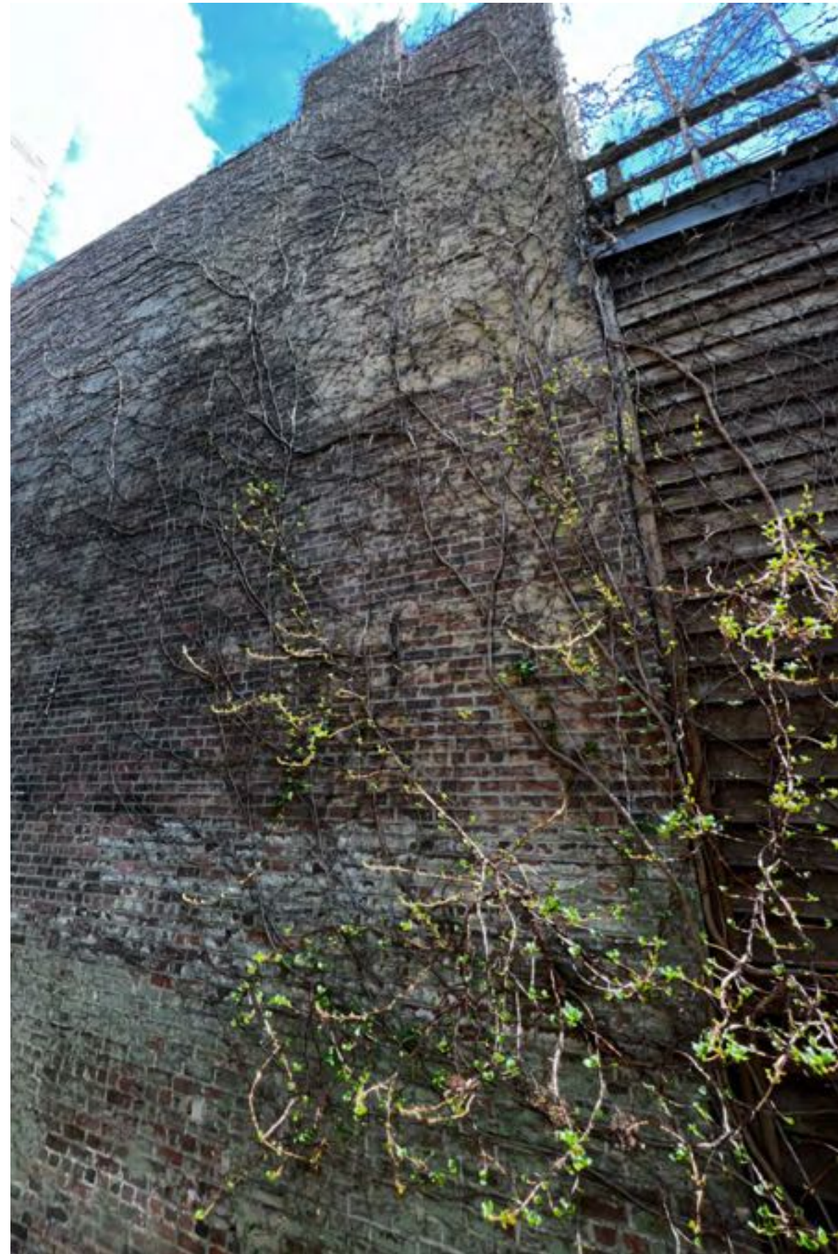
Side (West) Facade
