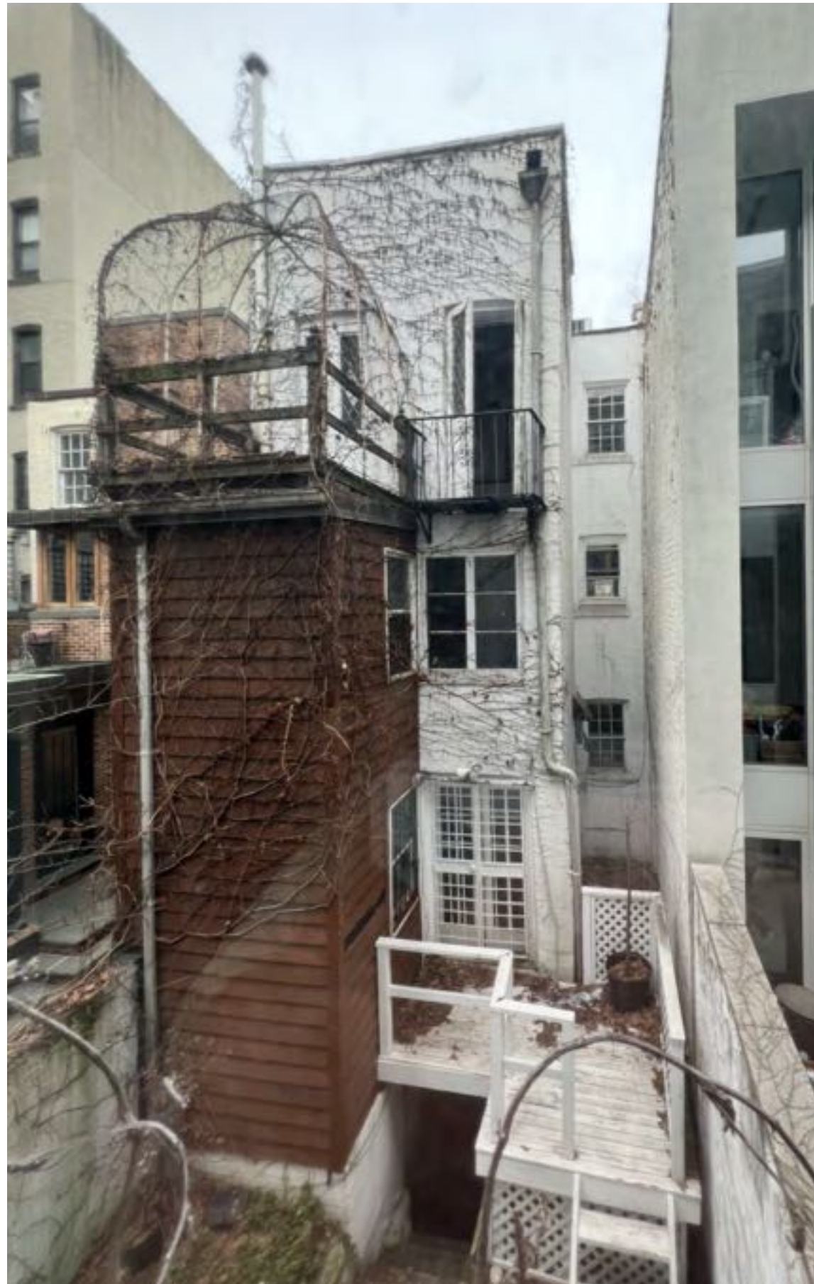
Rear (South) Facade
