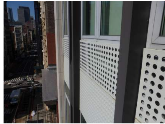
Existing Facade - Broadway
