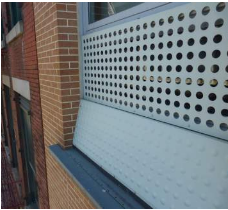
Existing Facade - Mercer Street
