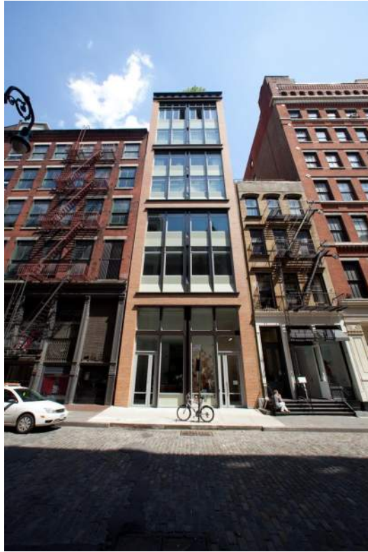
72 Mercer Facade, 2008, after construction completion (TRA Studio)
