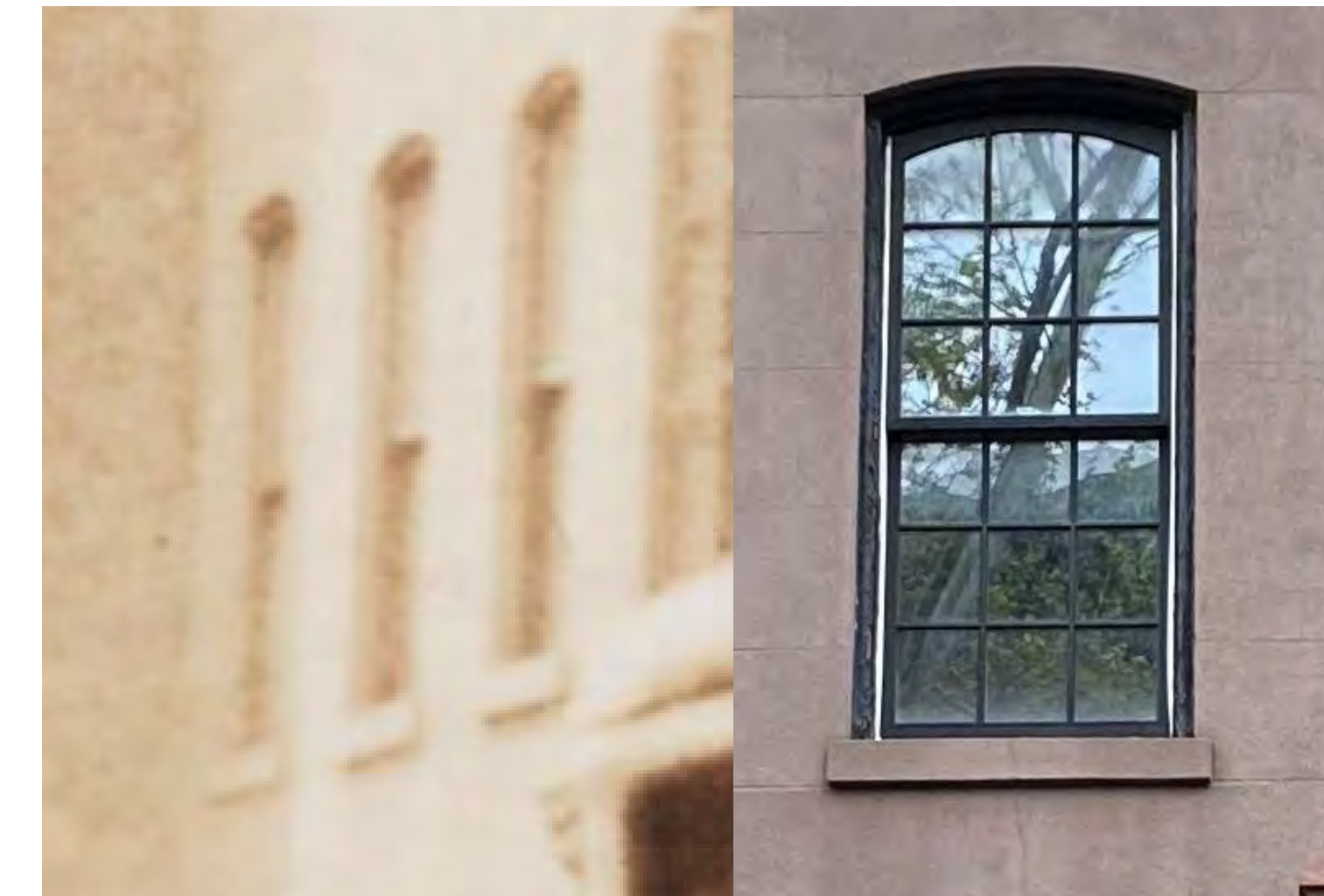
3 Upper Floor Windows (Before & After Renovation) SCALE: 1:0.17
