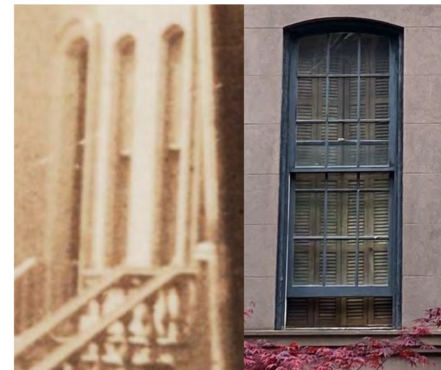
2 1st Floor Windows (Before & After Renovation) SCALE: 1:0.17
