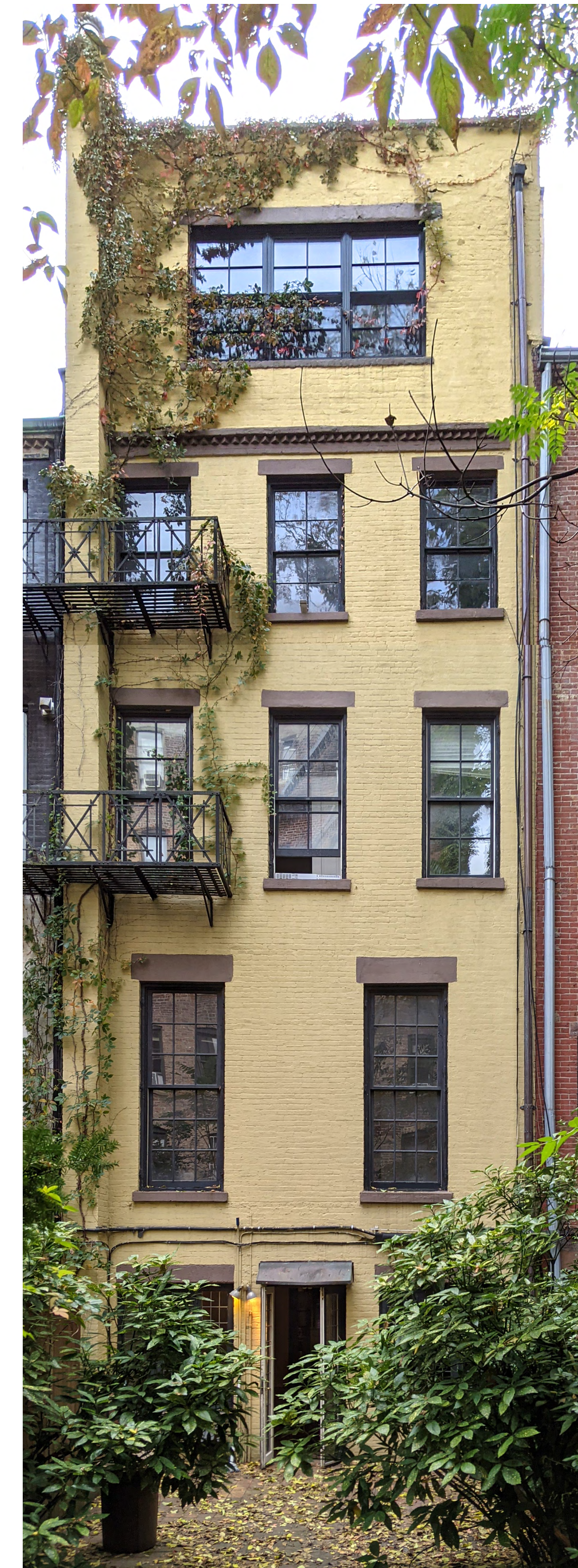
1 Existing Rear Yard Photo SCALE: 1:5
