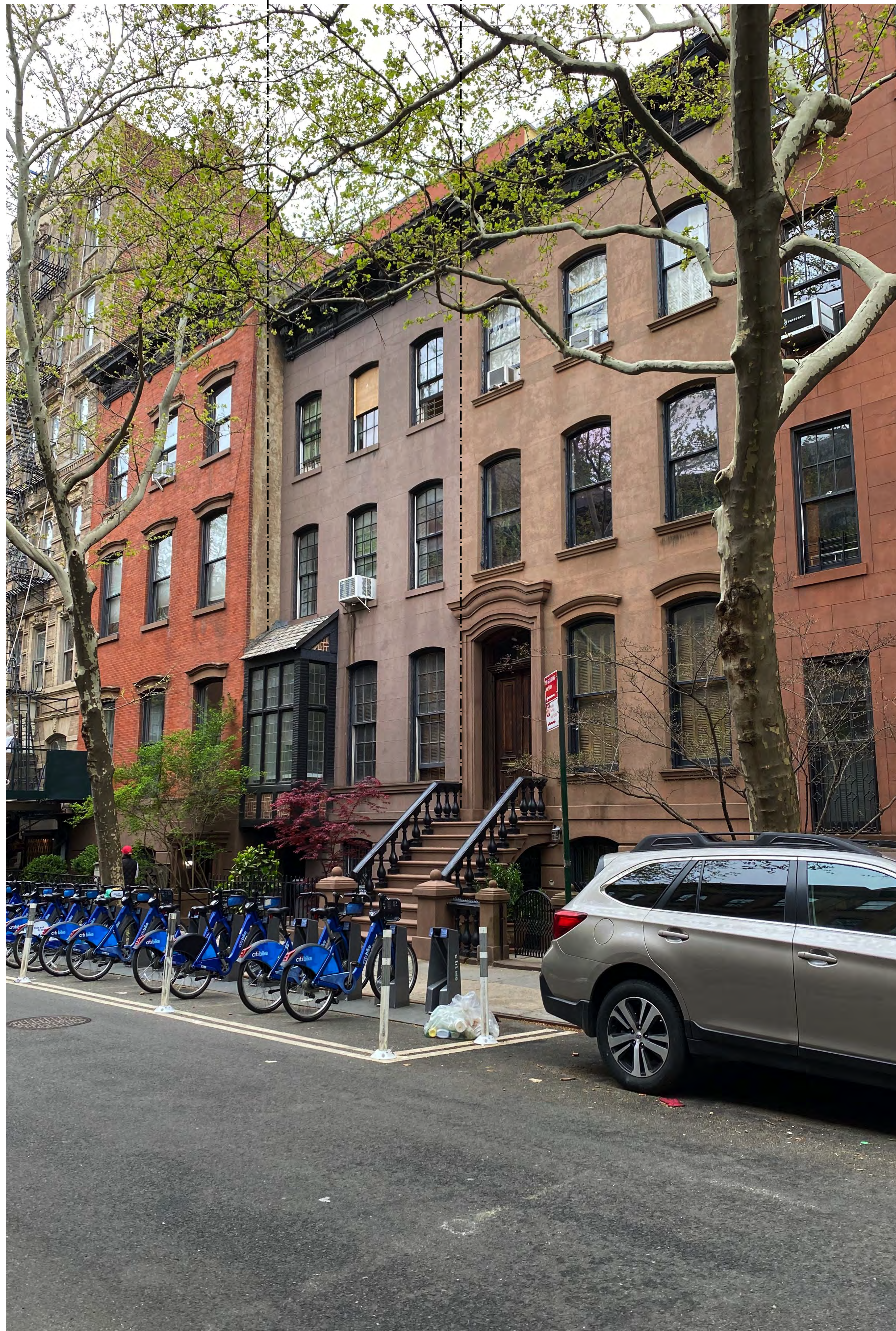
1 73 Perry St: Existing Photo SCALE: 1:2.70
