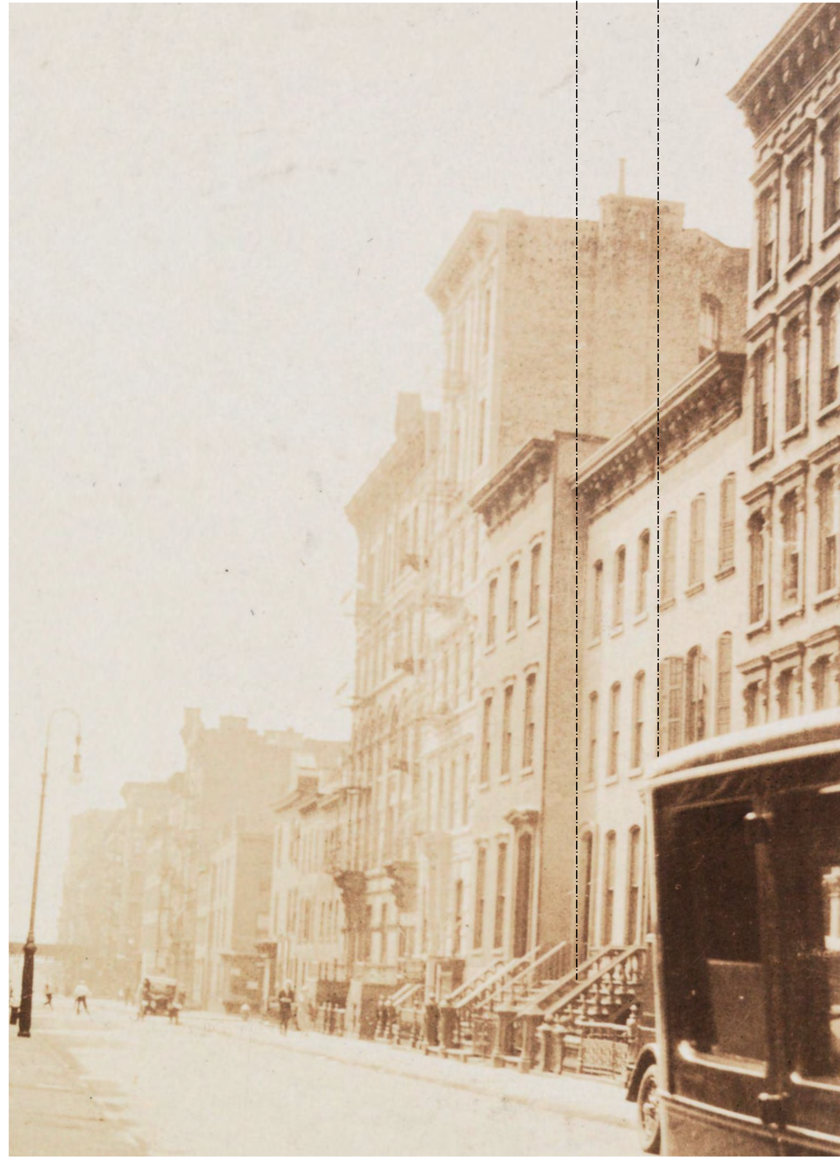
2 Perry St: (1925, Before Renovation) SCALE: 1:0.33
