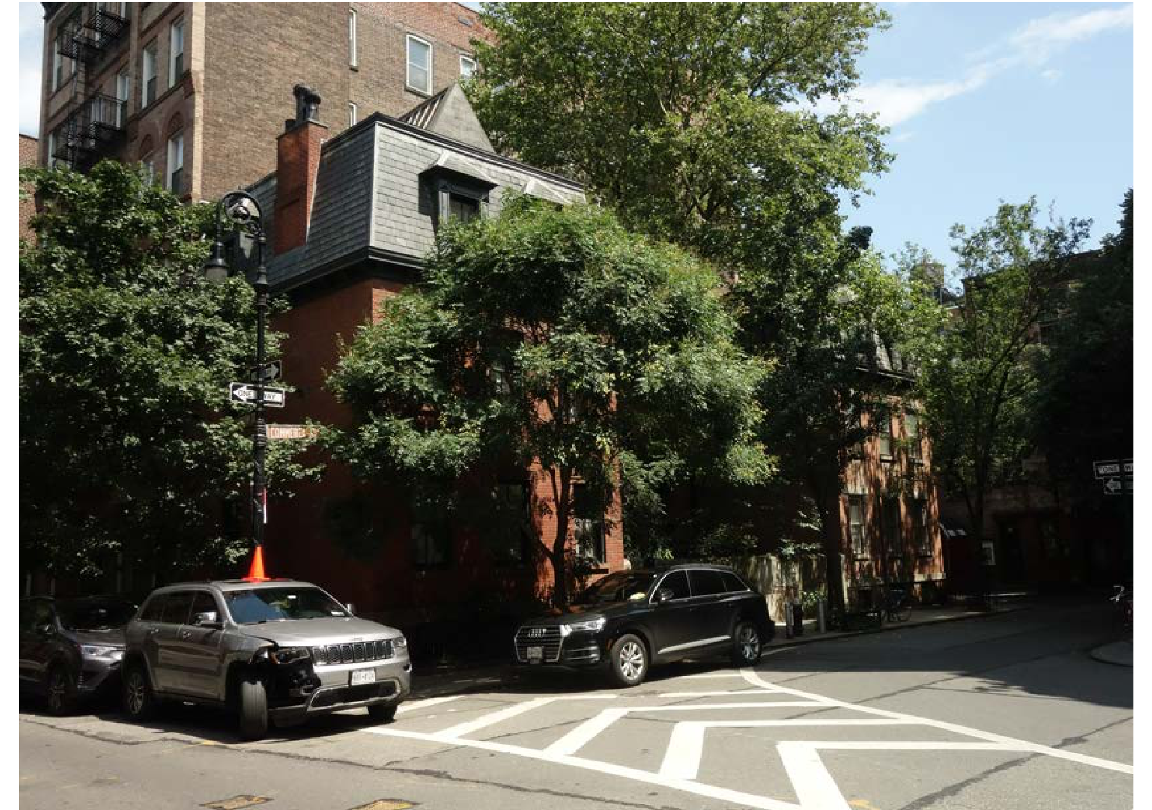
PHOTO OF 41 & 39 COMMERCE STREET EX'G SOUTHWEST FACADE, 2021 N.T.S.
