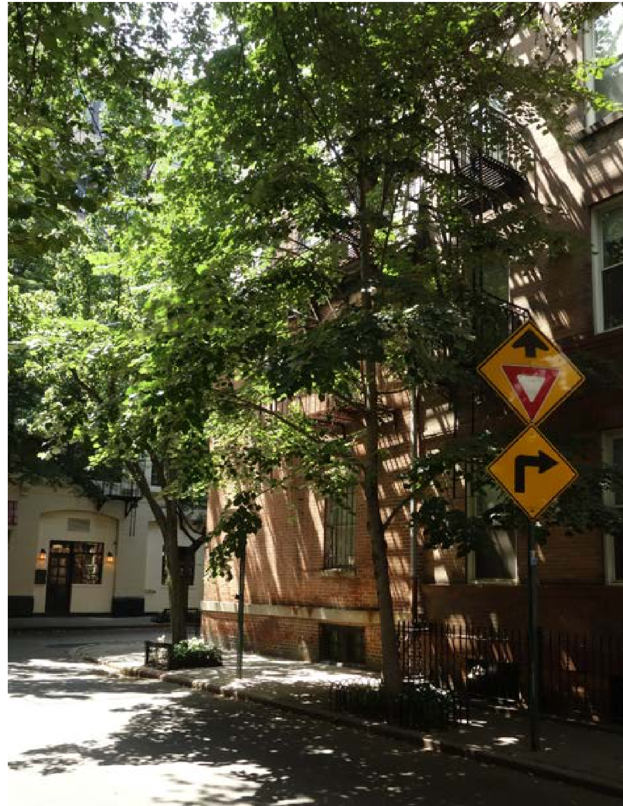
PHOTO OF 39 COMMERCE STREET EX'G SOUTHEAST FACADE, 2021, N.T.S.
