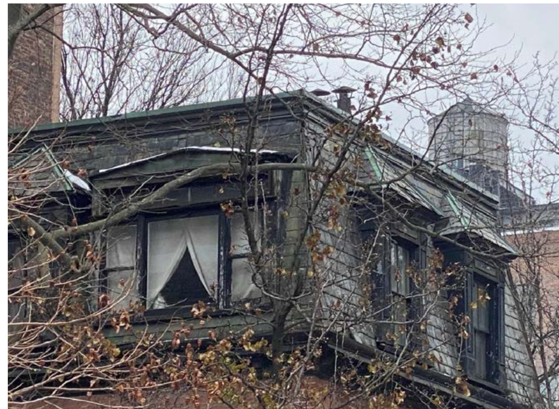
39 COMMERCE ST ROOF CLOSE-UP PHOTO, 2021 N.T.S.
