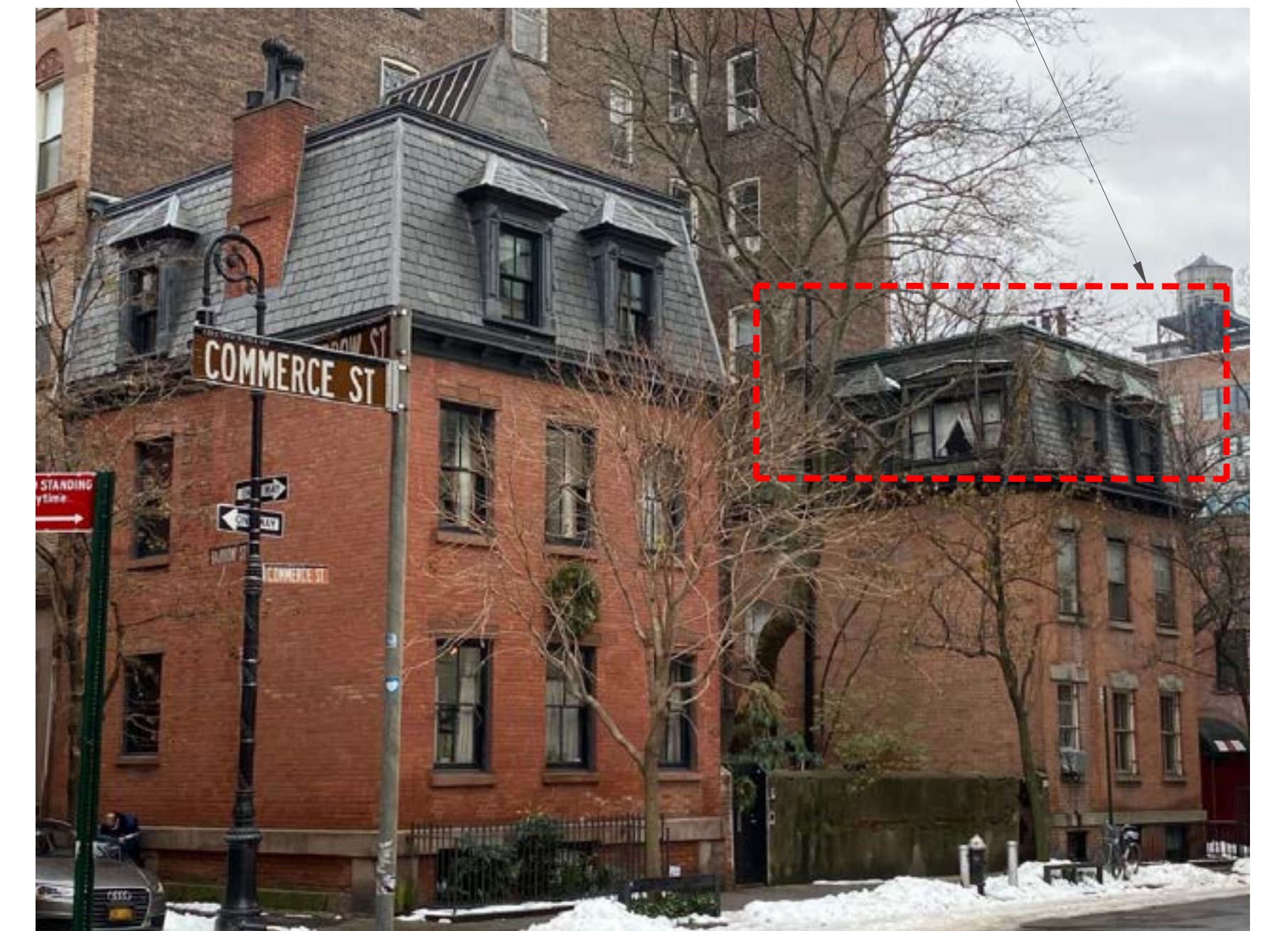
PHOTO OF COMMERCE STREET SOUTHWEST FACADE, 2021 N.T.S.
