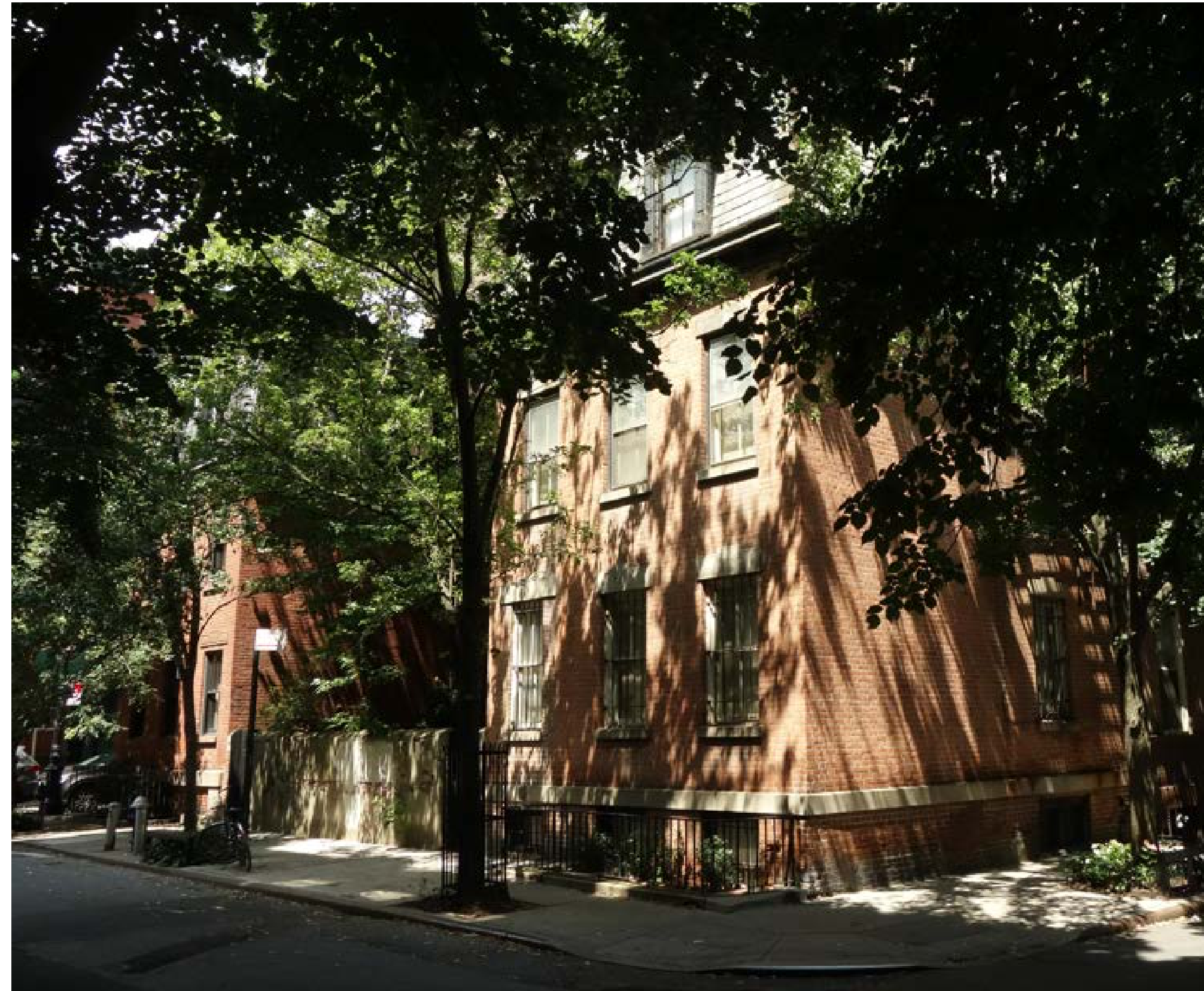
PHOTO OF 39 COMMERCE STREET EX'G SOUTHWEST FACADE, 2021 N.T.S.
