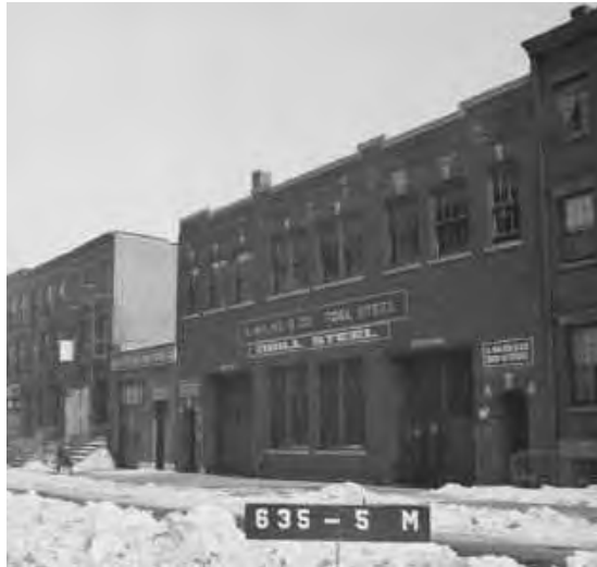
1940 Photo - Steel warehouse and office
