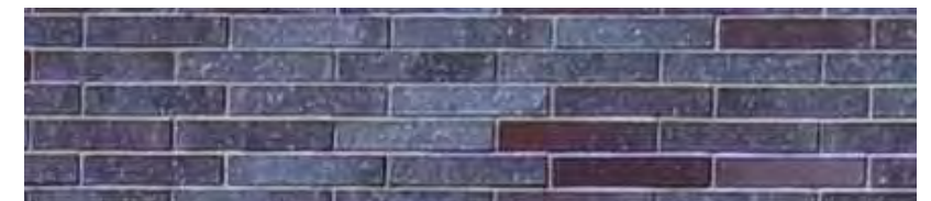
Rear east facade brick veneer over stucco, 2008
