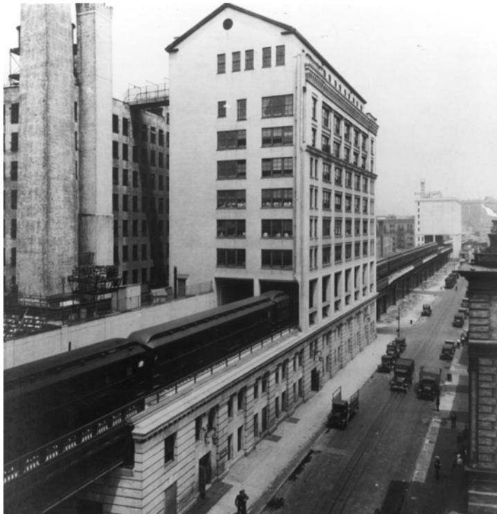
VIEW 2 Bell Laboratories Building, 1936 (Westbeth)
