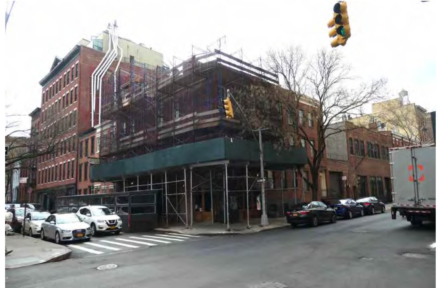
Block context, looking south-east
