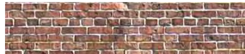
Washington Street facade brick, 1913
