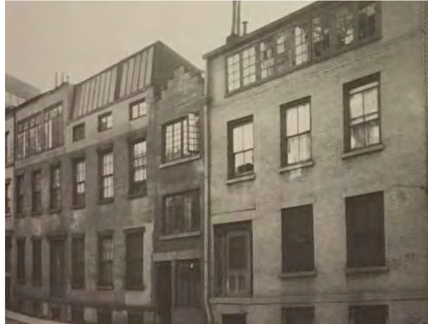
Early 20th-century studio additions, 73-77 Bedford Street, date unknown. (The Row House Reborn)
