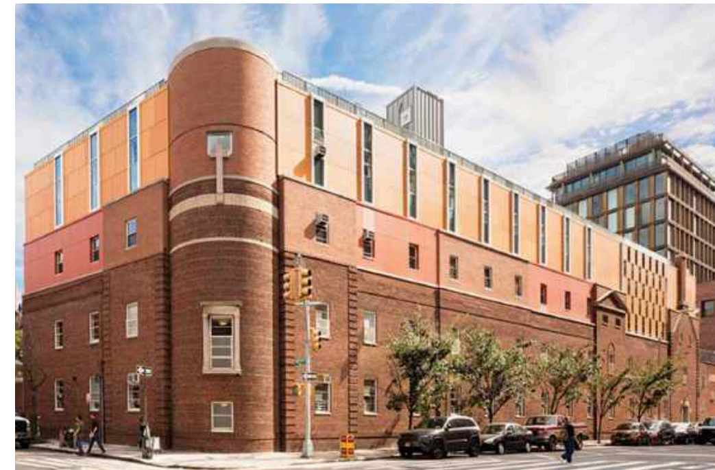
St. Luke's School, 2014 LPC Approval. (ABA Studio) (Google Maps, Architectural Record)
