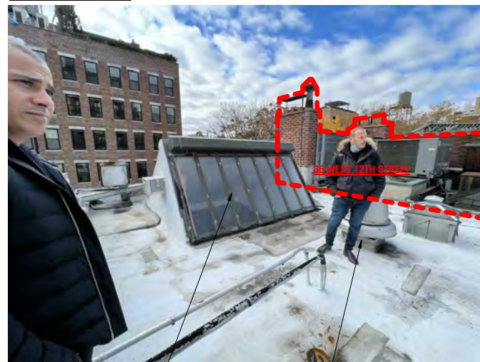
ROOF VIEW LOOKING SOUTH
