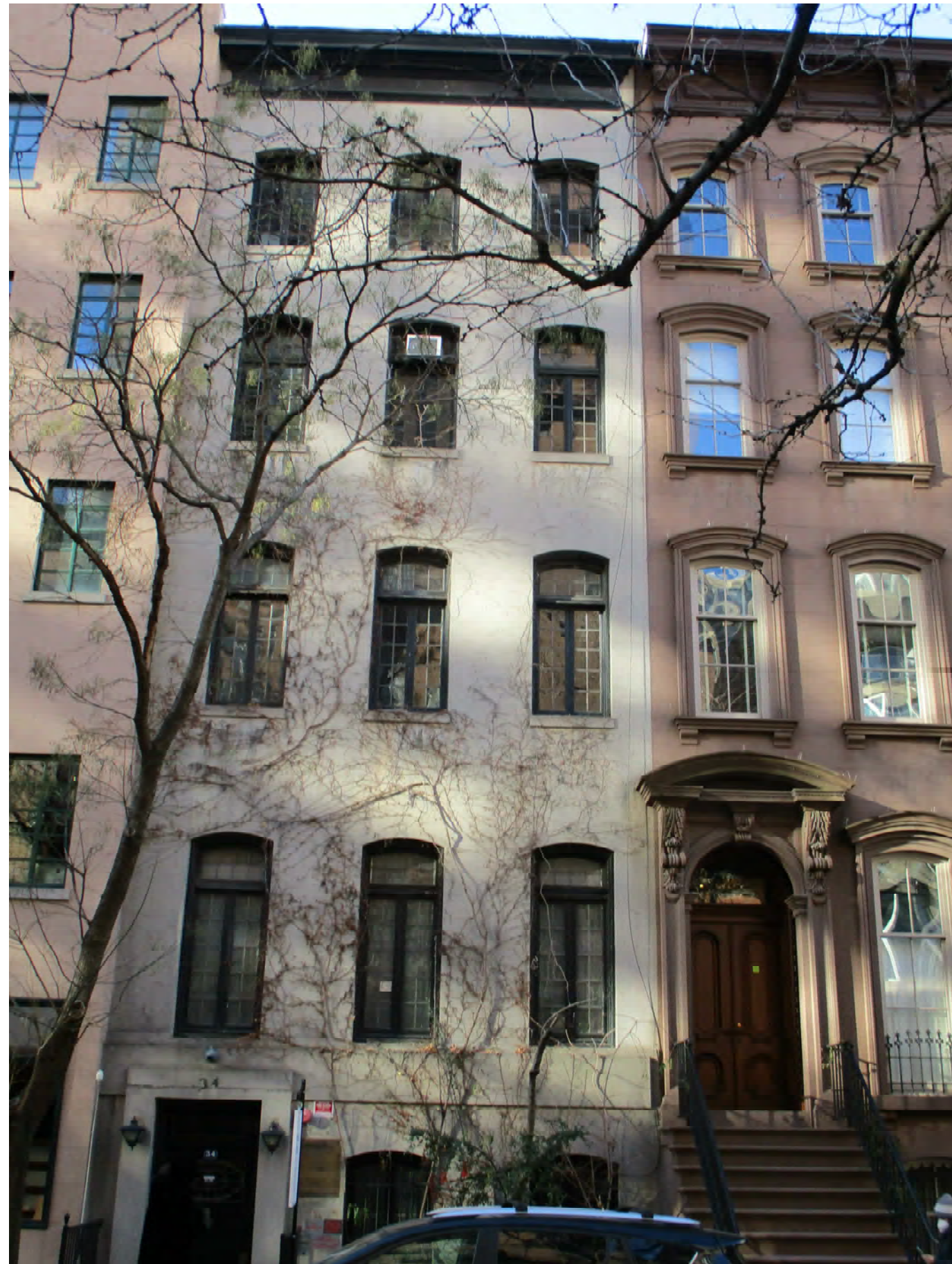
1 EXISTING FRONT FACADE (2022)
