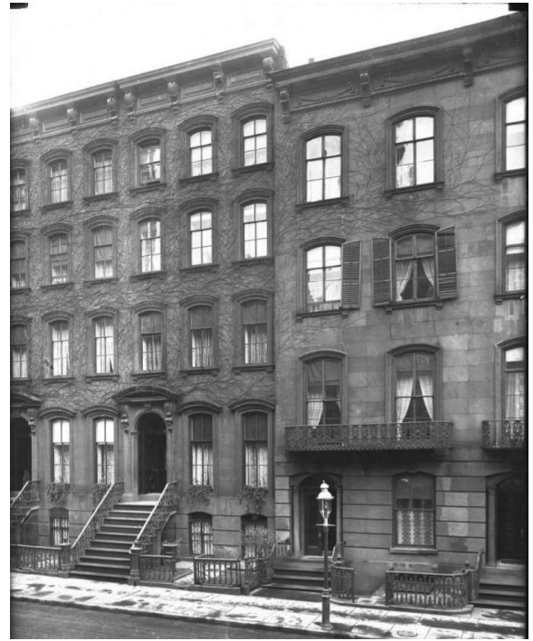
44- 48 W 12TH STREET ( BEFORE RENOVATION)
