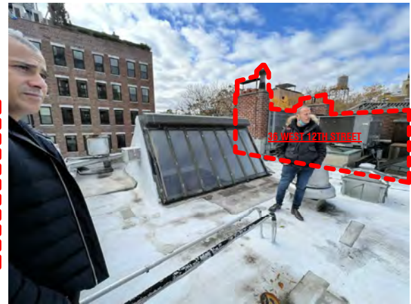
ROOF VIEW LOOKING SOUTH
