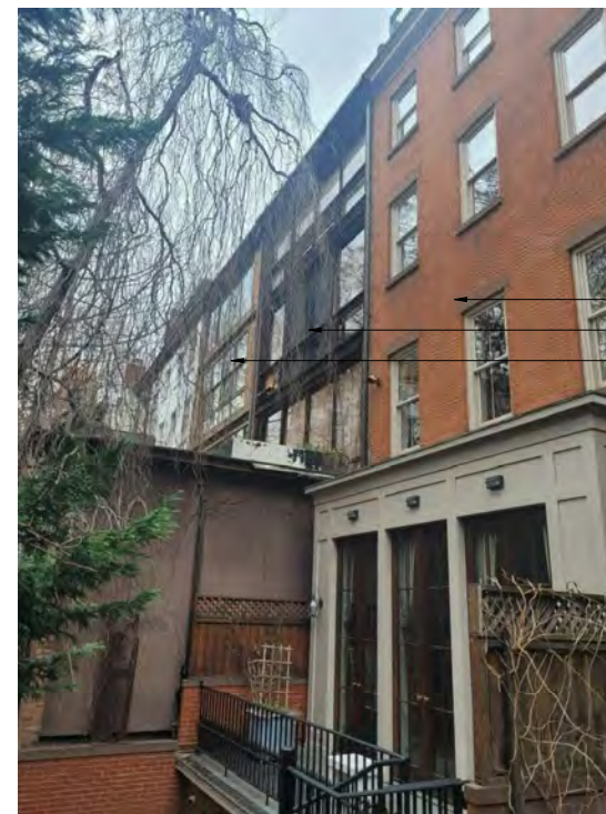
4 ANALYSIS OF NEIGHBORING REAR FACADES
