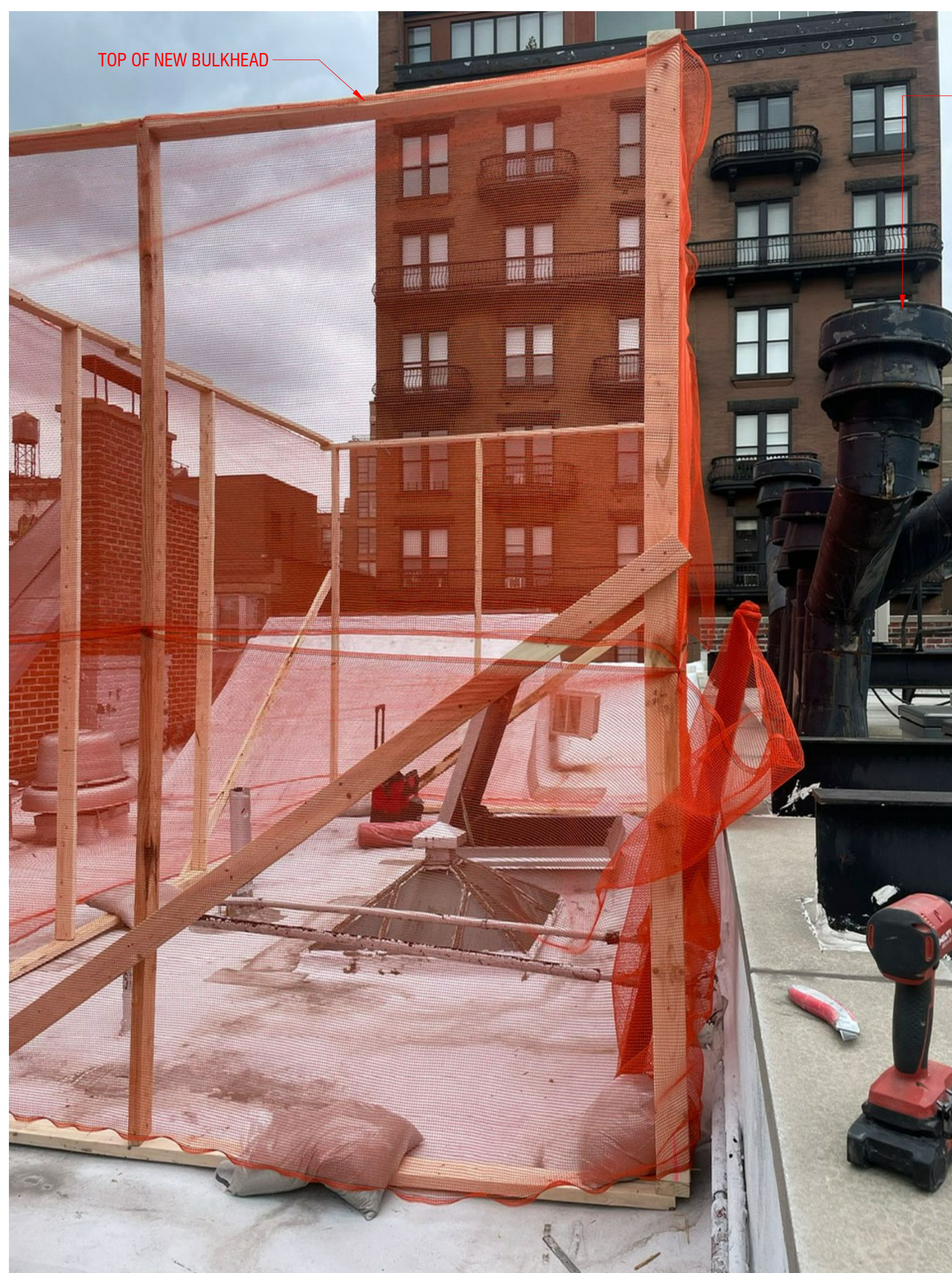
P3 MOCKUP AT ROOF LOOKING NORTH
