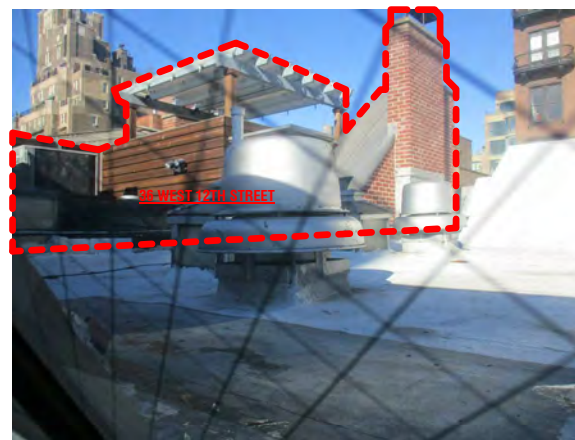
ROOF VIEW LOOKING AT 36 W 12TH STREET FROM INSIDE LOFT
