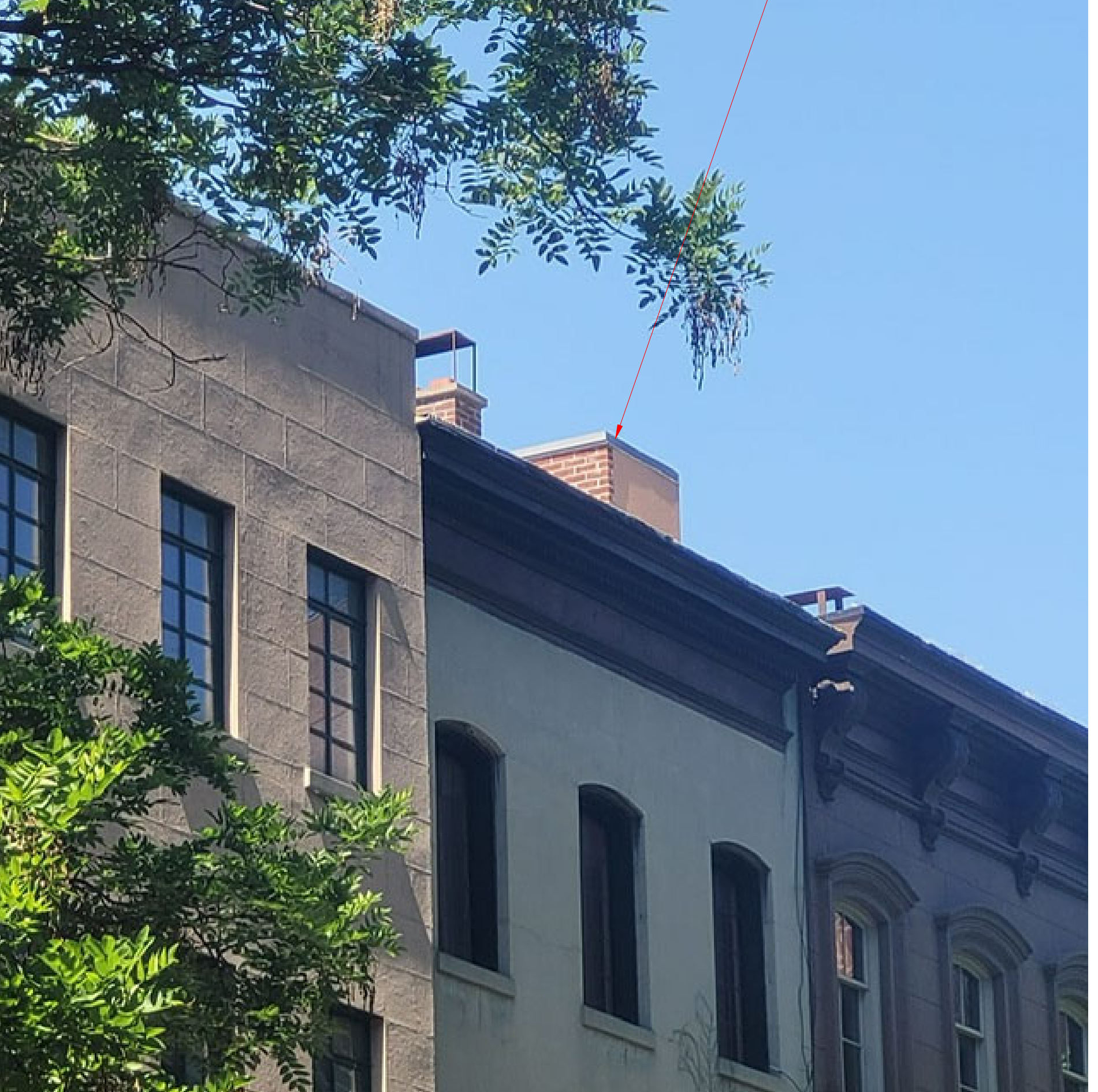
P3 MOCKUP AT STREET LOOKING WEST
