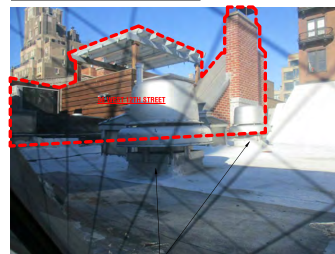
ROOF VIEW LOOKING AT 36 W 12TH STREET FROM INSIDE LOFT
