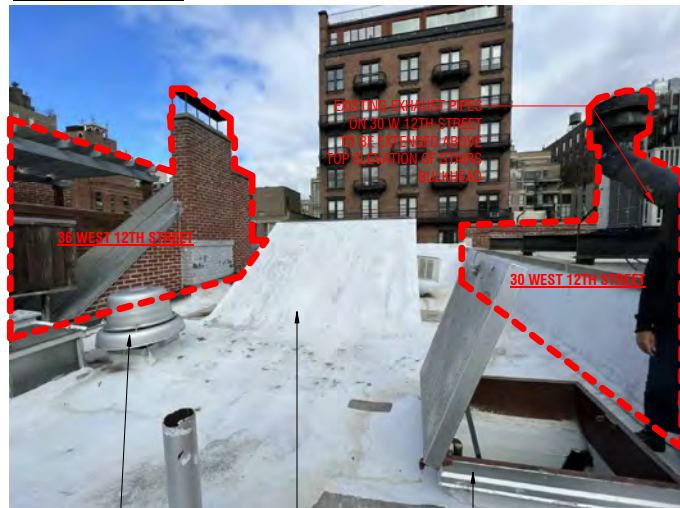
ROOF VIEW LOOKING NORTH
