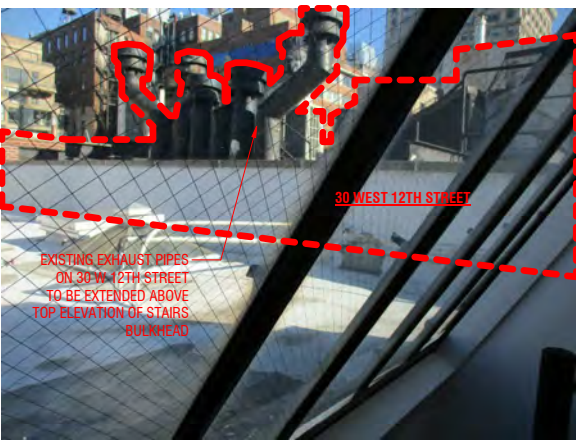
ROOF VIEW LOOKING AT 30 W 12TH STREET FROM INSIDE LOFT
