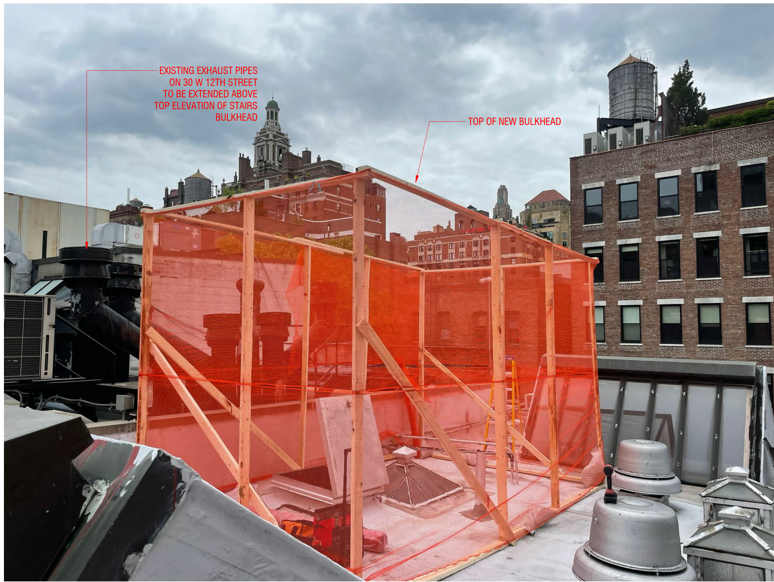
P1 MOCKUP AT ROOF LOOKING SOUTH
