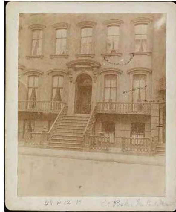
44 W 12TH STREET ( BEFORE RENOVATION)
