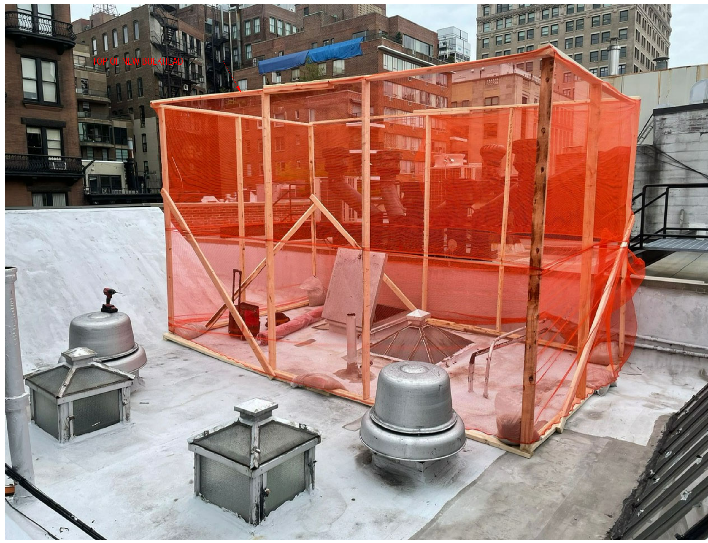
4 MOCKUP AT ROOF LOOKING EAST
