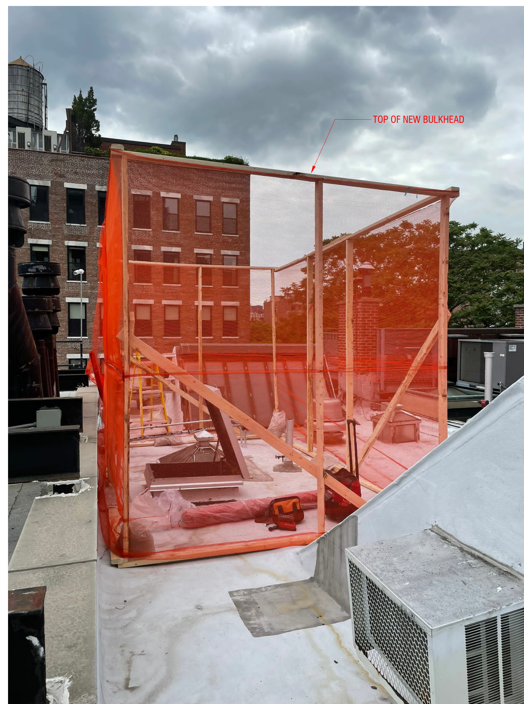
P2 MOCKUP AT ROOF LOOKING SOUTHWEST
