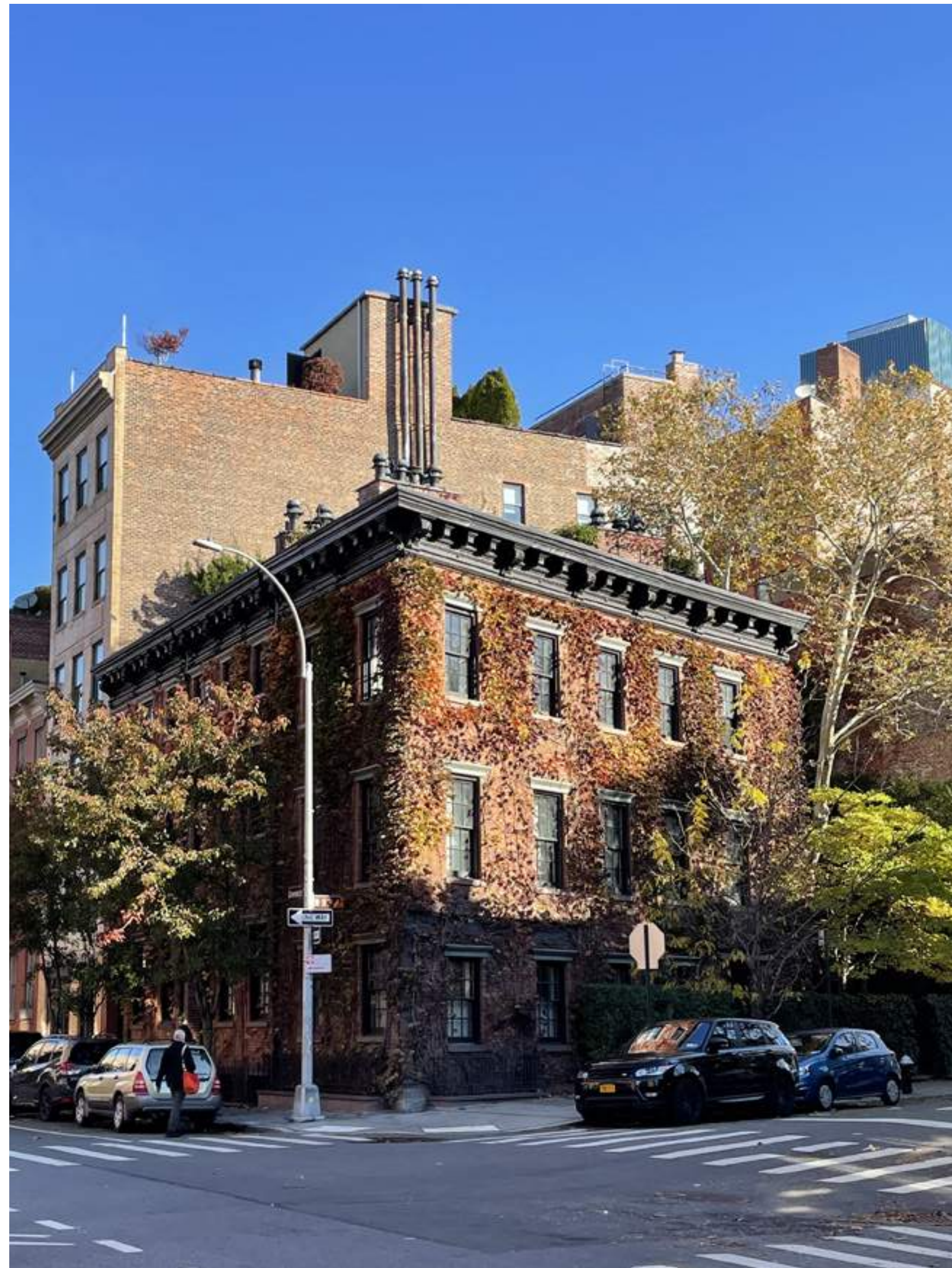
view from southwest corner Greenwich and 11th Street
