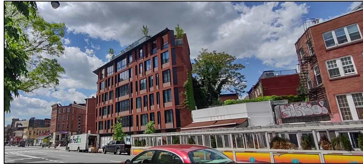
Looking southwest on Seventh Avenue South, from near Charles Street.
