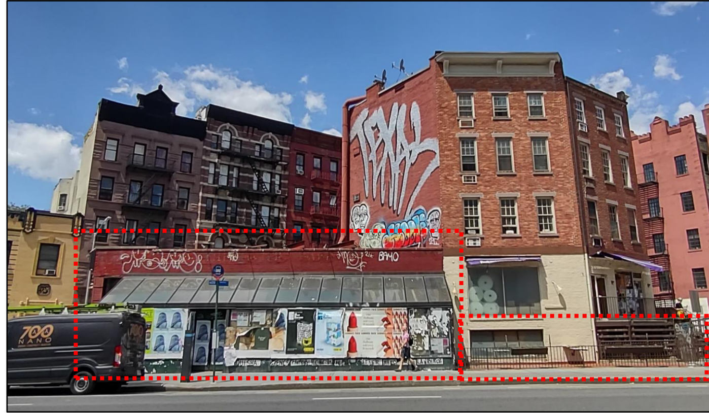
Seventh Avenue South elevation.
