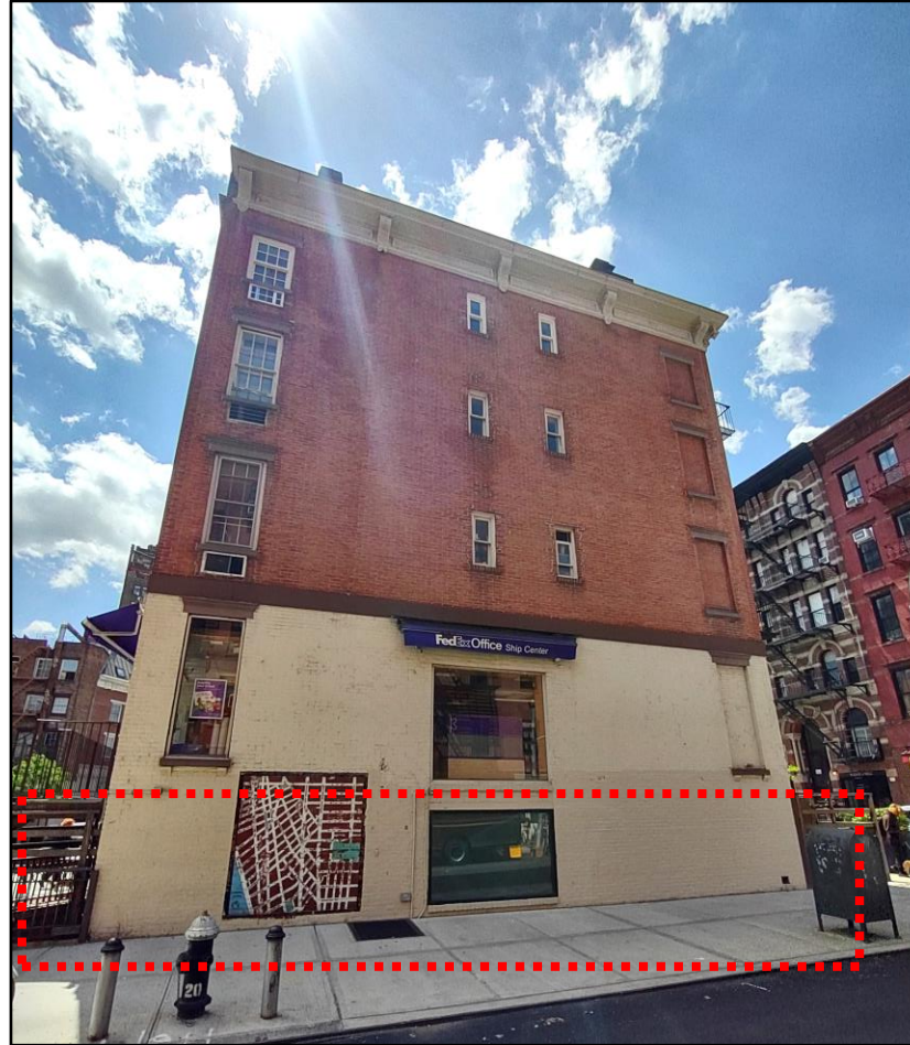
Restaurant space at West 10 th Street elevation.
