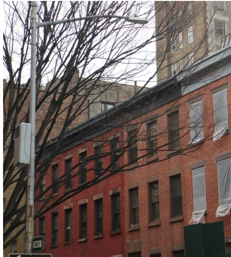
existing (close up)
