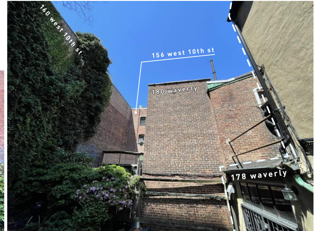
view of northern neighbors from 178 rear yard
