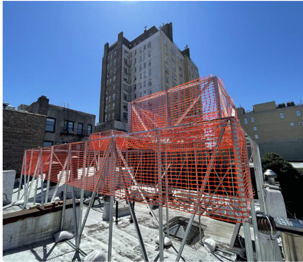
mock up in place on the roof of 176-178 waverly place
