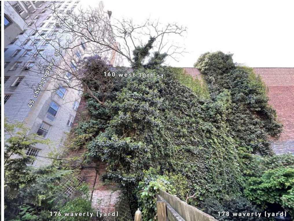
view of back side of yard
