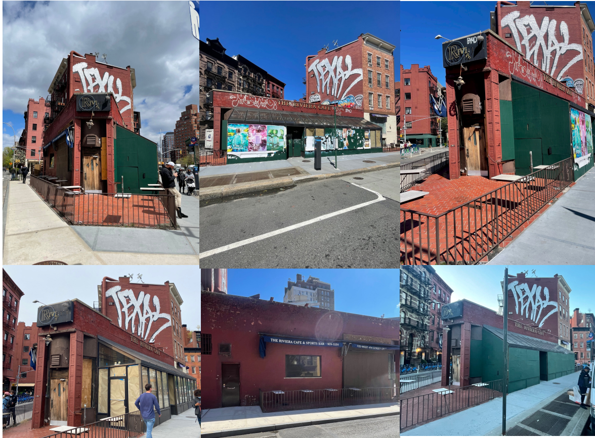
Existing Conditions – Façades
