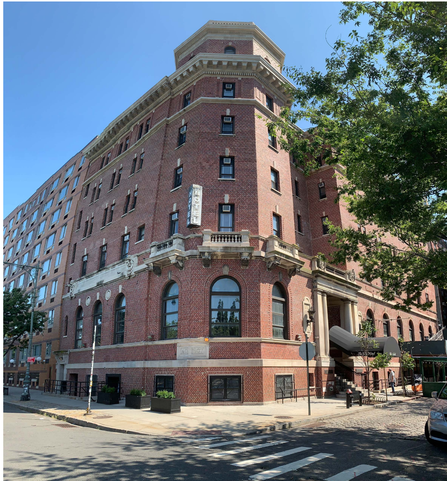
EXISTING BUILDING FACADE - SOUTH WEST CORNER FROM WEST STREET
