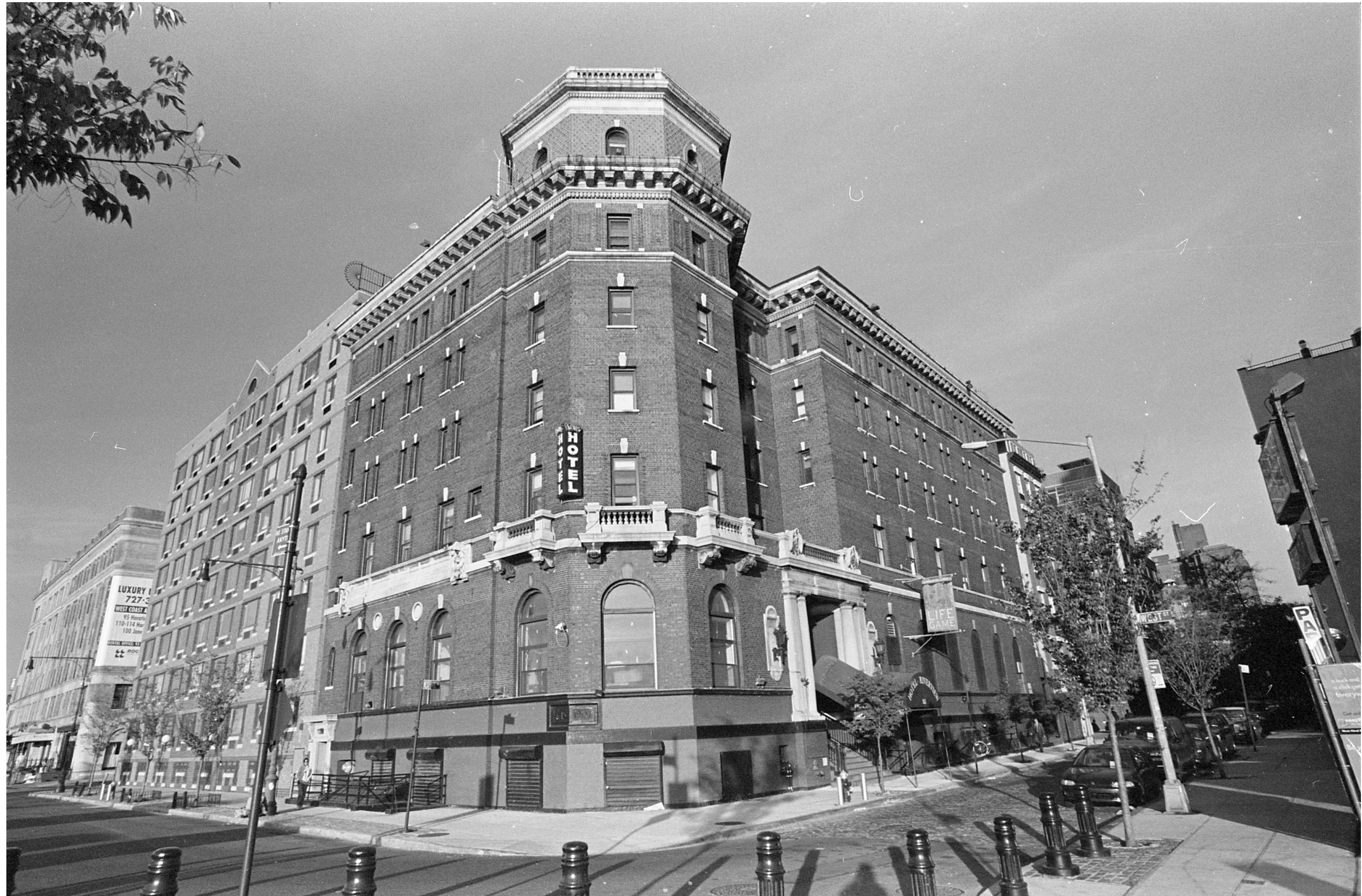
LPC DESIGNATION PHOTO, 2000
