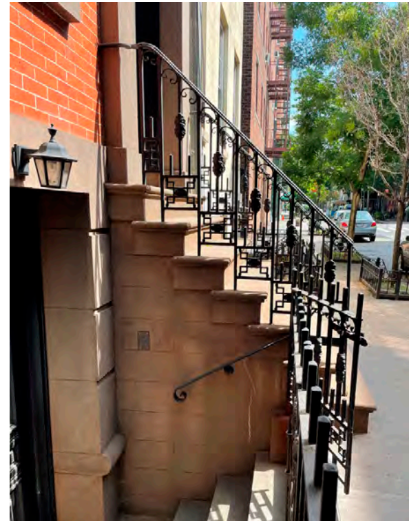
2. View of 107 Areaway
