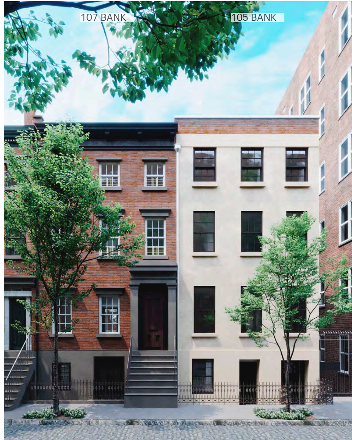
Existing 107 and 105 bank
