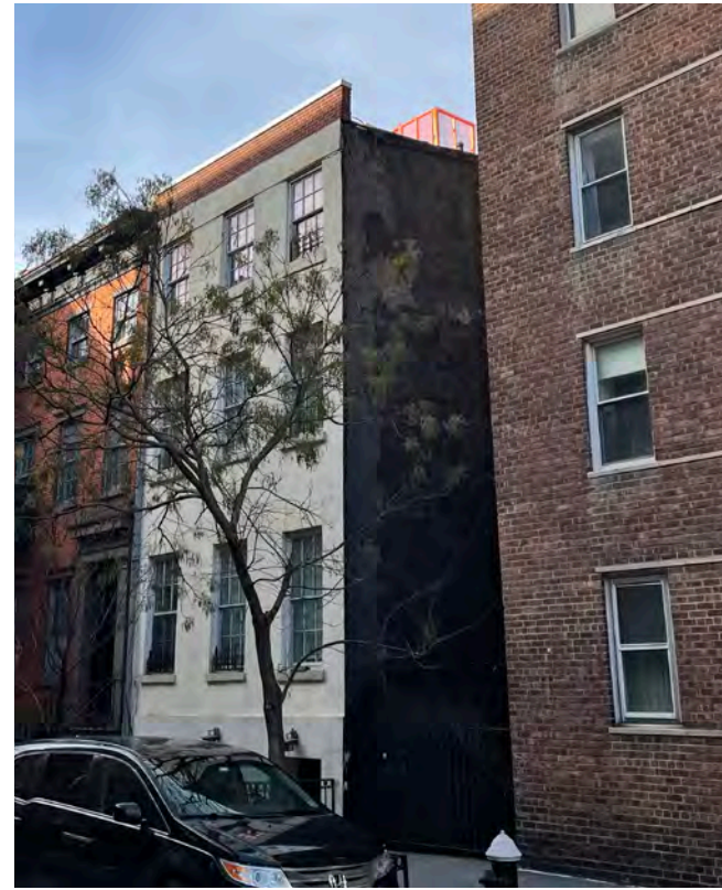
1. View of Existing 105 Alley
