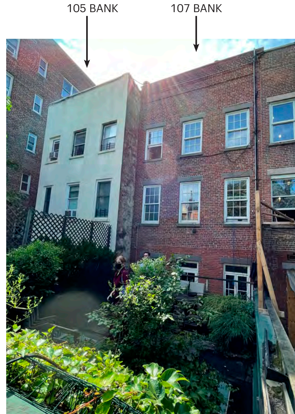
105 and 107 Bank - Current Rear Elevation
