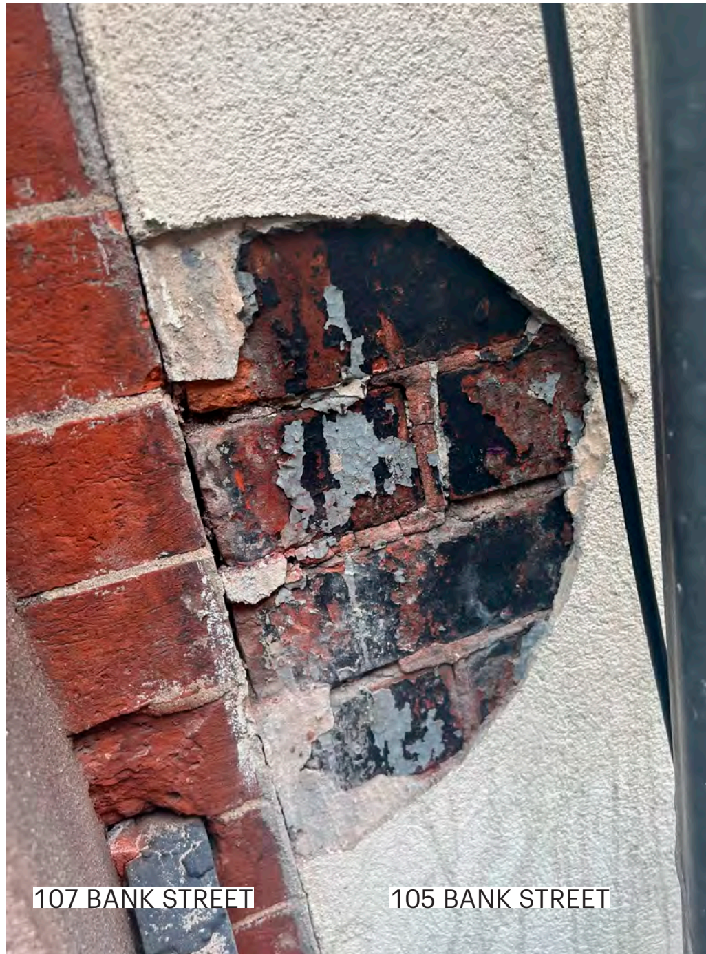
EXISTING BRICK UNDER STUCCO
