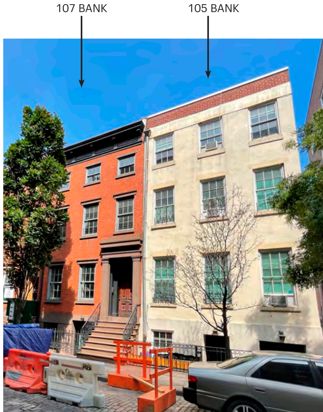
107 and 105 Bank - Current Street Elevation
