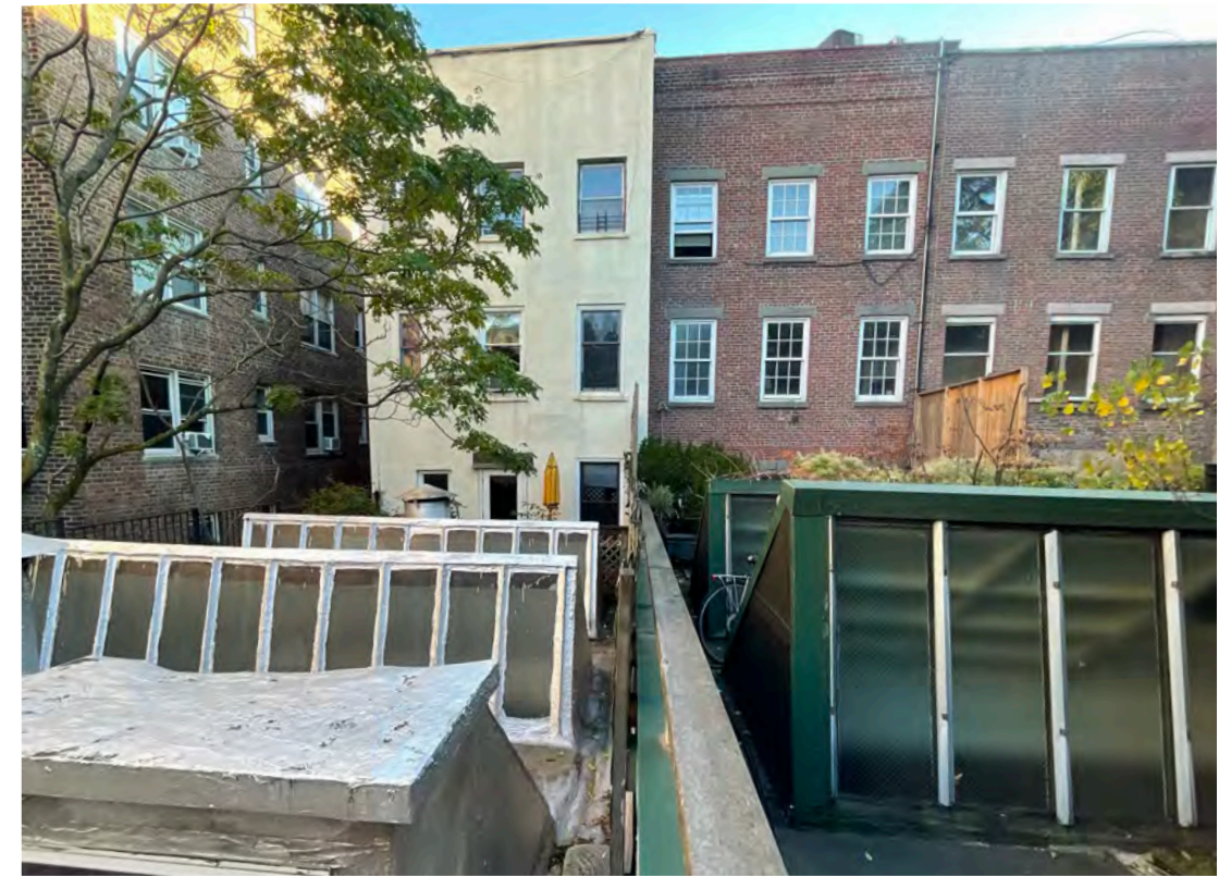
3. View of 105 and 107 Rear Facades.
