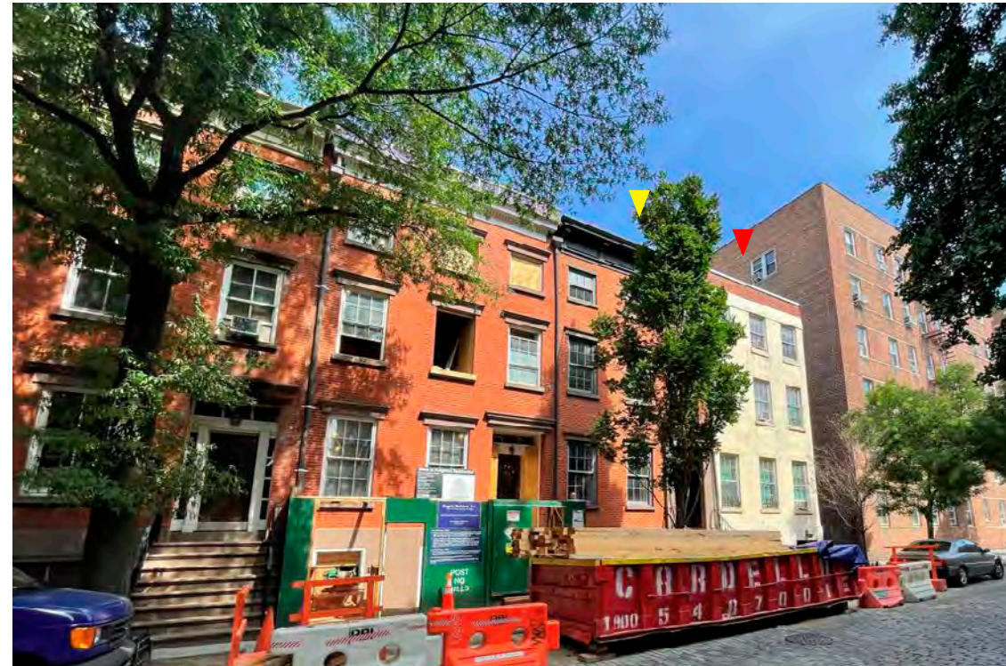
2. View down Bank St.
