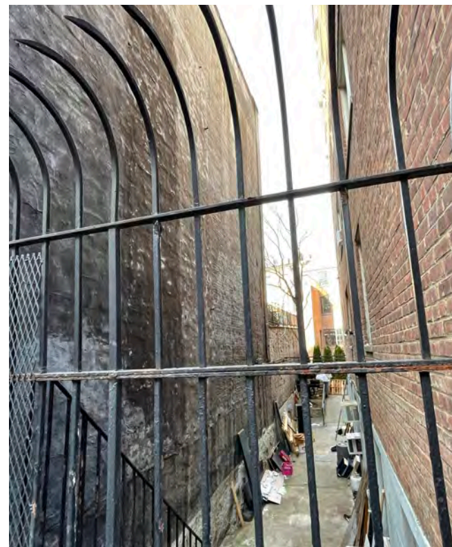
3. View of Existing 105 Alley
