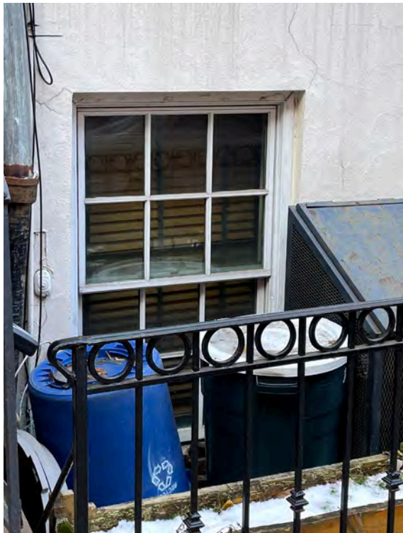
Existing 105 areaway window
