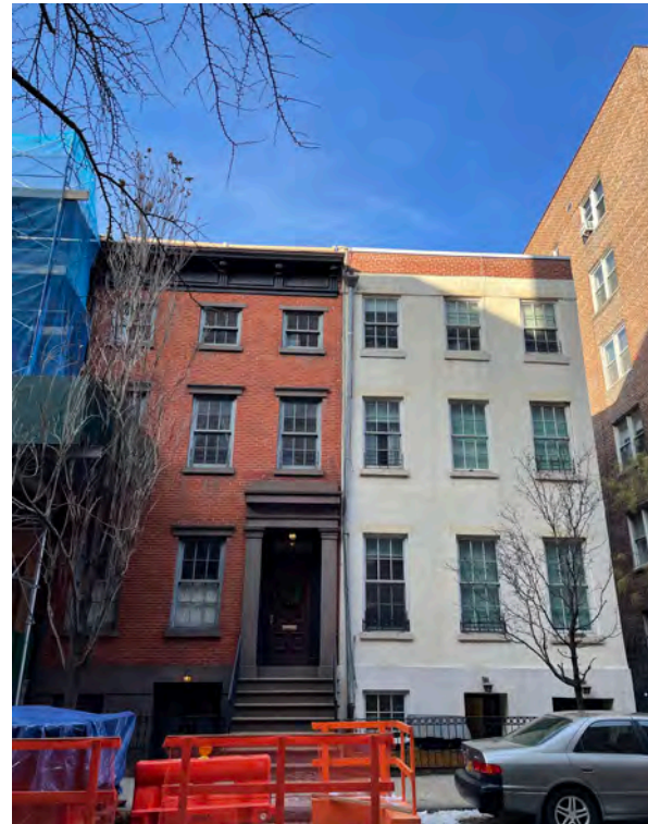
1. View of Street Facade
