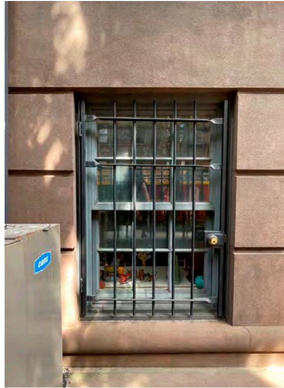
Existing 105 areaway window
