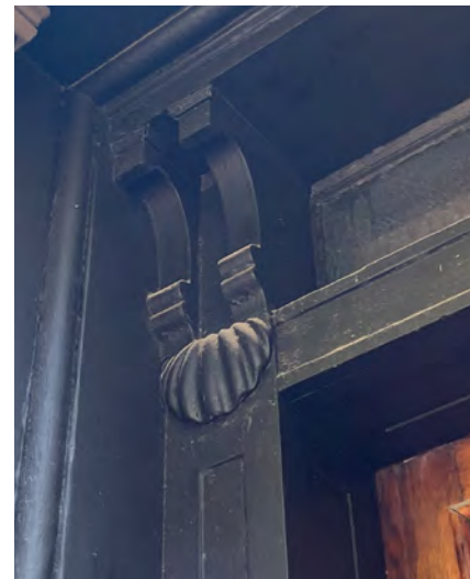
Existing door frame bracket detail
