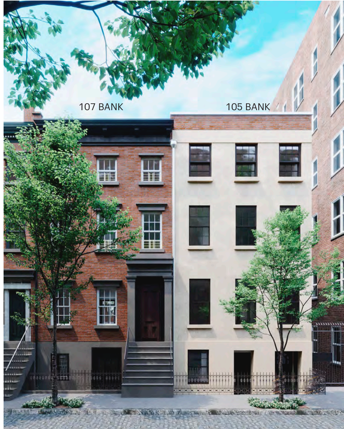
Existing 107 and 105 Bank
