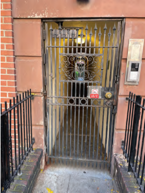
11th Street Gate to passageway to interior yard
