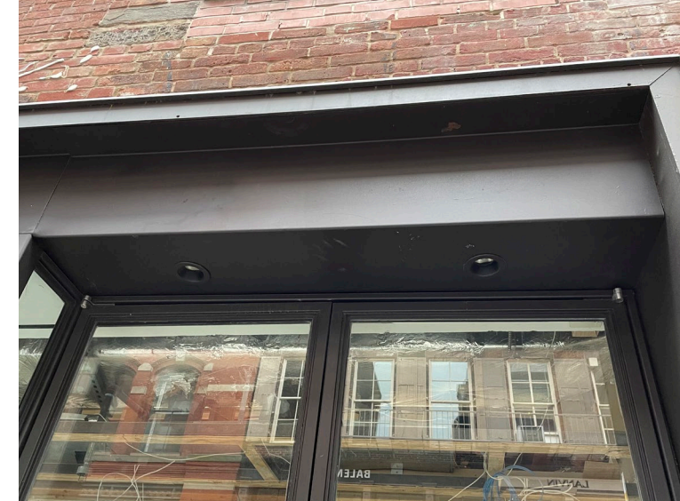
Retail entry header and lighting detail.
