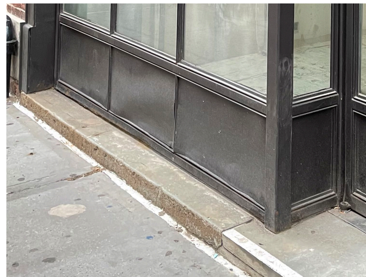
Storefront base, granite sill.
