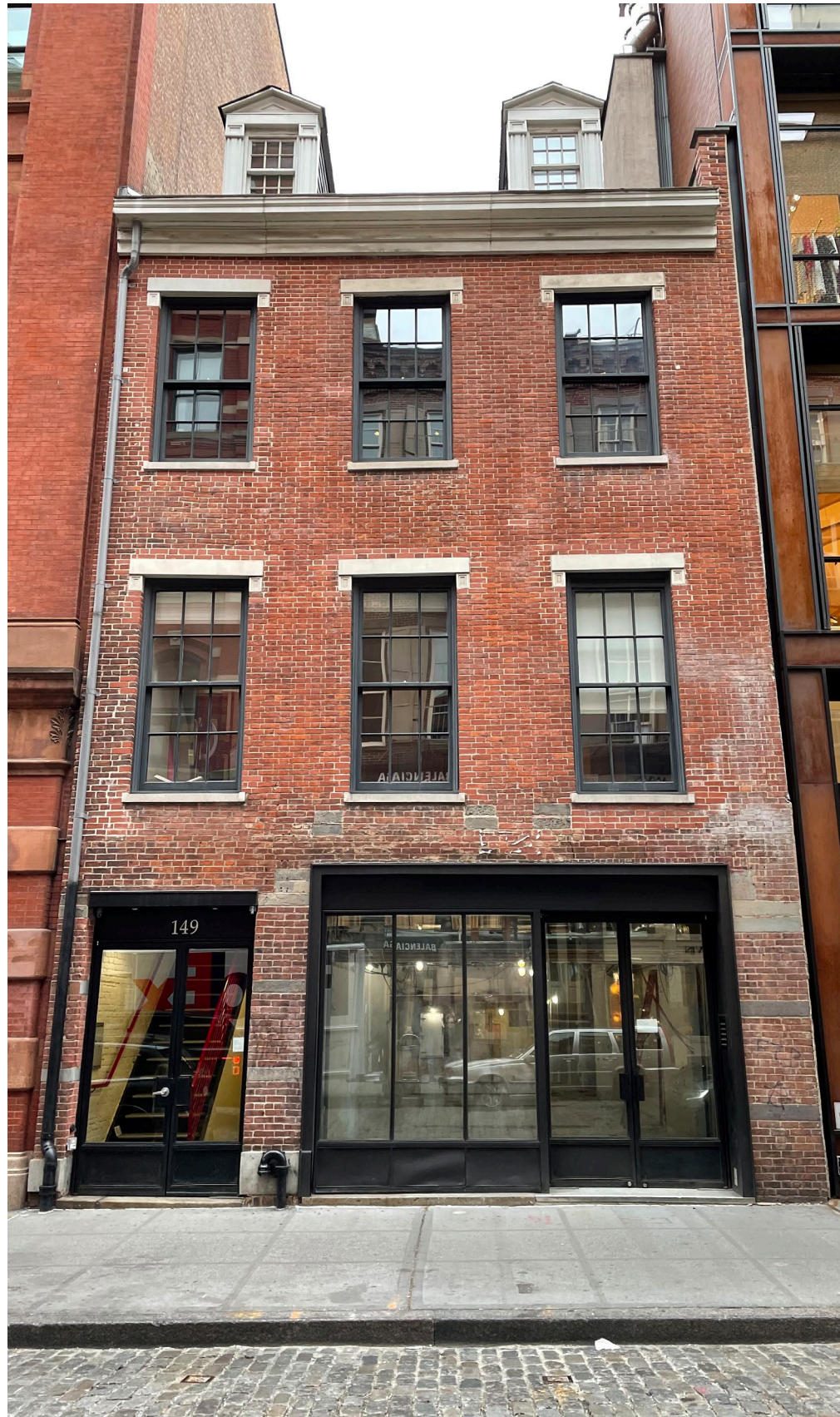
149 Mercer, existing conditions
