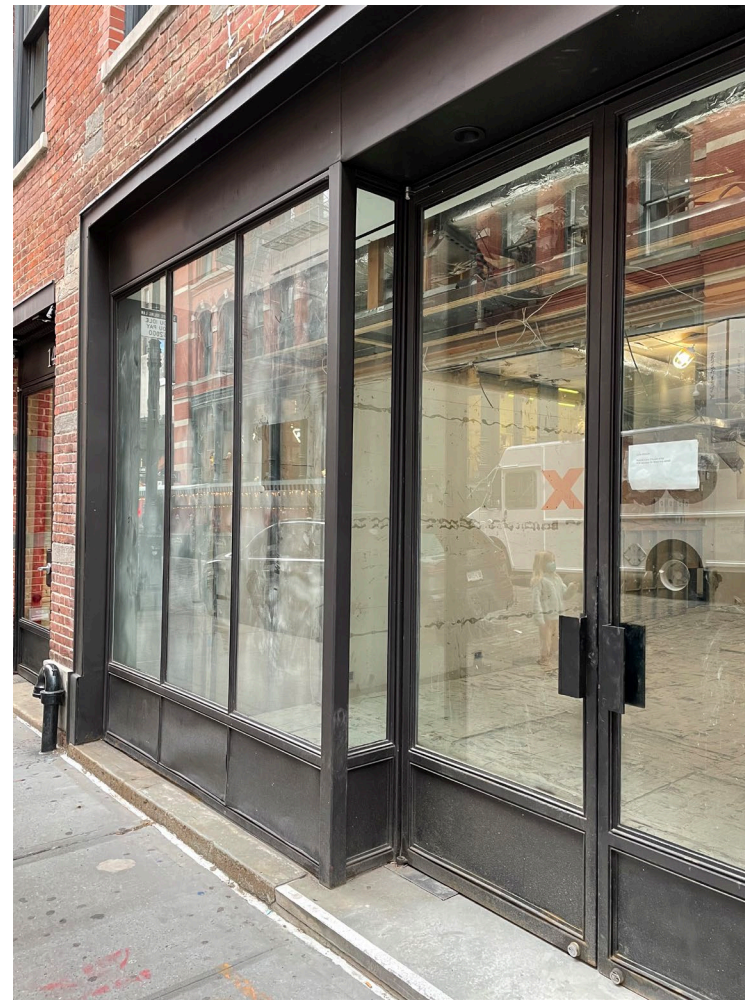
Storefront overview, looking southwest.
