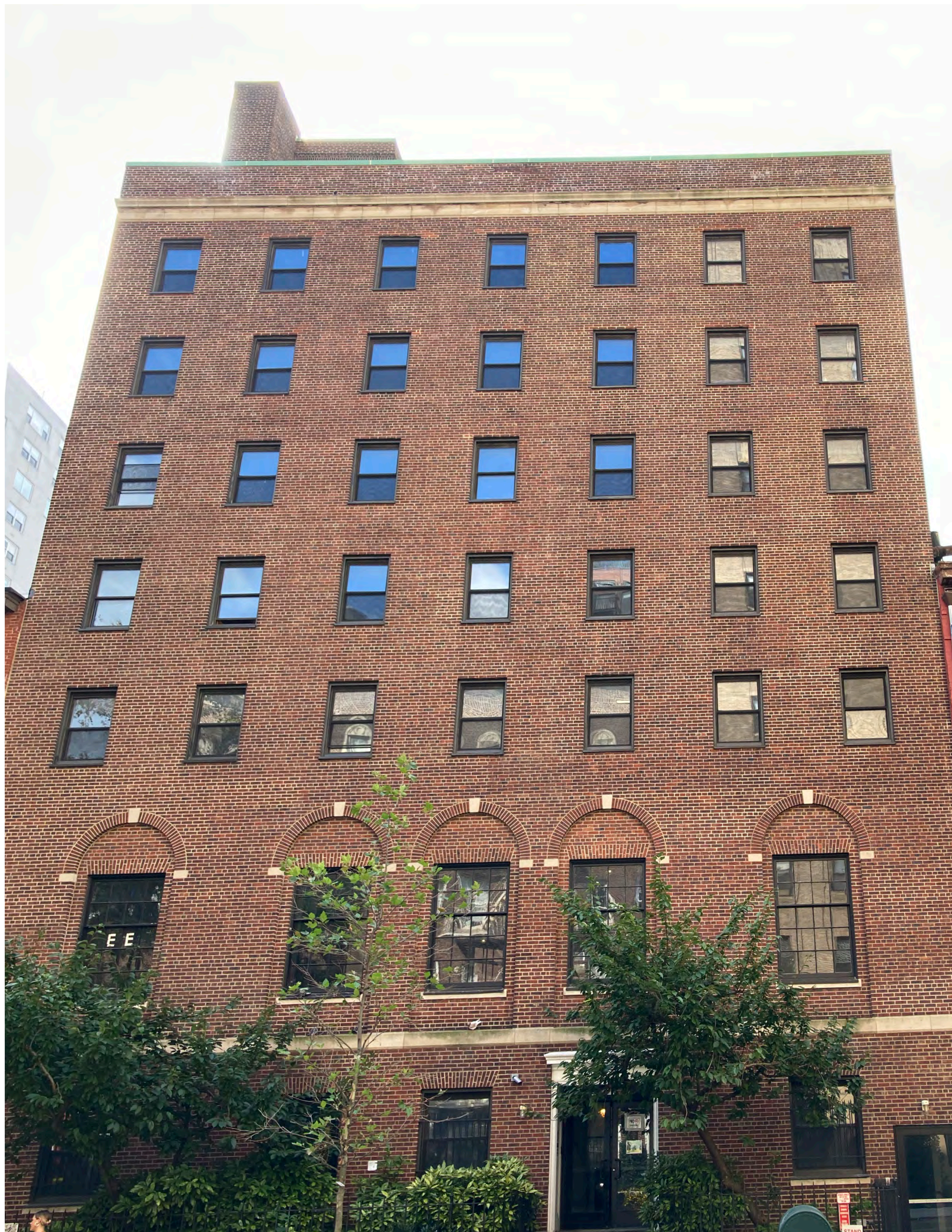
FRONTAL VIEW - EXISTING
