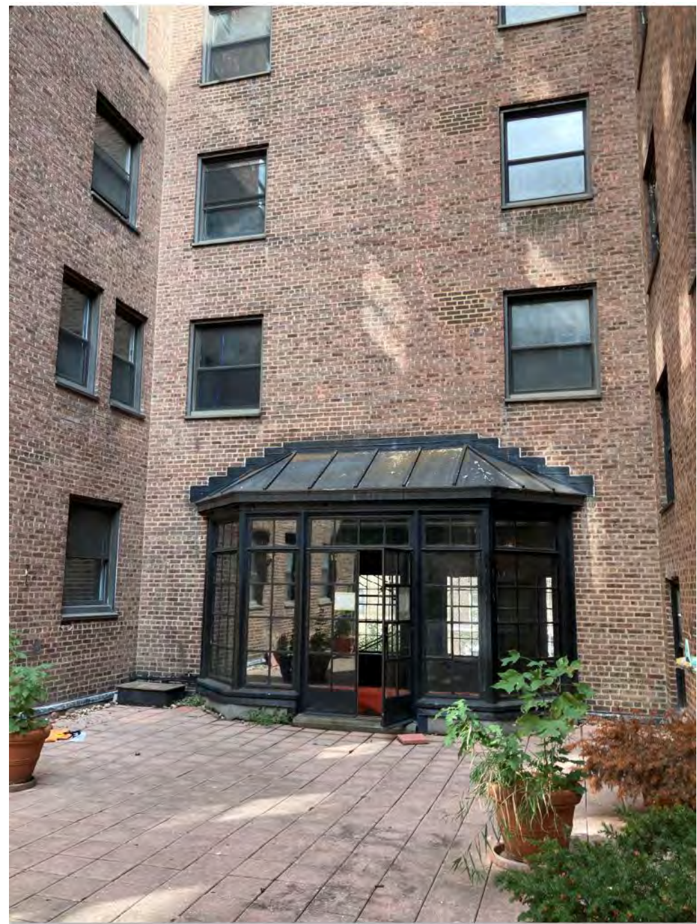
2) COURTYARD NORTH (2ND FLOOR BAY)
