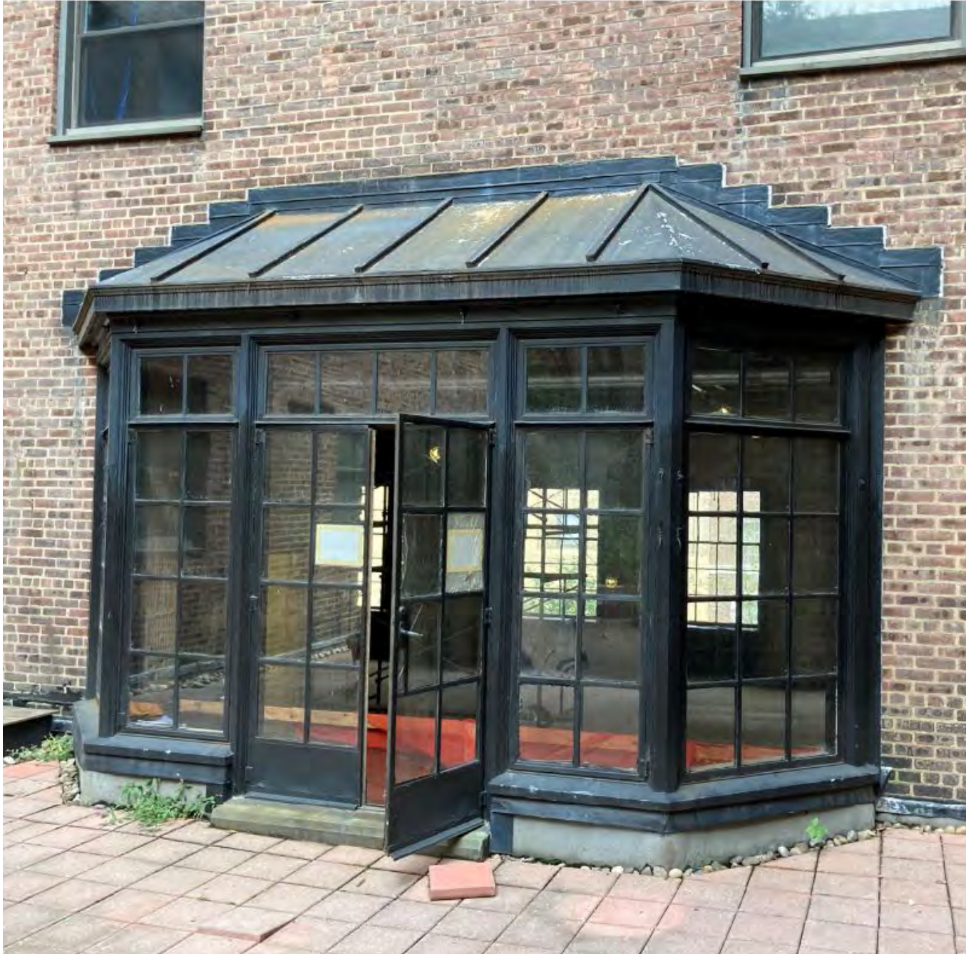
3) COURTYARD NORTH (2ND FLOOR BAY)
