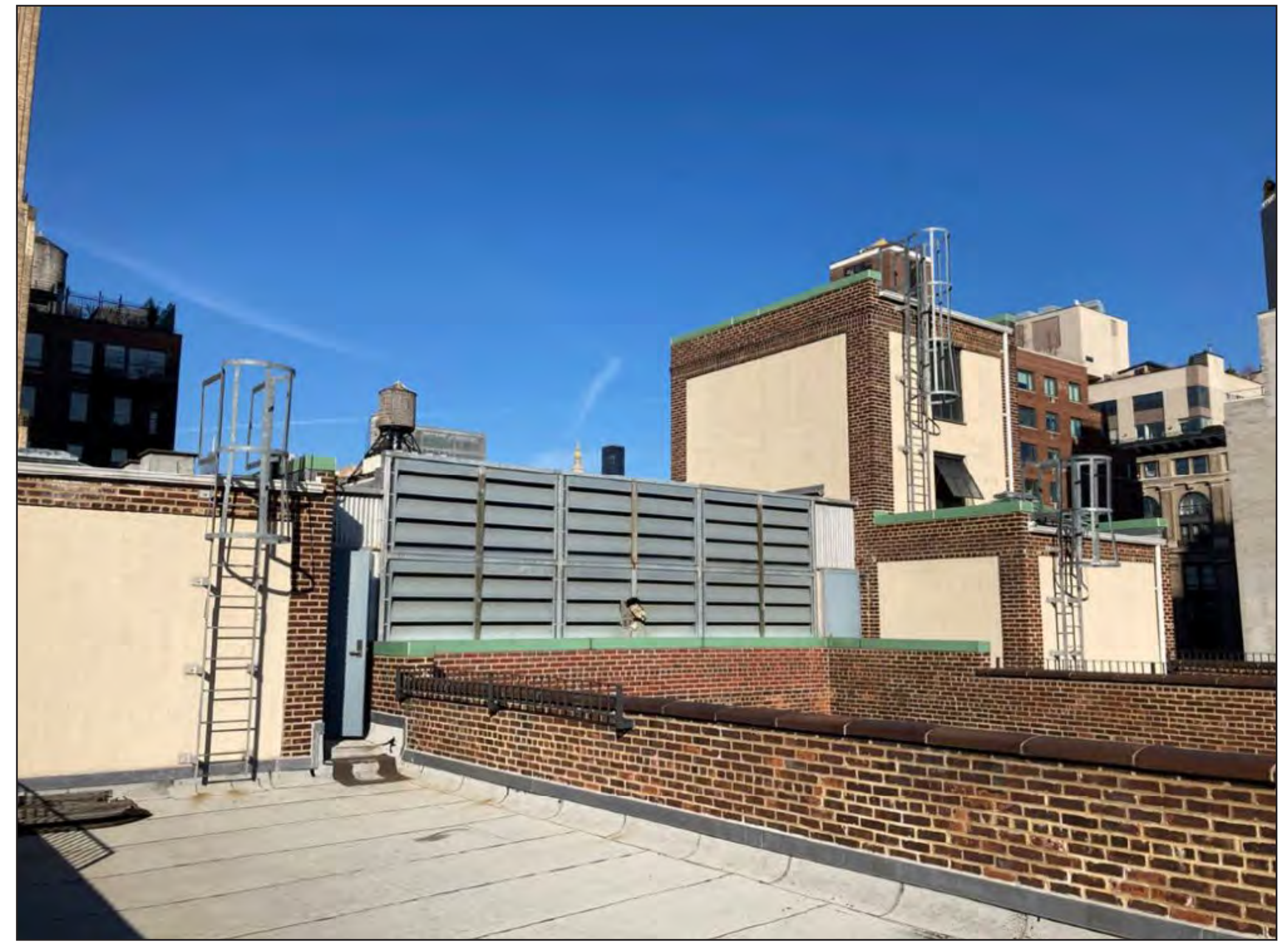
EAST BULKHEAD (VIEW FROM SOUTH WEST)
