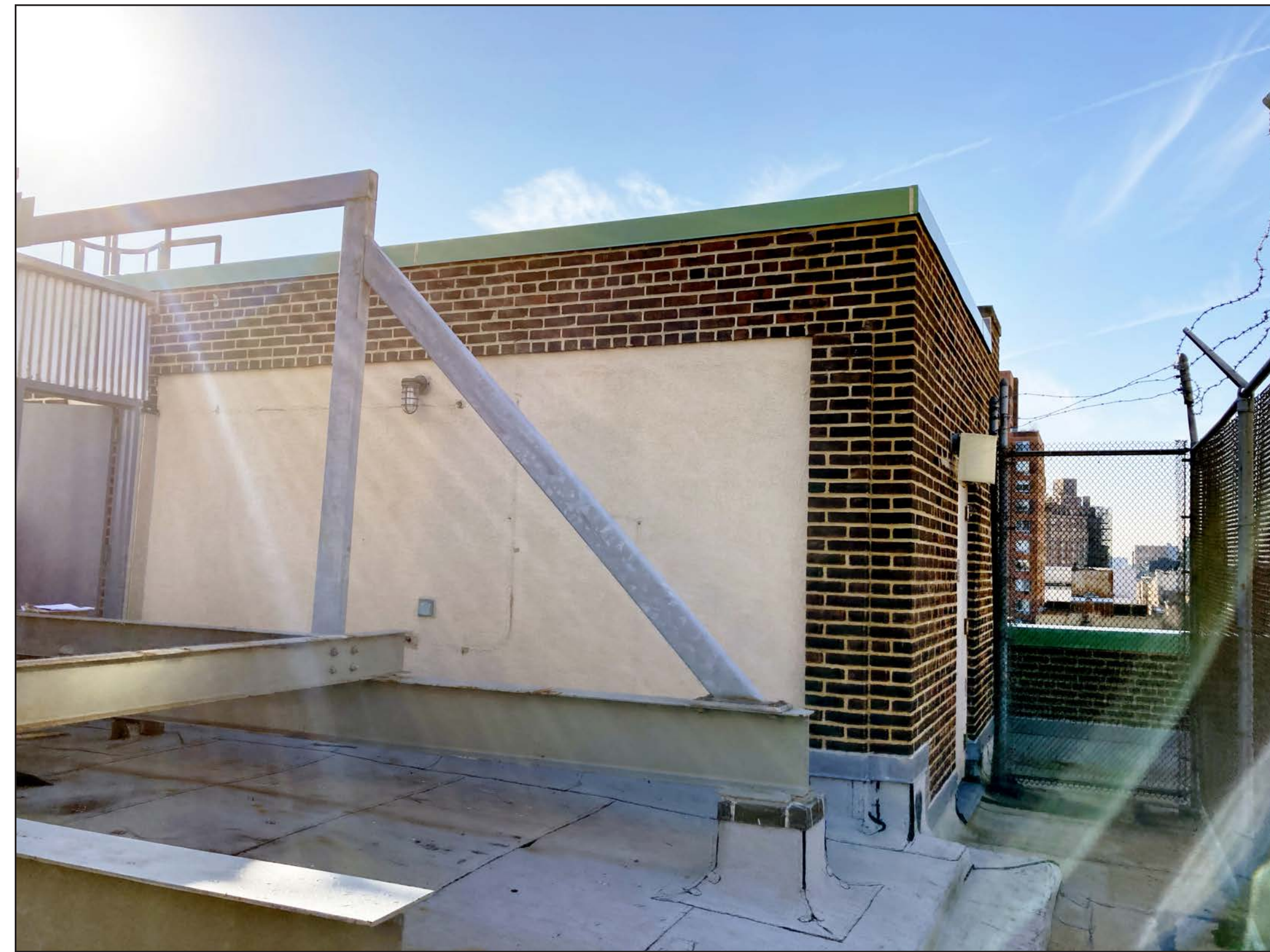
WEST BULKHEAD (VIEW FROM NORTH EAST)
