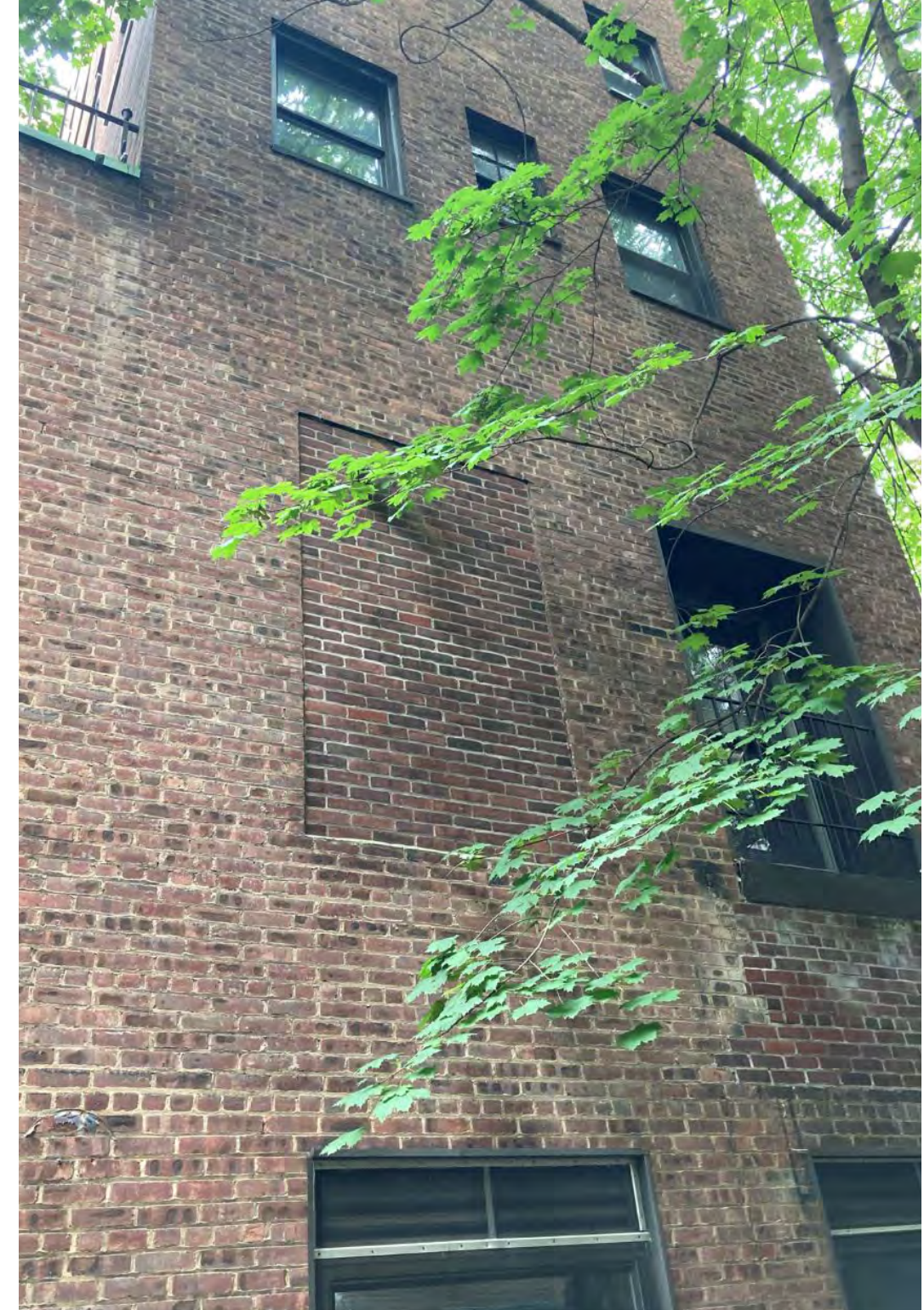
8) SOUTH FACADE AT EAST WING (LOWER FLOORS)
