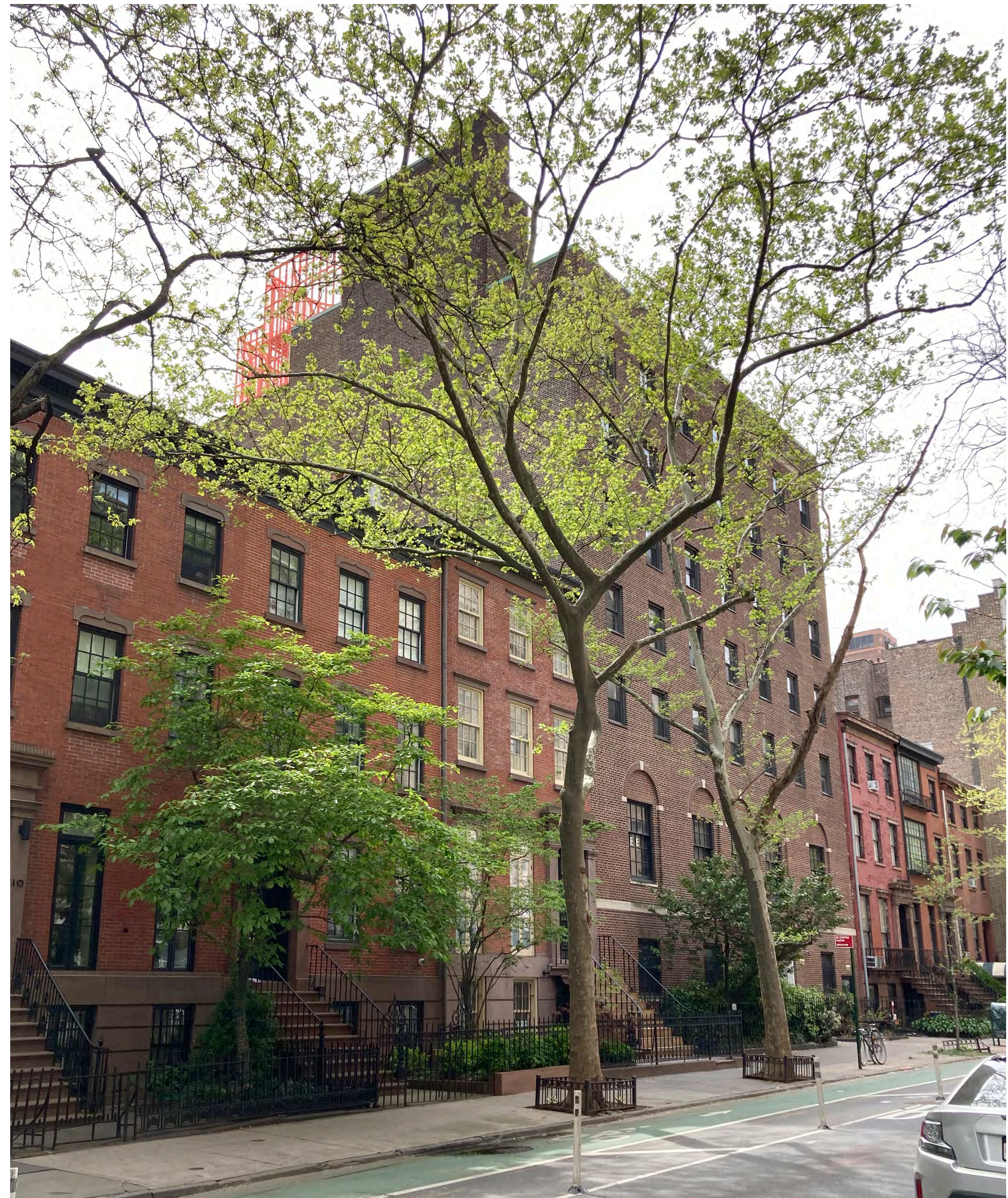
VIEW FROM EAST - WITH MOCKUP
