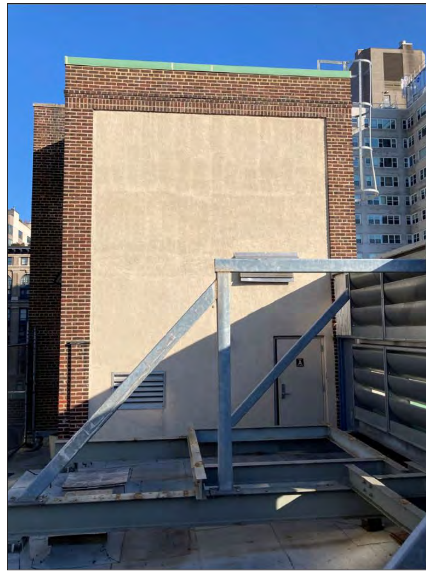
EAST BULKHEAD (VIEW FROM WEST)
