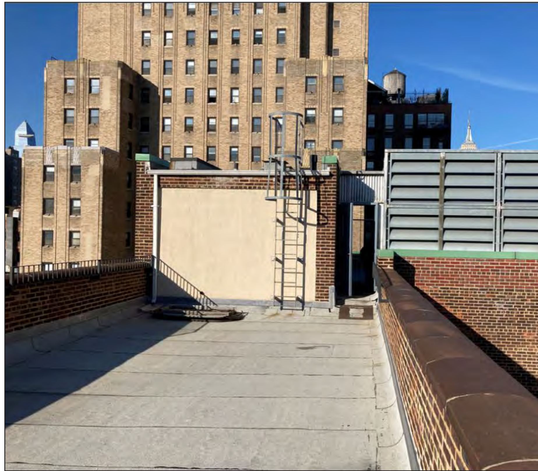
WEST BULKHEAD (VIEW FROM SOUTH)
