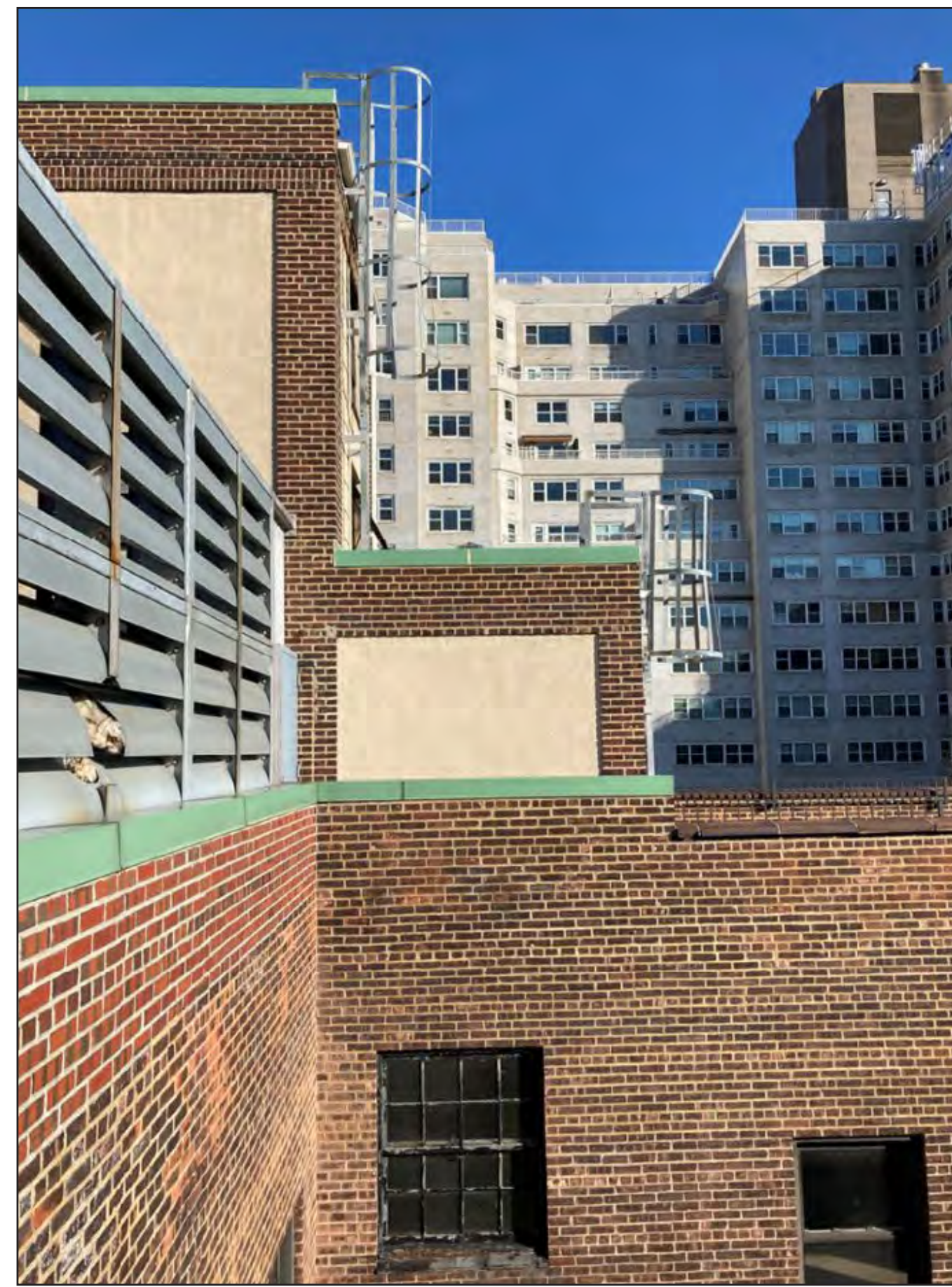
EAST BULKHEAD (VIEW FROM WEST)
