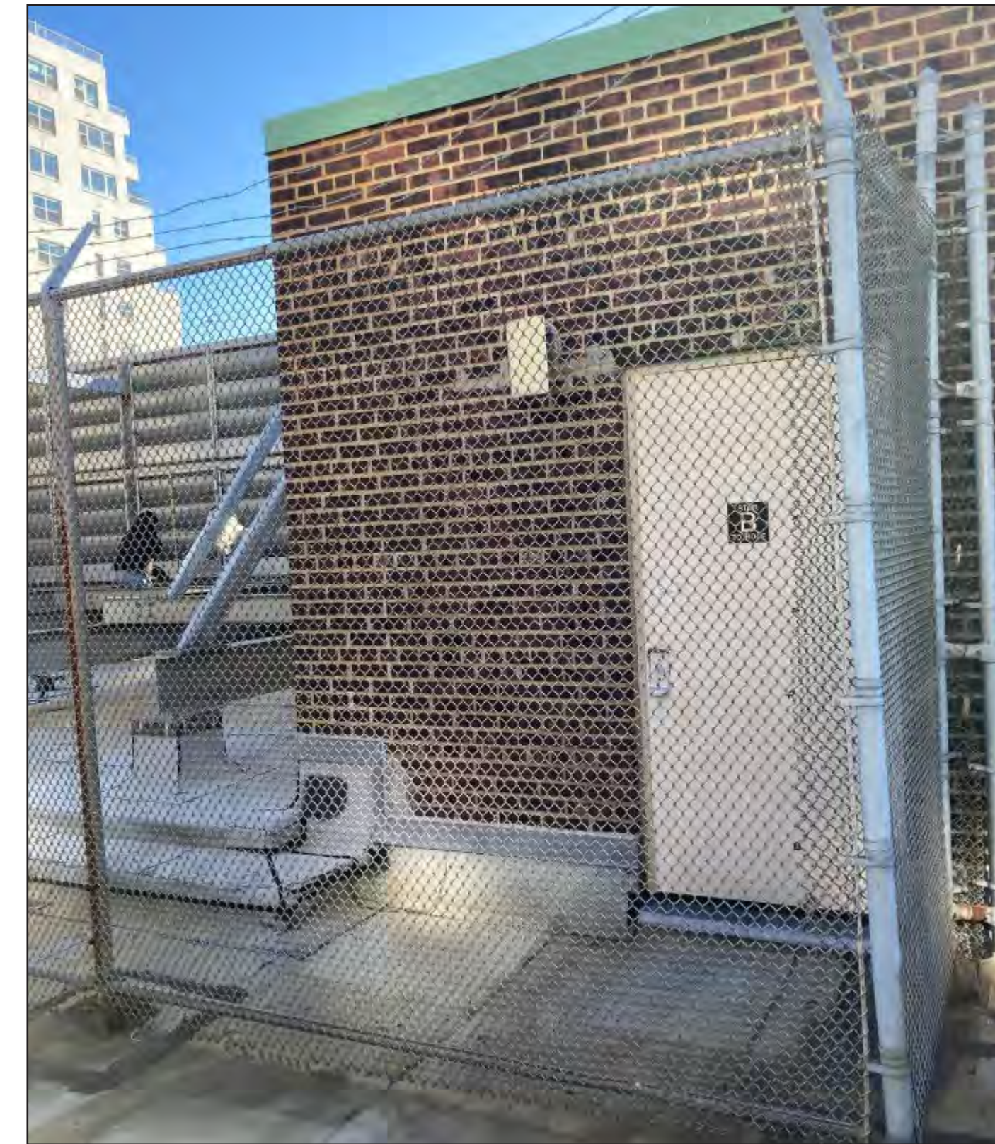
WEST BULKHEAD (VIEW FROM NORTH)
