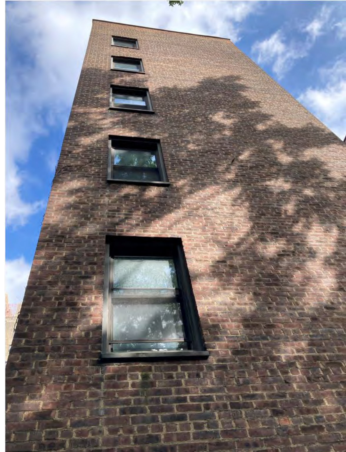
5) SOUTH FACADE AT WEST WING
