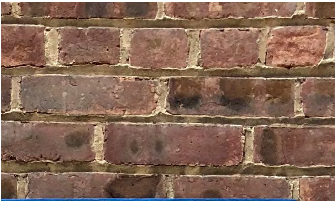
EXISTING COURTYARD BRICK (WITHOUT STAIN)
