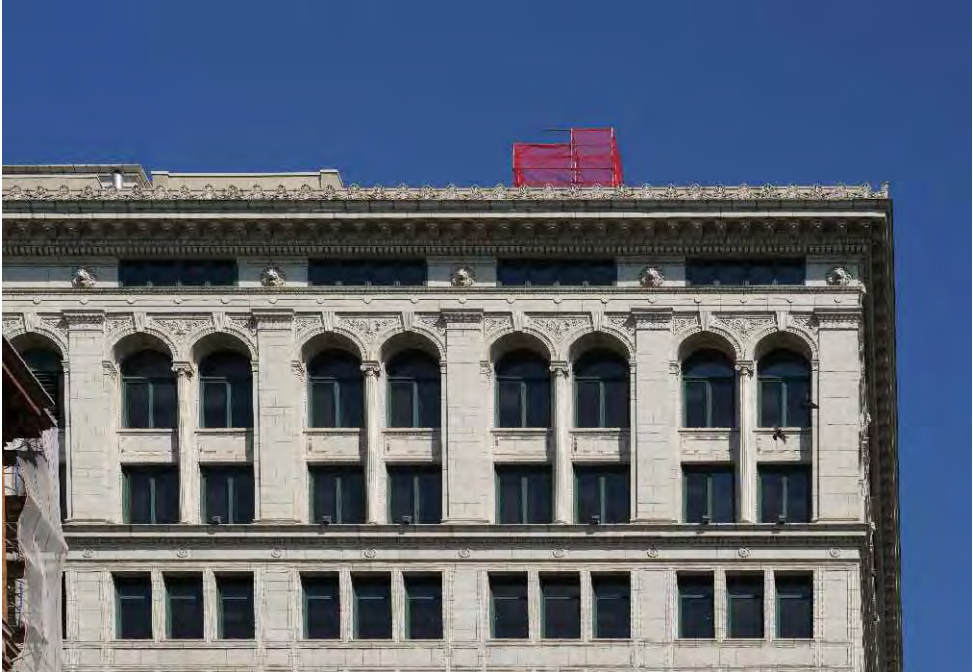
3 COOLING TOWER MOCK-UP PHOTO - ENLARGED NTS
