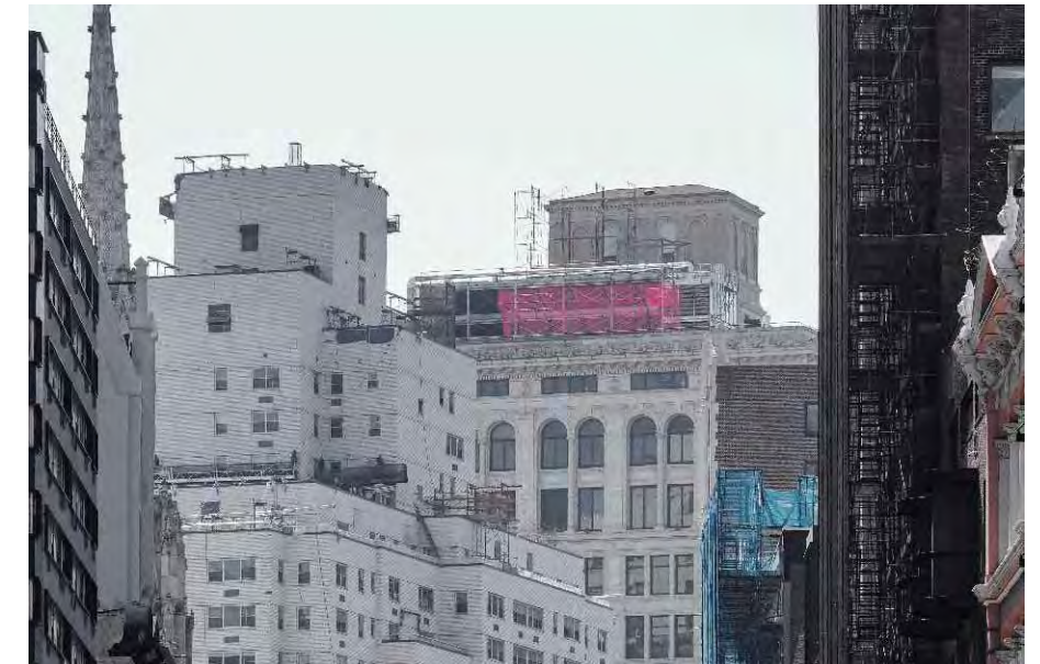
3 GENERATOR MOCK-UP PHOTO - ENLARGED NTS
