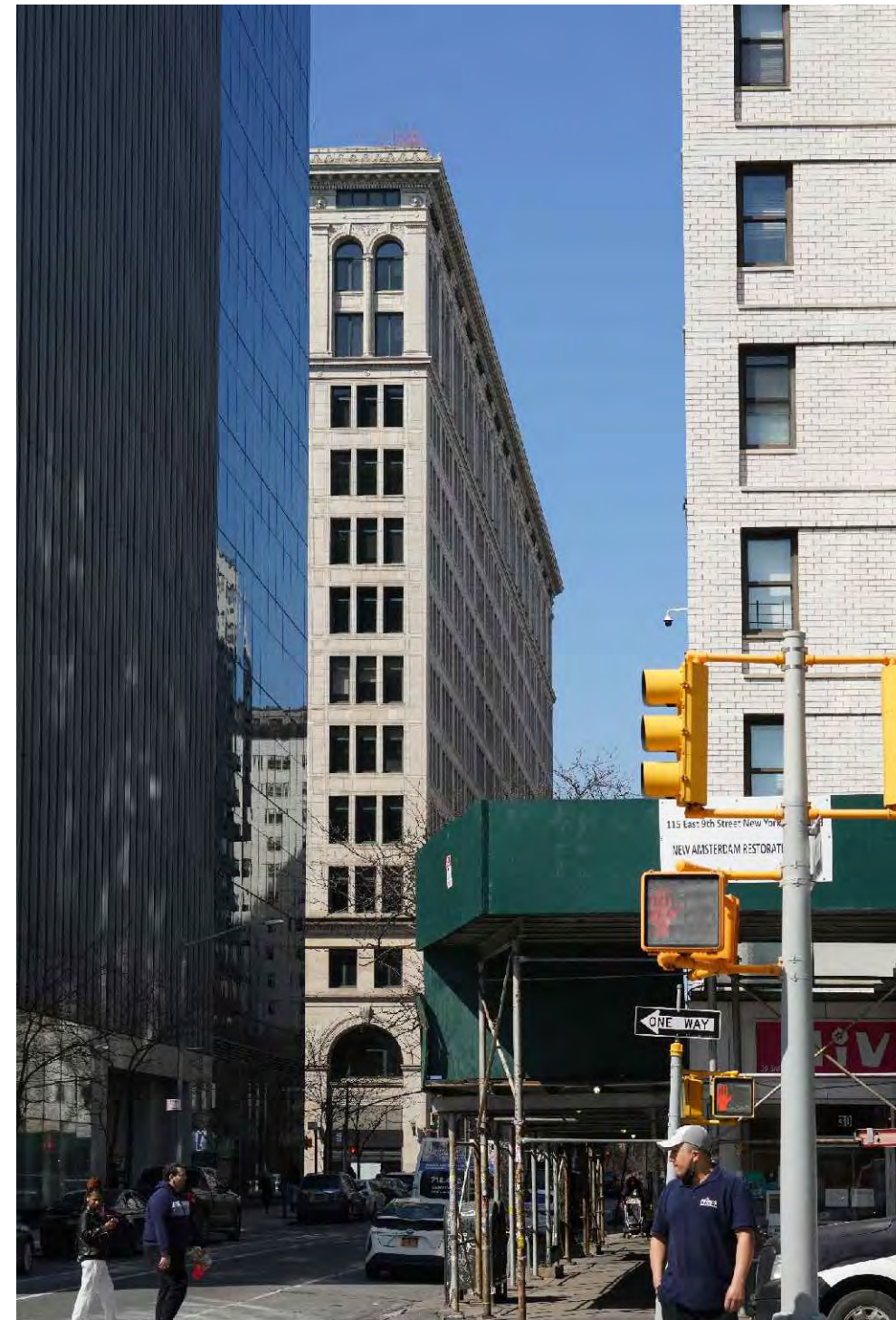
1 GENERATOR MOCK-UP PHOTO FROM EAST 9TH ST. AND 3RD AVE. NTS
