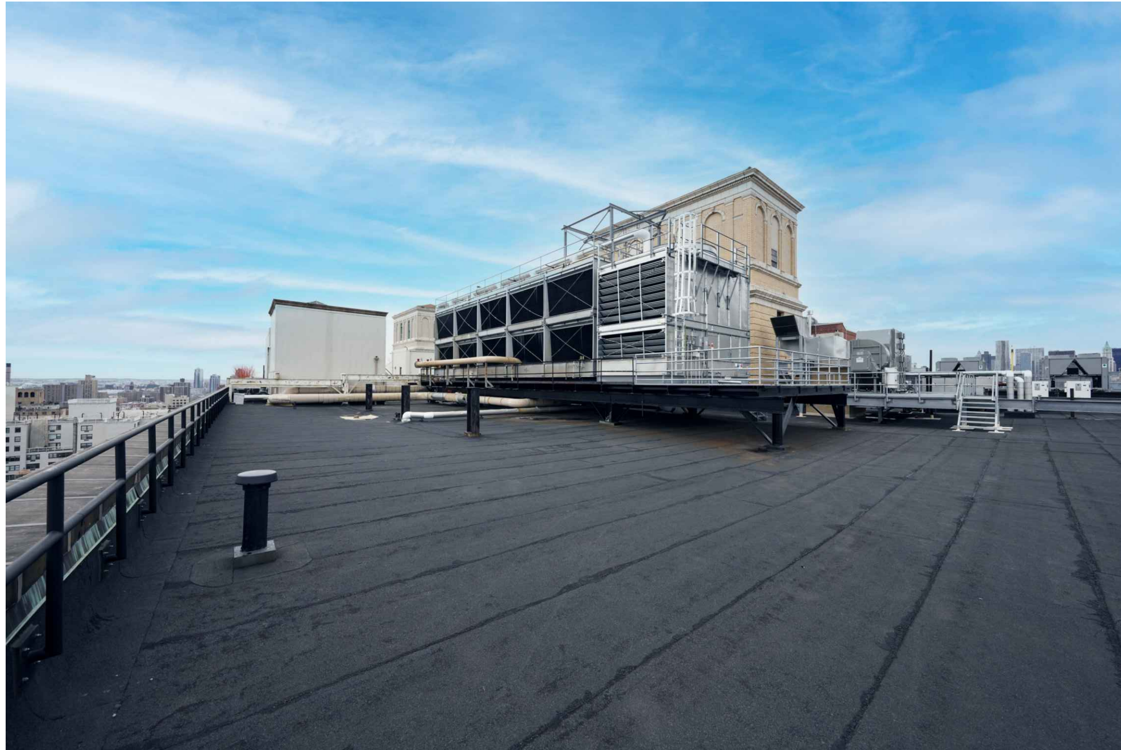
① PHOTO - EXISTING ROOF CONDITIONS NTS
