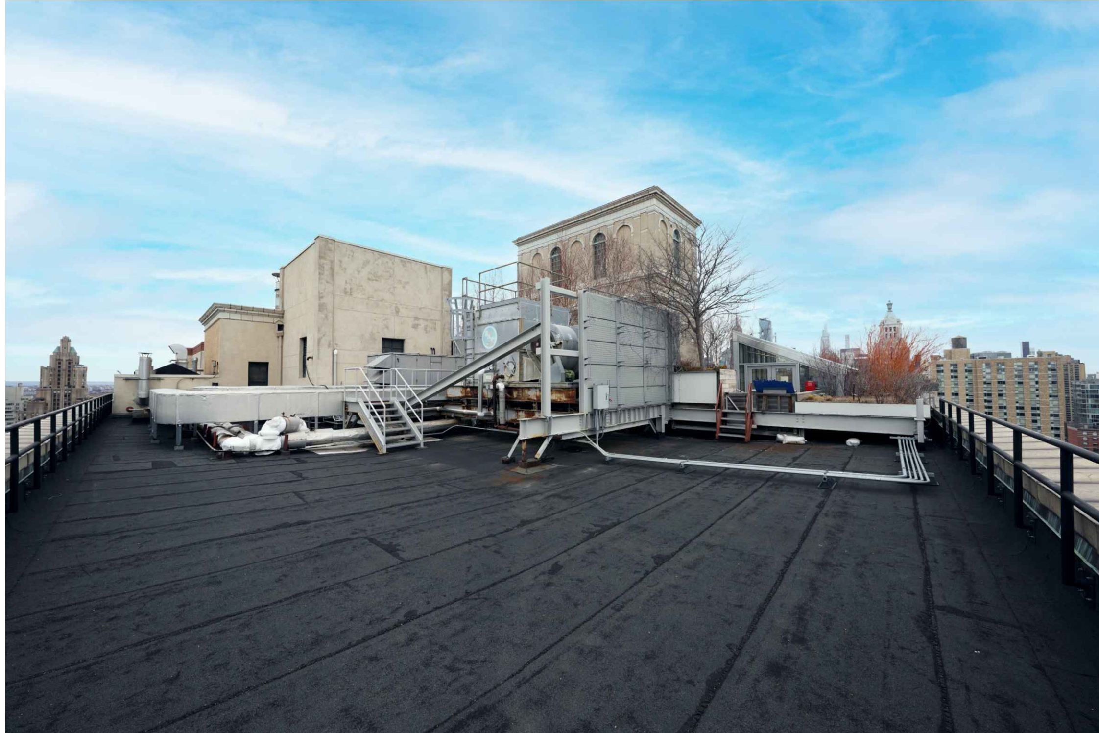
① PHOTO - EXISTING COOLING TOWER TO BE REPLACED NTS
