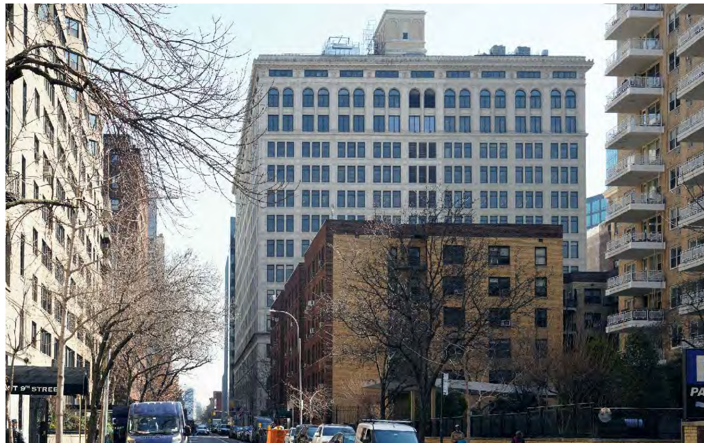
1 GENERATOR MOCK-UP PHOTO FROM 35 EAST 9TH STREET NTS
