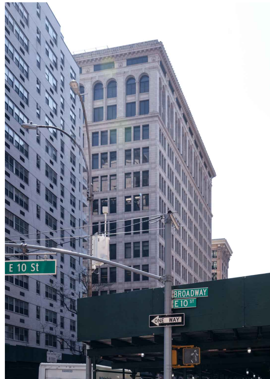
1 GENERATOR MOCK-UP PHOTO FROM 10TH & BROADWAY NTS
