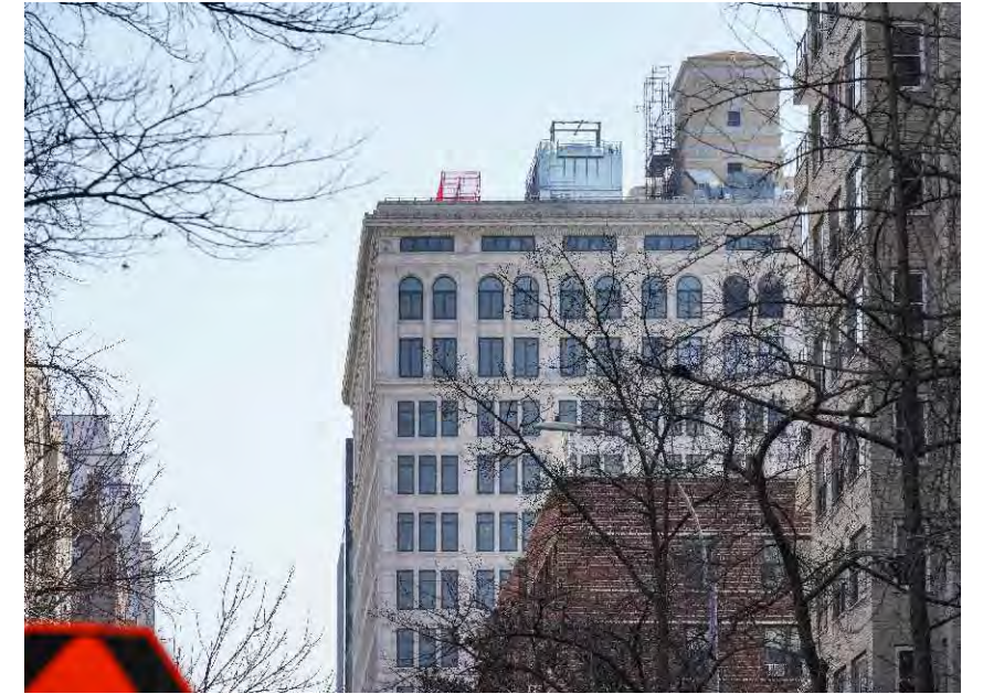
③ GENERATOR MOCK-UP PHOTO - ENLARGED NTS
