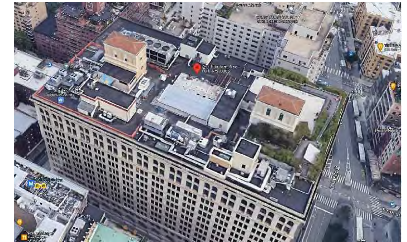
3 AERIAL VIEW FROM SOUTH EAST NTS
