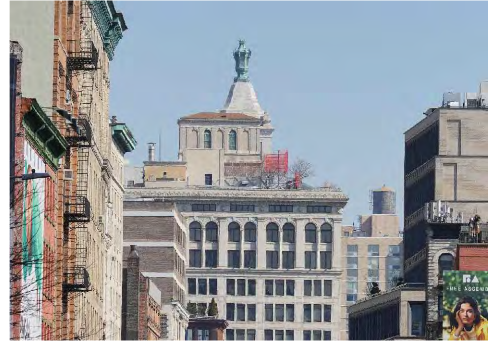
3 COOLING TOWER MOCK-UP PHOTO - ENLARGED NTS
