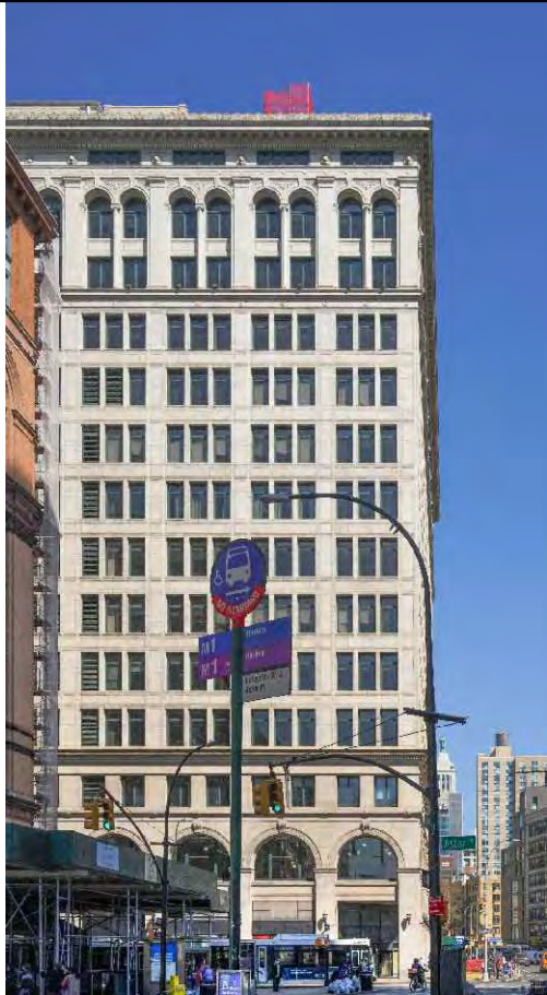
1 COOLING TOWER MOCK-UP PHOTO FROM 425 LAFAYETTE NTS
