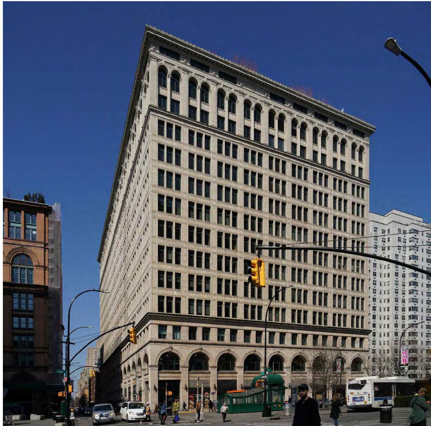
3 COOLING TOWER MOCK-UP PHOTO FROM STREET - FROM ASTOR PLACE AT COOPER SQUARE NTS
