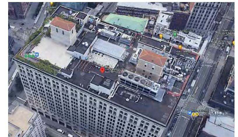
4 AERIAL VIEW FROM NORTH WEST NTS
