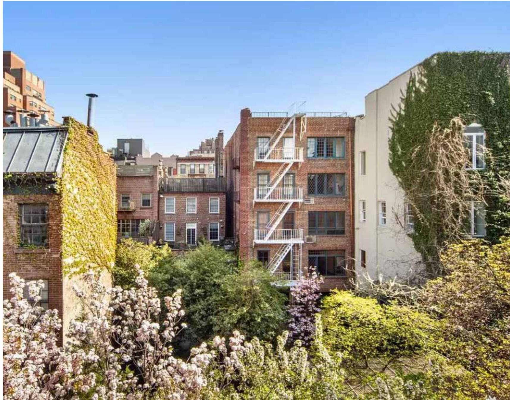
G 31 Perry East Facade (Looking Southwest from 226 West 11th)
