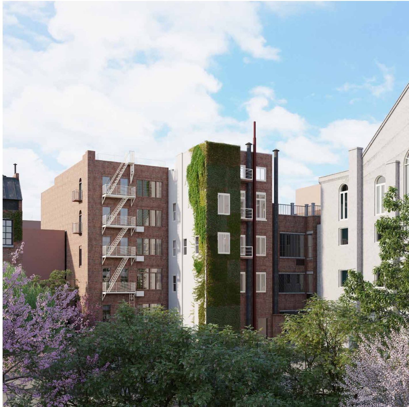
Existing Rear Massing from Northeast
