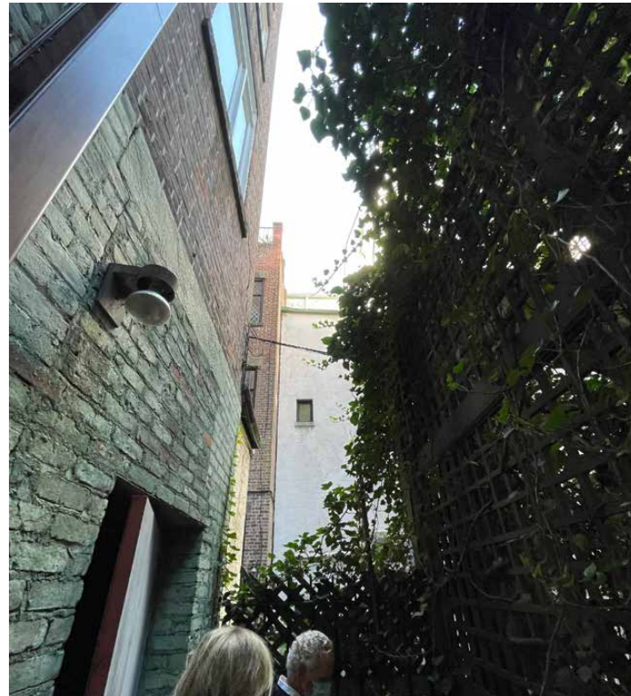
D 31 Perry Rear Elevation (Looking Southwest)
