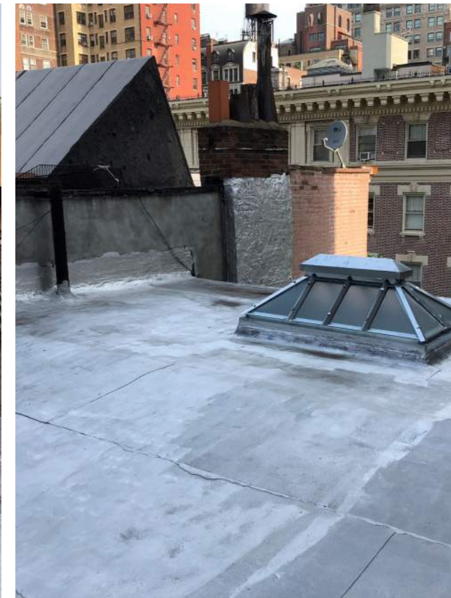
From high roof looking northwest
