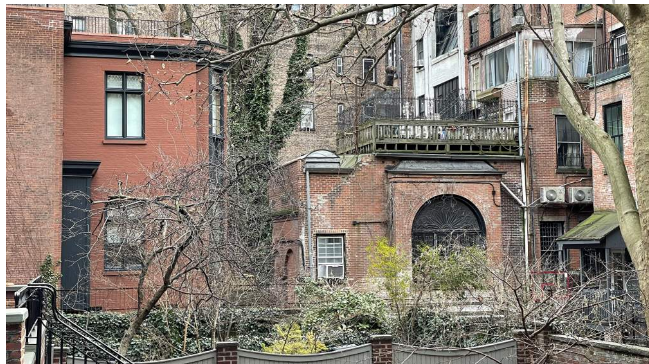
16 East 10th (Pen and Brush at left) and 15 East 9th rear additions at right
