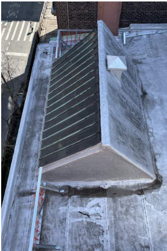
From 22 East 10th looking east
