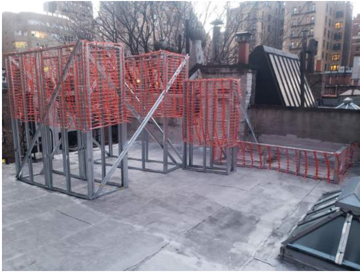
HVAC and elevator overrun mockup
