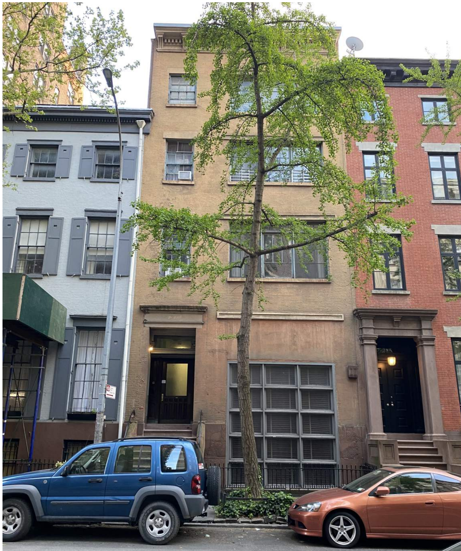
Front facade existing
