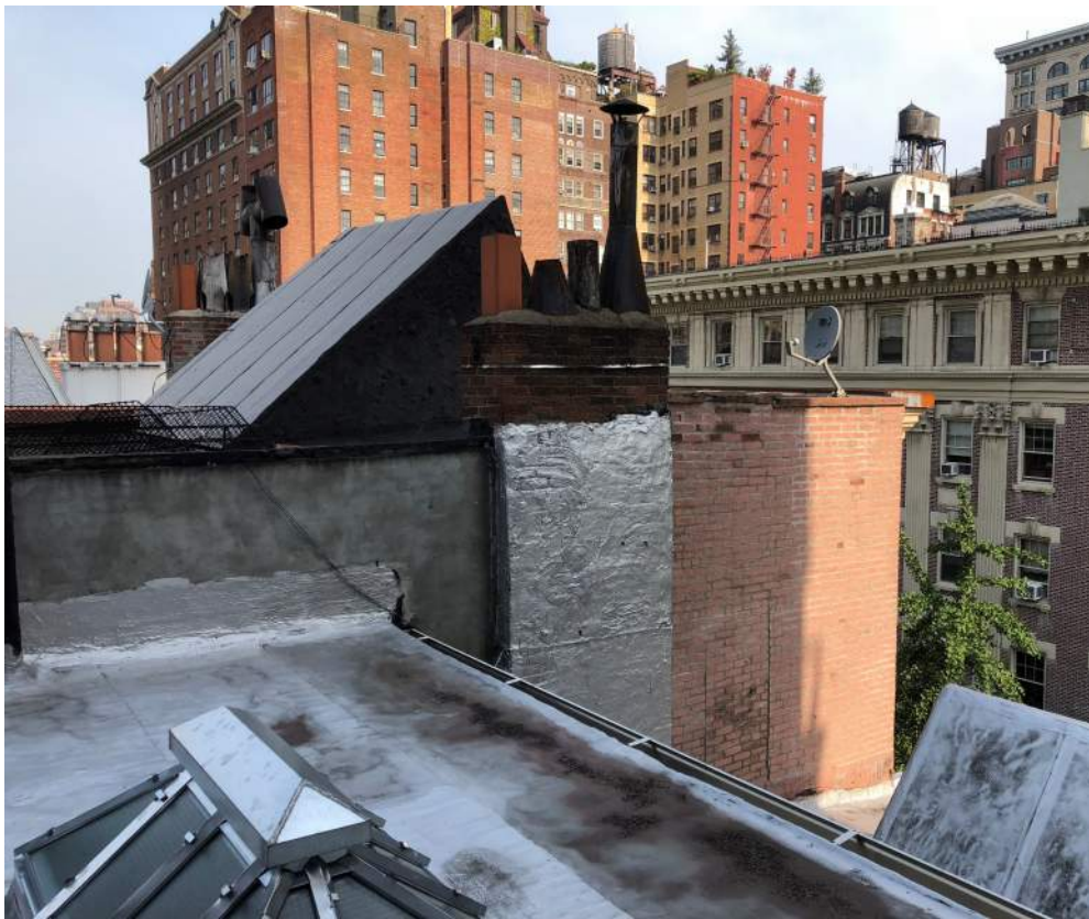
From high roof looking northwest
