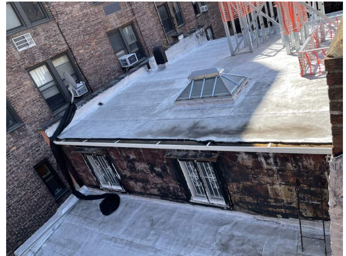
Existing fourth floor front facade
