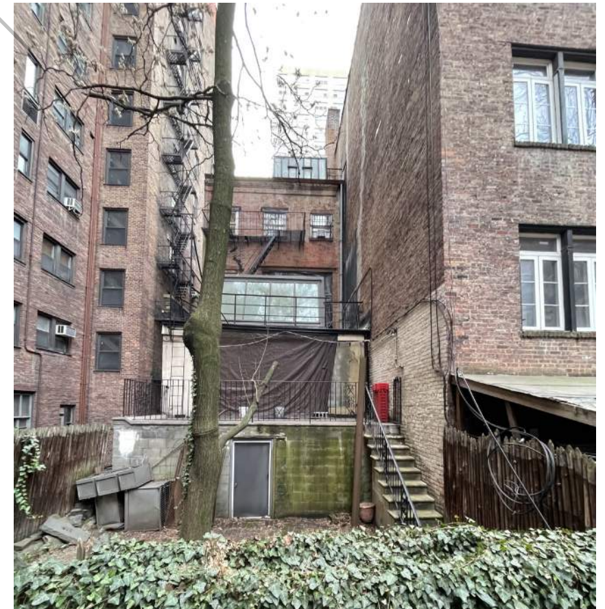
23 East 9th Rear Additions
