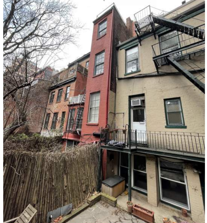
18-24 East 10th from 24 East 10th rear yard
