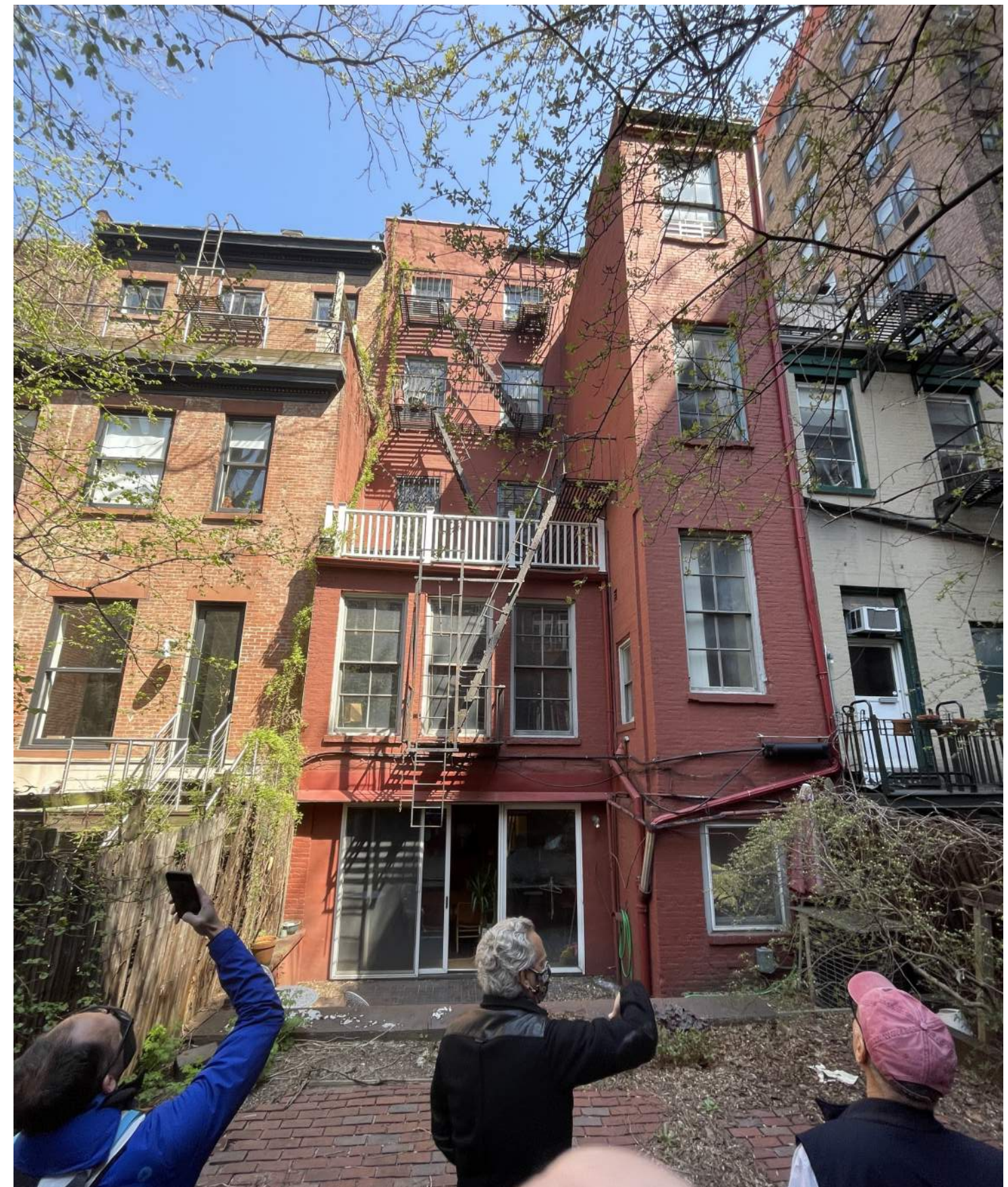
Rear facade existing
