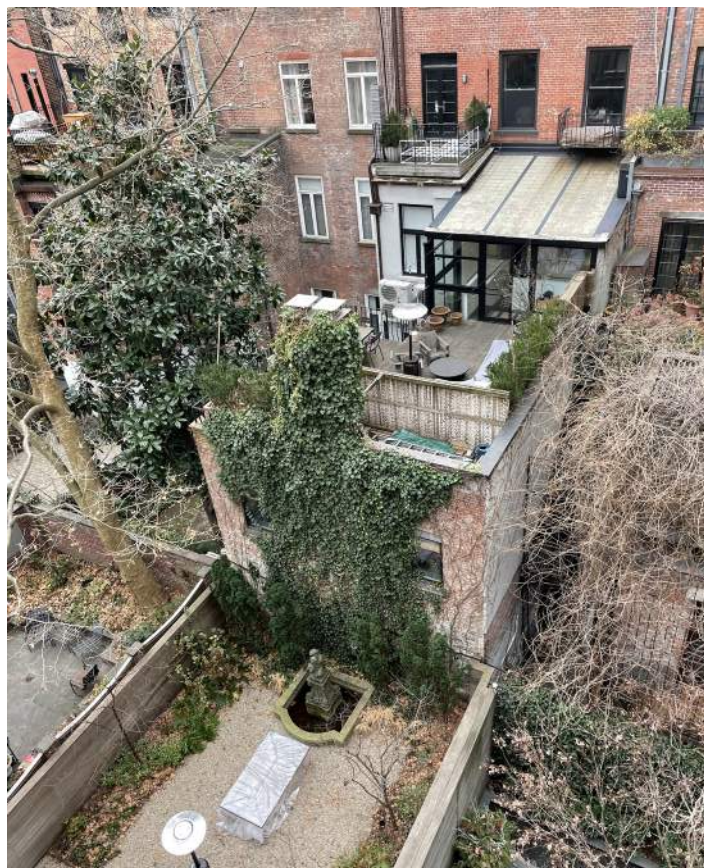
7 East 9th lot-line back house / rear additions
