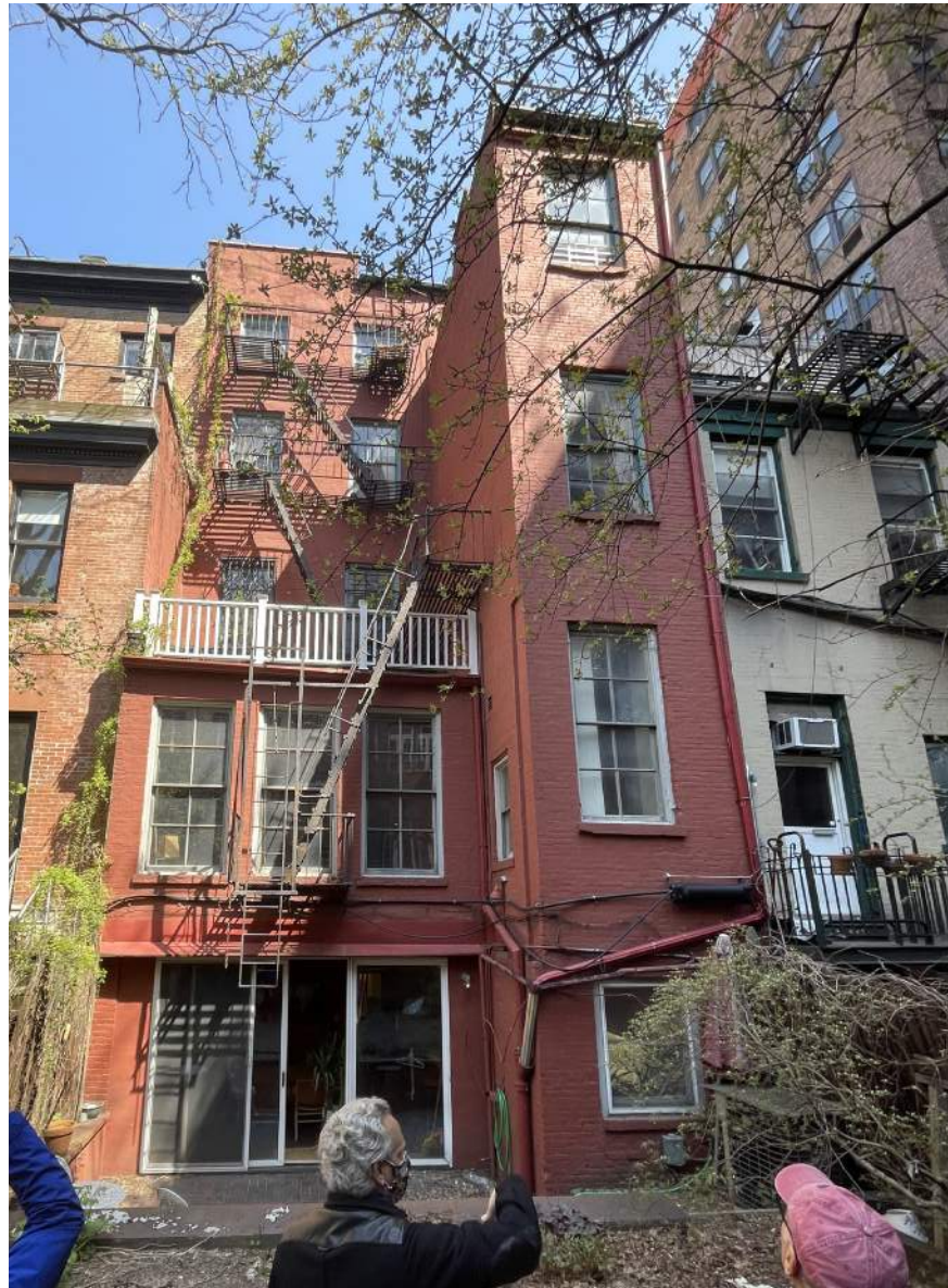
Existing rear facade photo
