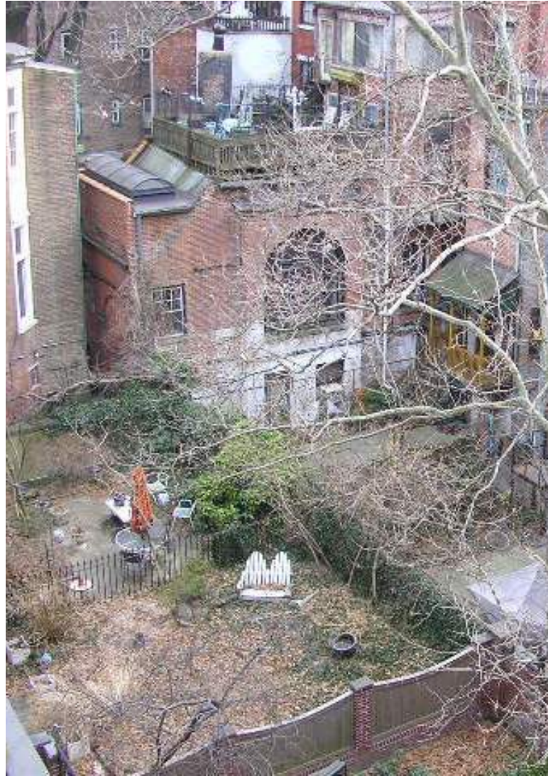
15 East 9th Street rear additions from 10th Street roof
