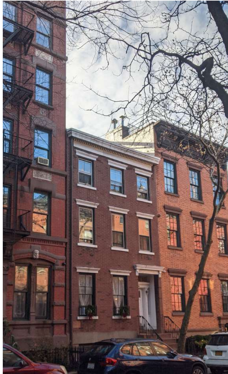
01. TO THE EAST OF 90 CHARLES FRONT FACADE (NORTH)
