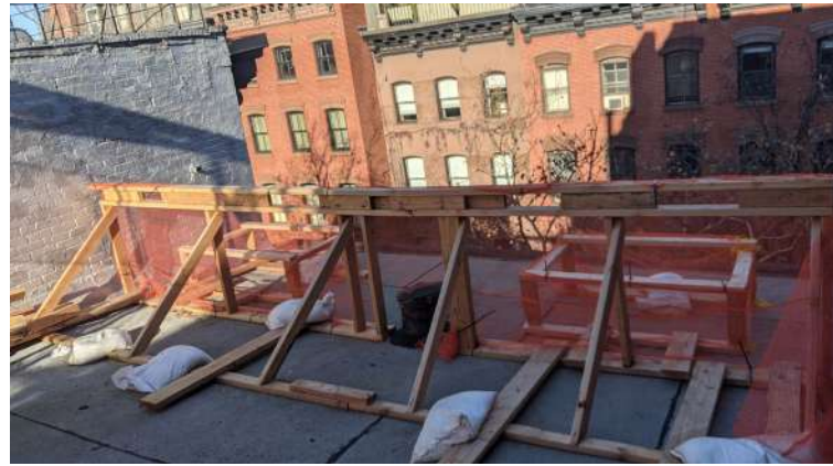
PARAPET & SKYLIGHT MOCK-UP
