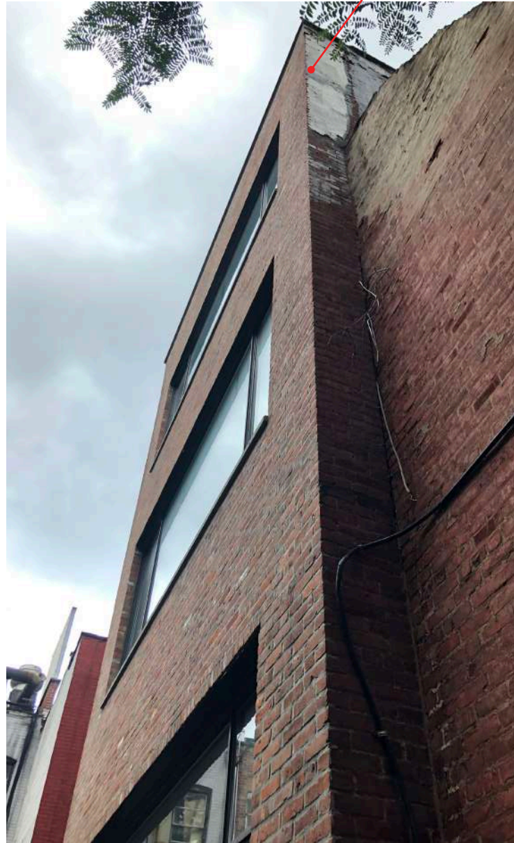
92 CHARLES STREET - REAR FACADE (SOUTH)
