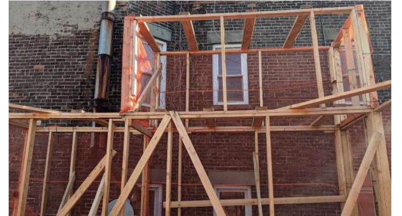
MECHANICAL BULKHEAD MOCK-UP
