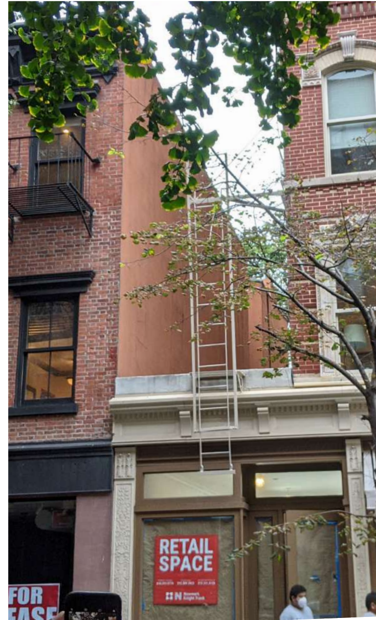
06. THROUGH VIEW FROM 355 BLEECKER STREET
