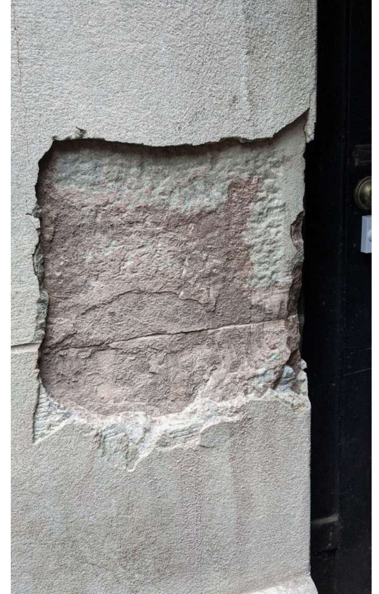
HISTORIC MASONRY EXPOSURE TEST ON BROWNSTONE
