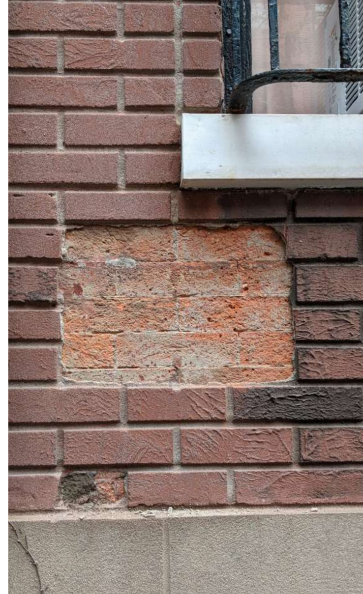
HISTORIC BRICK EXPOSURE TEST ON 1960'S FACE BRICK
