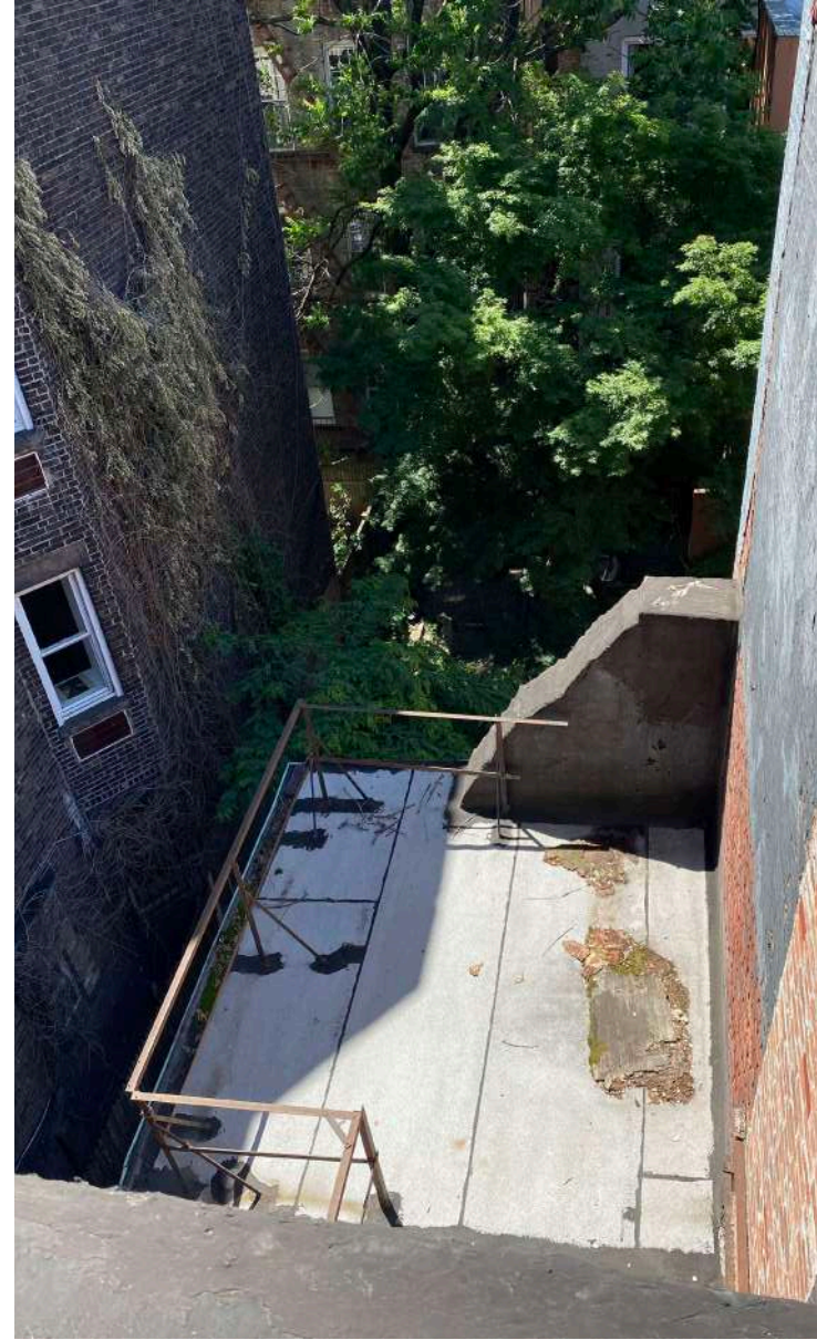
REAR YARD AND ADDITION FROM ROOF
