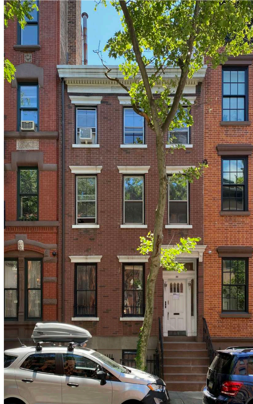
EXISTING BUILDING FROM CHARLES STREET
