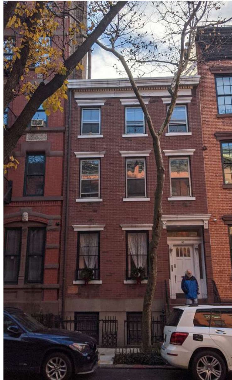
02. 90 CHARLES STREET - FRONT FACADE (NORTH)
