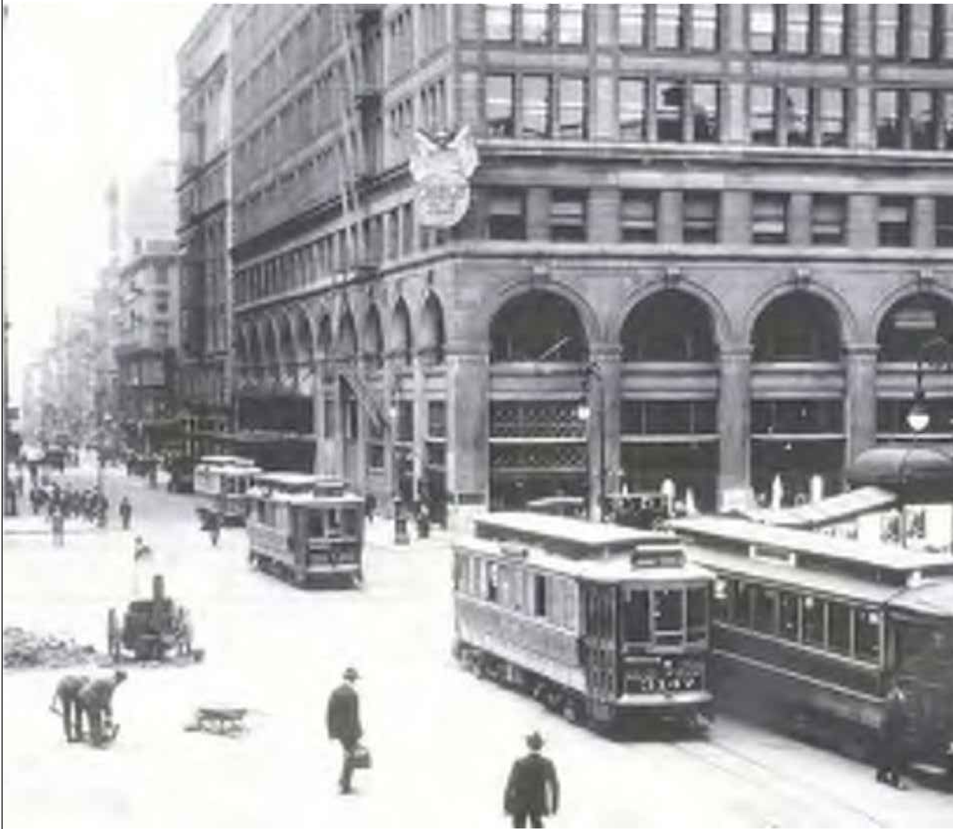
1 HISTORICAL PHOTOGRAPH - 8TH & LAFAYETTE STREET - 1913 NTS
