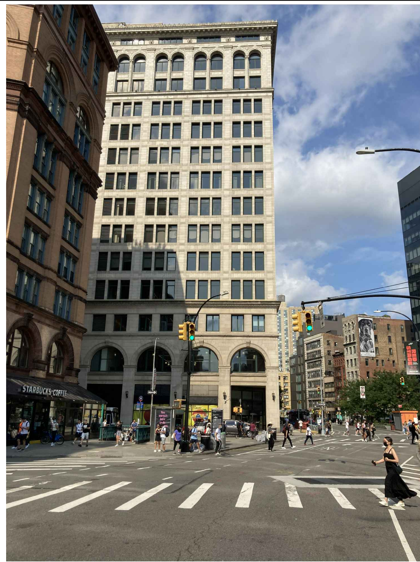
1 PHOTOGRAPH - SOUTH ELEVATION NTS
