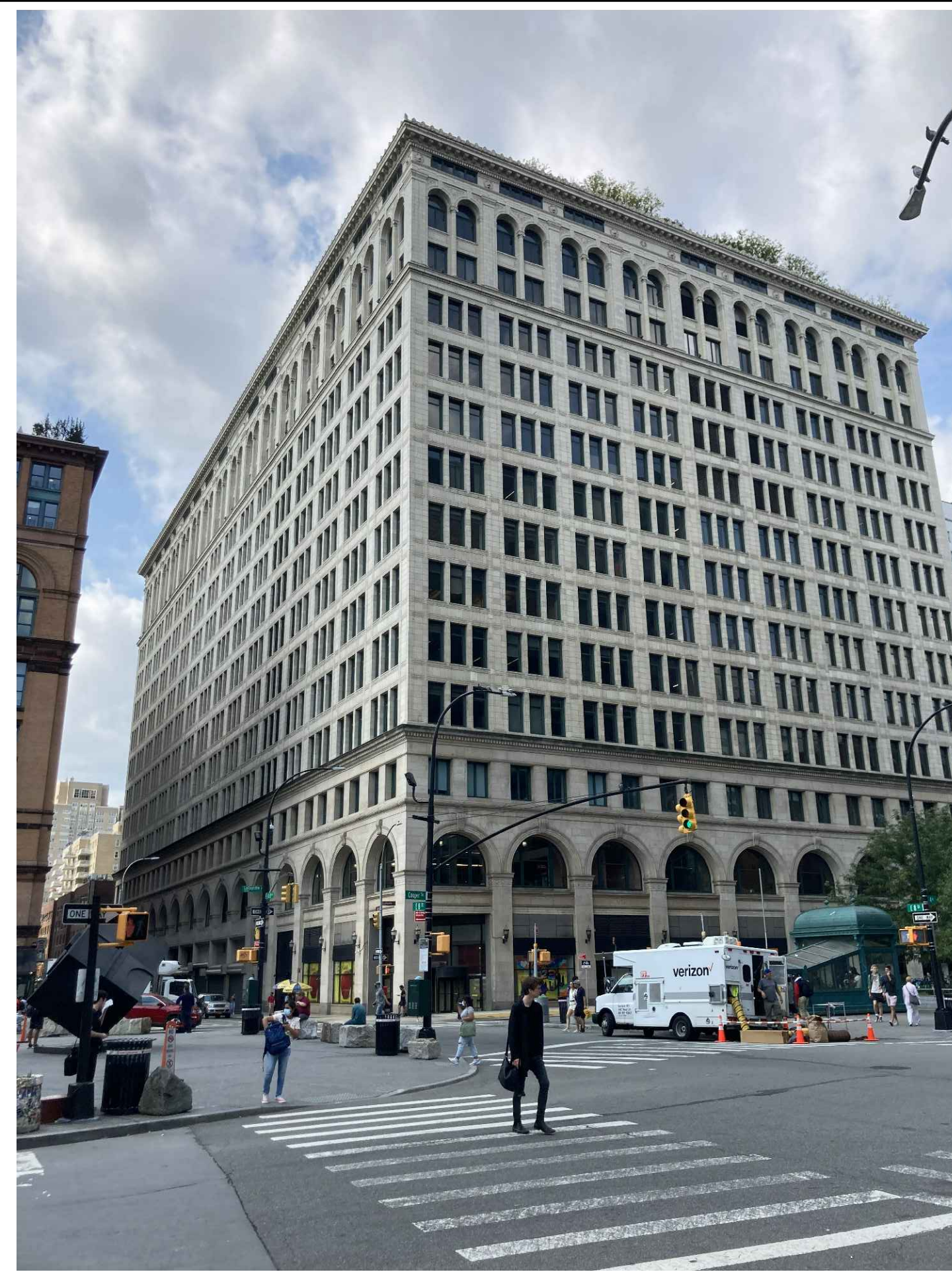
2 PHOTOGRAPH - SOUTH-EAST CORNER NTS
