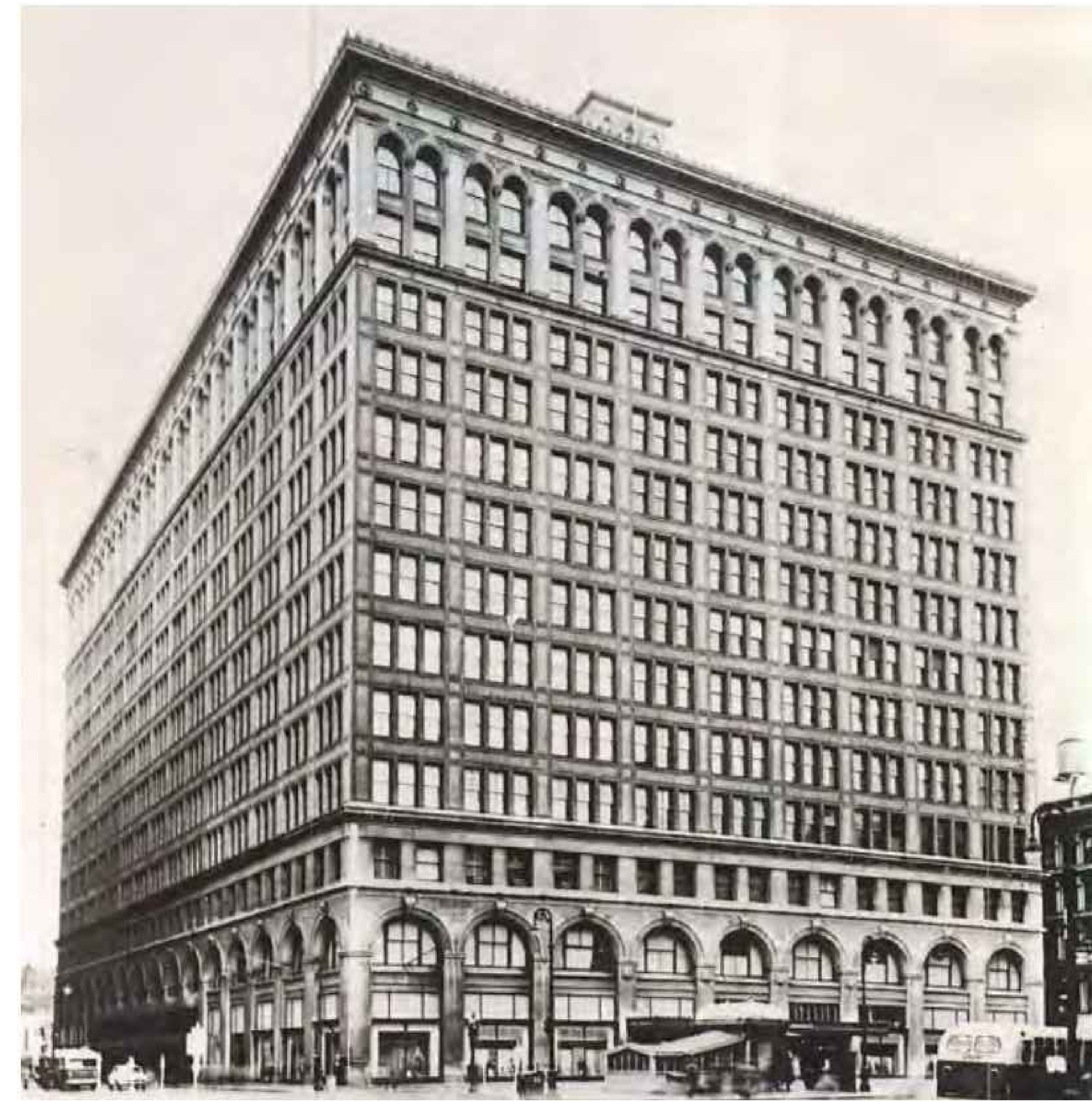
2 HISTORICAL PHOTOGRAPH - 8TH & LAFAYETTE STREET - 1933 NTS
