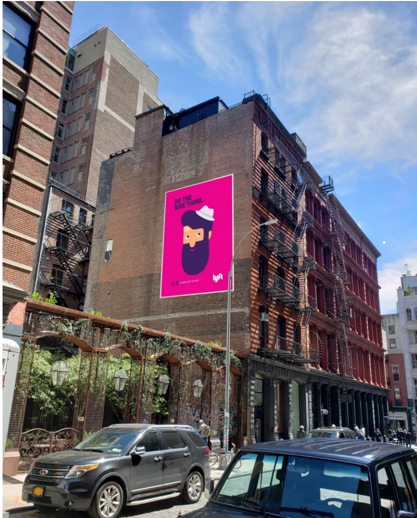
5 Crosby Srteet's north lot line wall.
