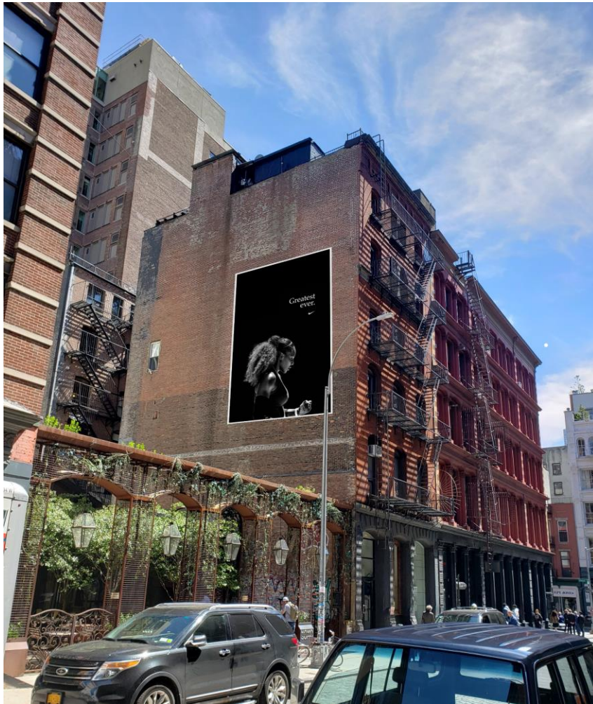
5 Crosby Street's north lot line wall.
