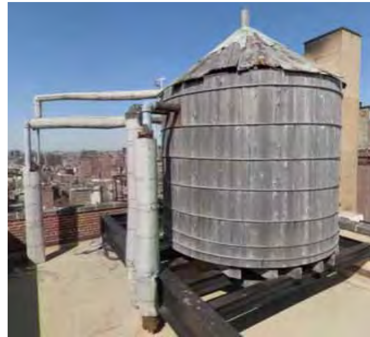
EXISTING WOOD WATER TANK
