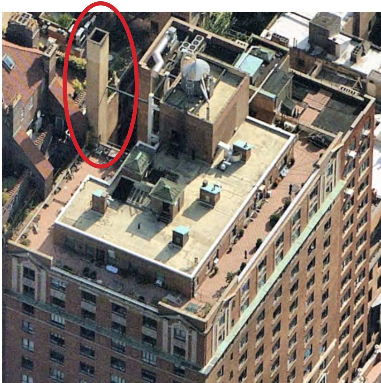
AERIAL VIEW OF ROOF - VIEW TO NORTHEAST
