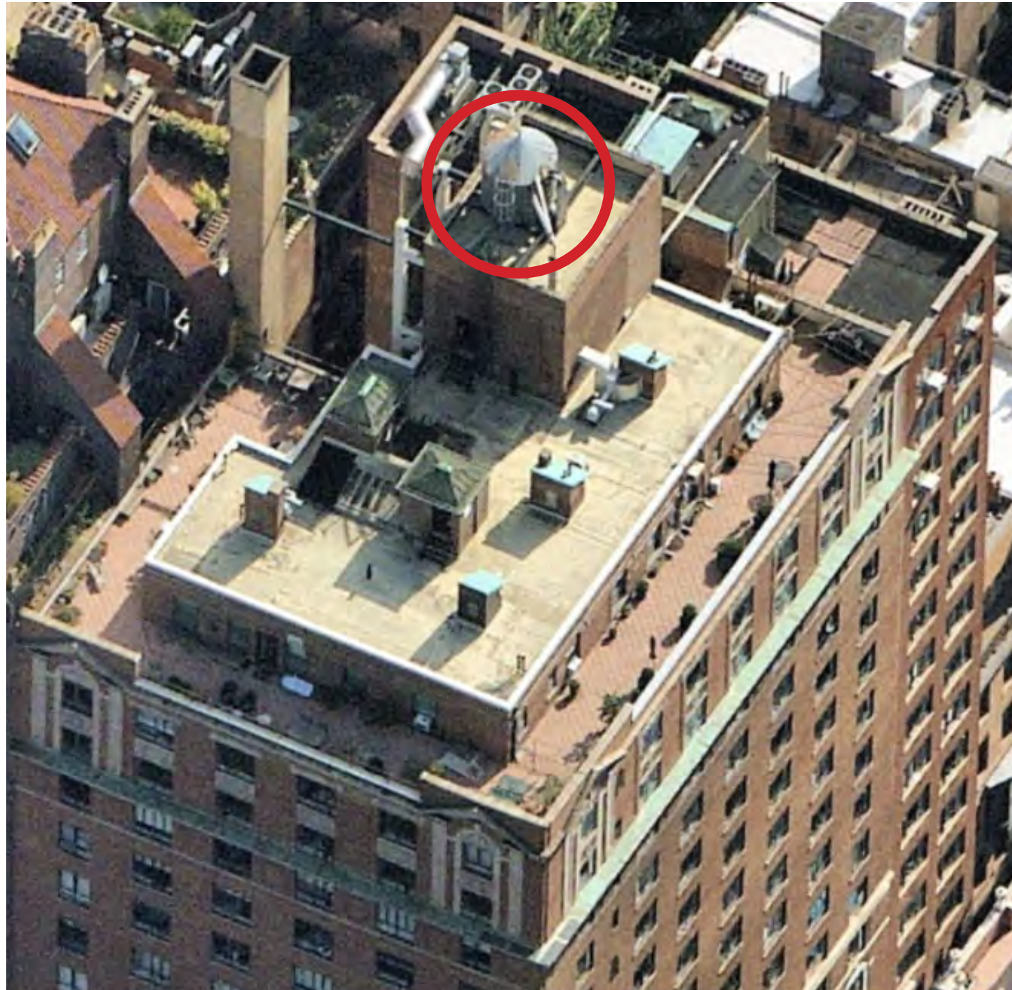
AERIAL VIEW OF ROOF - VIEW TO NORTHEAST
