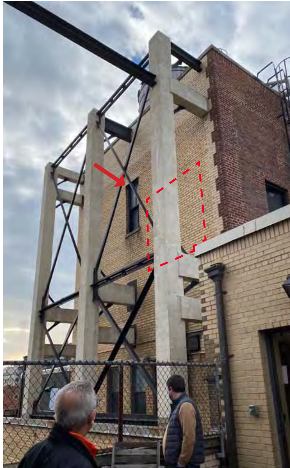
NORTH ELEVATION OF TANK HOUSE
