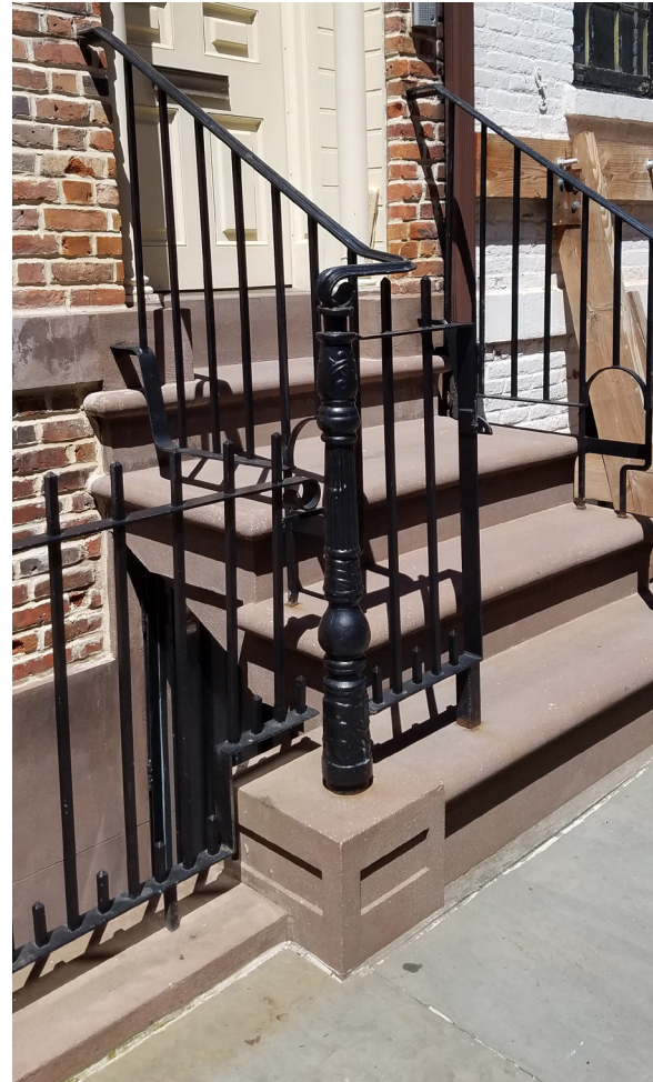
12 GAY STREET EXISTING CELLAR GATE
