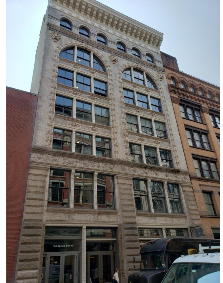
Spring Street elevation, September 2021.
