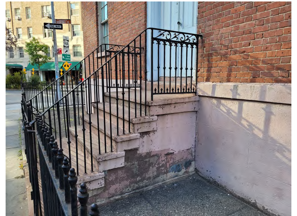
[Figure 18] West Facade, Area of Proposed Work, Main Entrance Stoop
