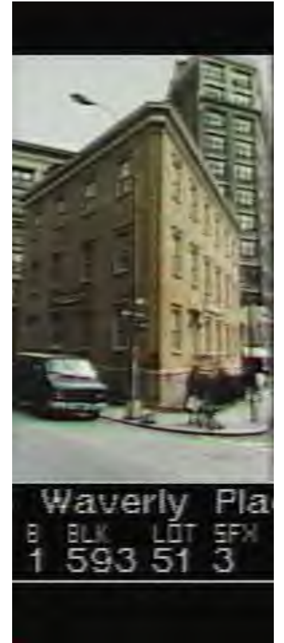
[Figure 09] Tax photo of north and west facades, 1980s. Christopher Street running to the left.
