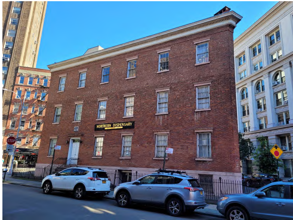
[Figure 10] West Facade
