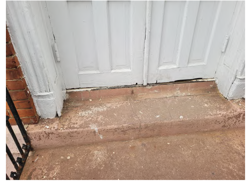
[Figure 21] Main Entrance Steps at Building
