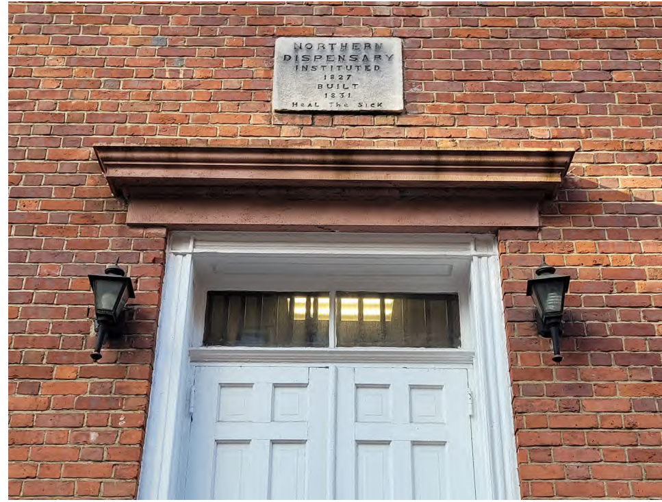
[Figure 20] Main Entrance Lintel, Door and Paneled Jamb
