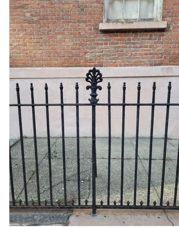
[Figure 27] Wrought Iron Fence Around Building
