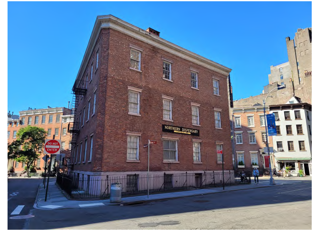
[Figure 12] North Facade
