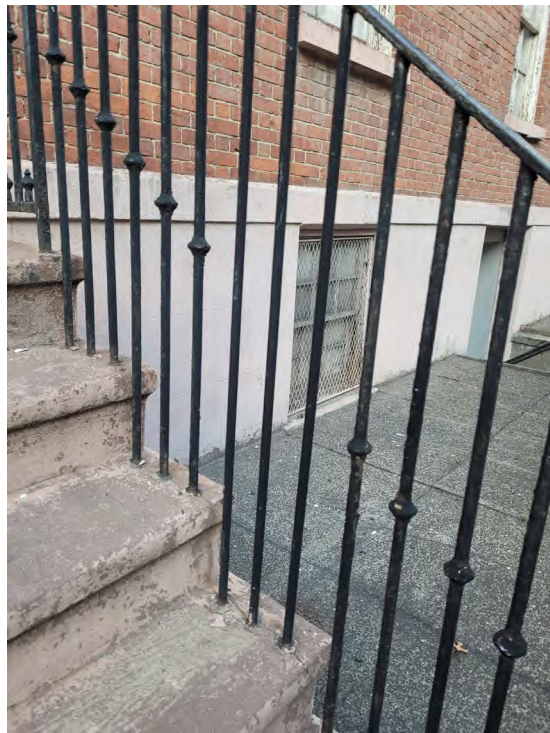
[Figure 22] Angled Railing at Stairs
