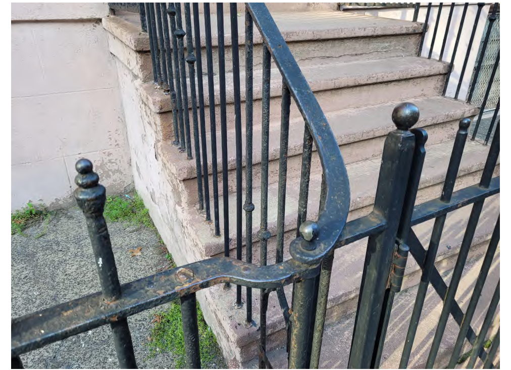
[Figure 24] Curved Handrail Transition into Wrought Iron Fence
