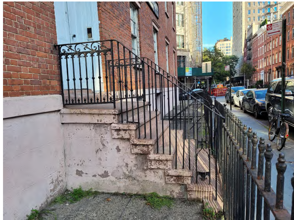
[Figure 17] West Facade, Area of Proposed Work, Main Entrance Stoop
