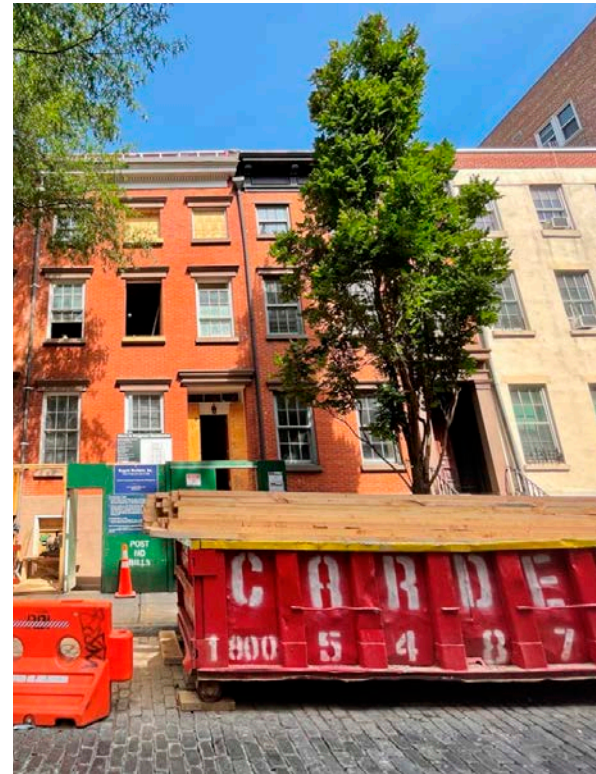
2. View of Front Facade & Adjacent Building
