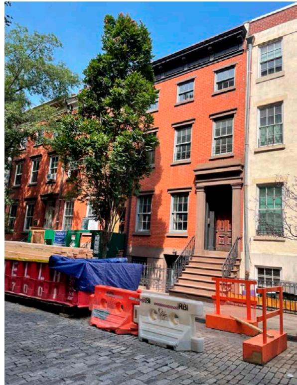
1. View of Front Facade
