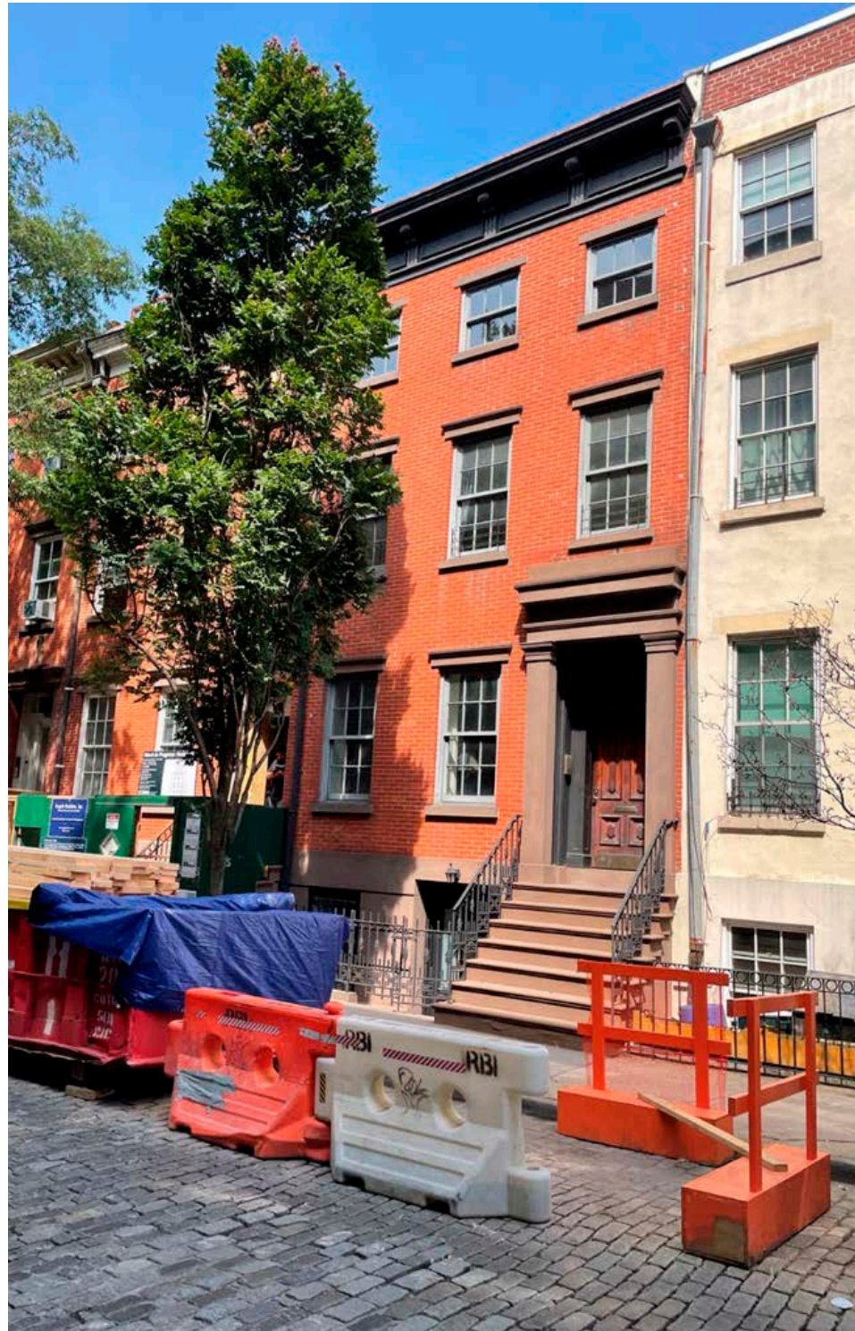
107 Bank - Current Street Facade
