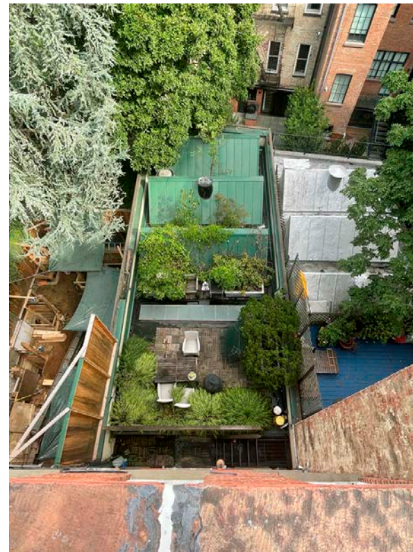
6. View of Rear Exterior from Roof
