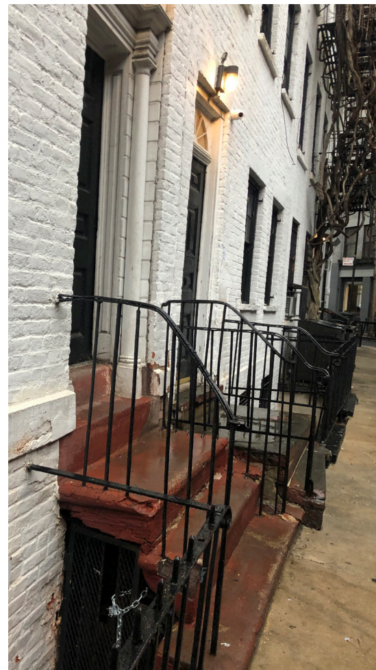
16 GAY STREET EXISTING CELLAR GATE
