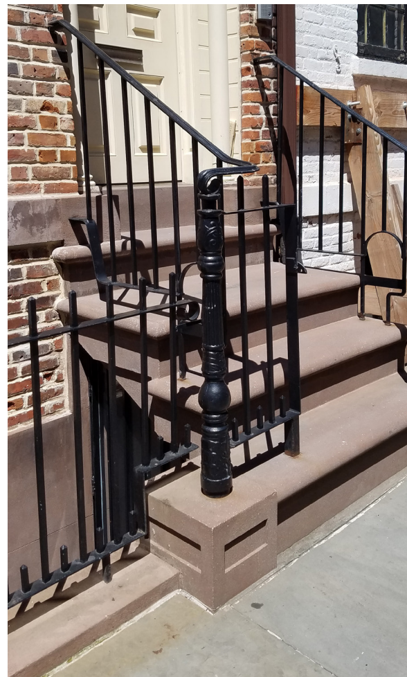
12 GAY STREET EXISTING CELLAR GATE
