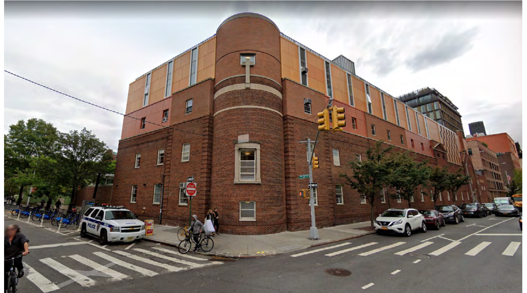
Existing conditions. View looking southeast at intersection of Greenwich and Christopher streets.
