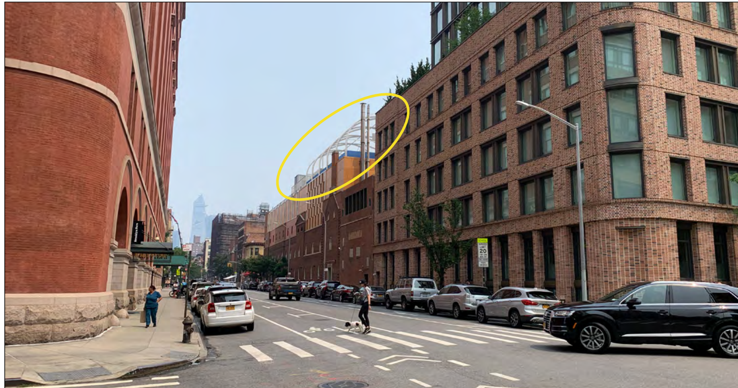
Photo collage - playcage, guardrail, exterior stair, mechanical flues, and wall safety pads are visible.
