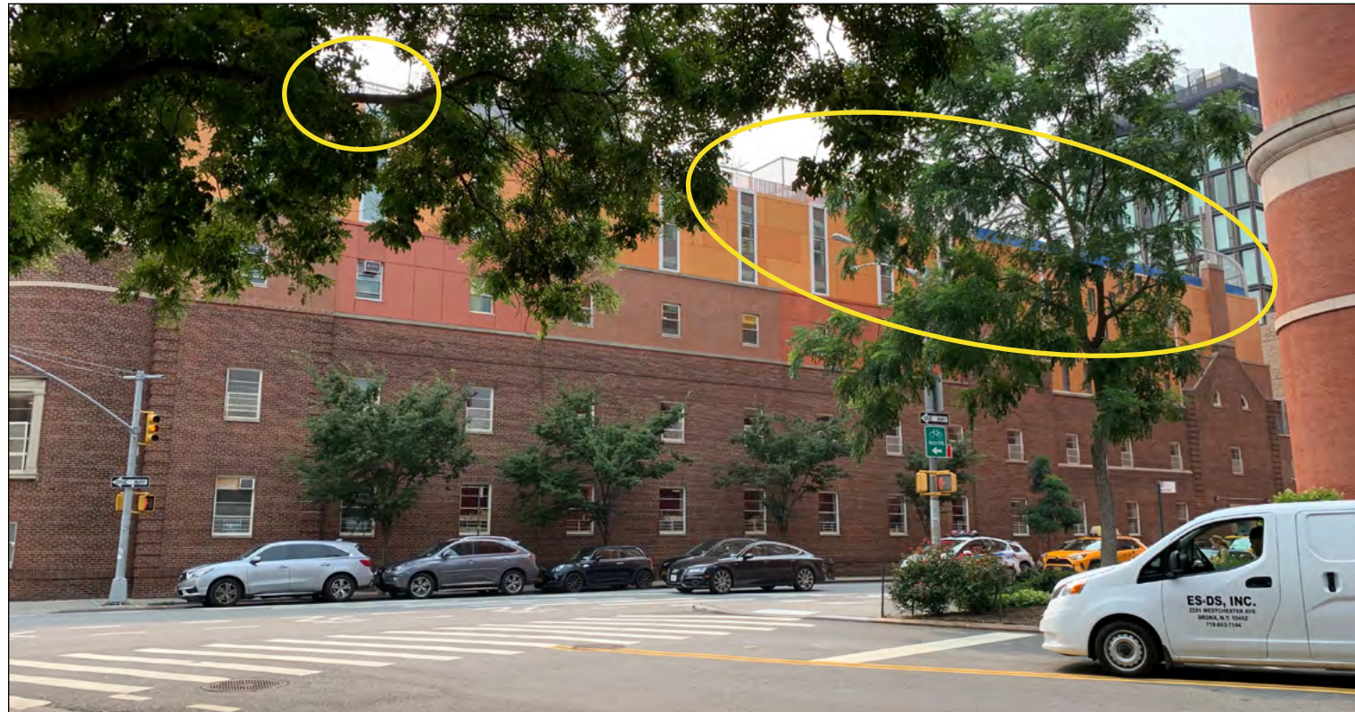
Photo collage - guardrail, playage, wall safety pads, and mechanical flues are visible.
