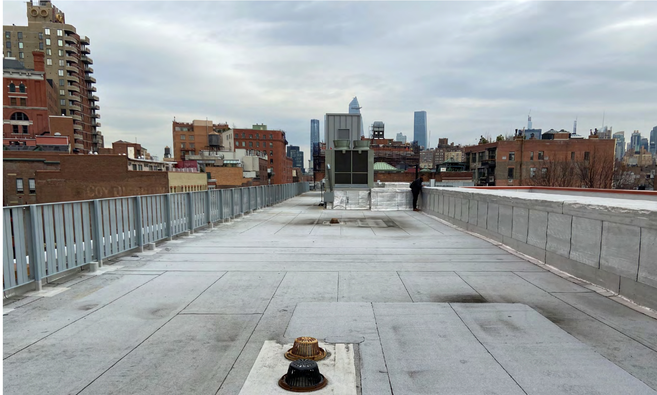
Existing condition at roof, main school building. View looking north.
