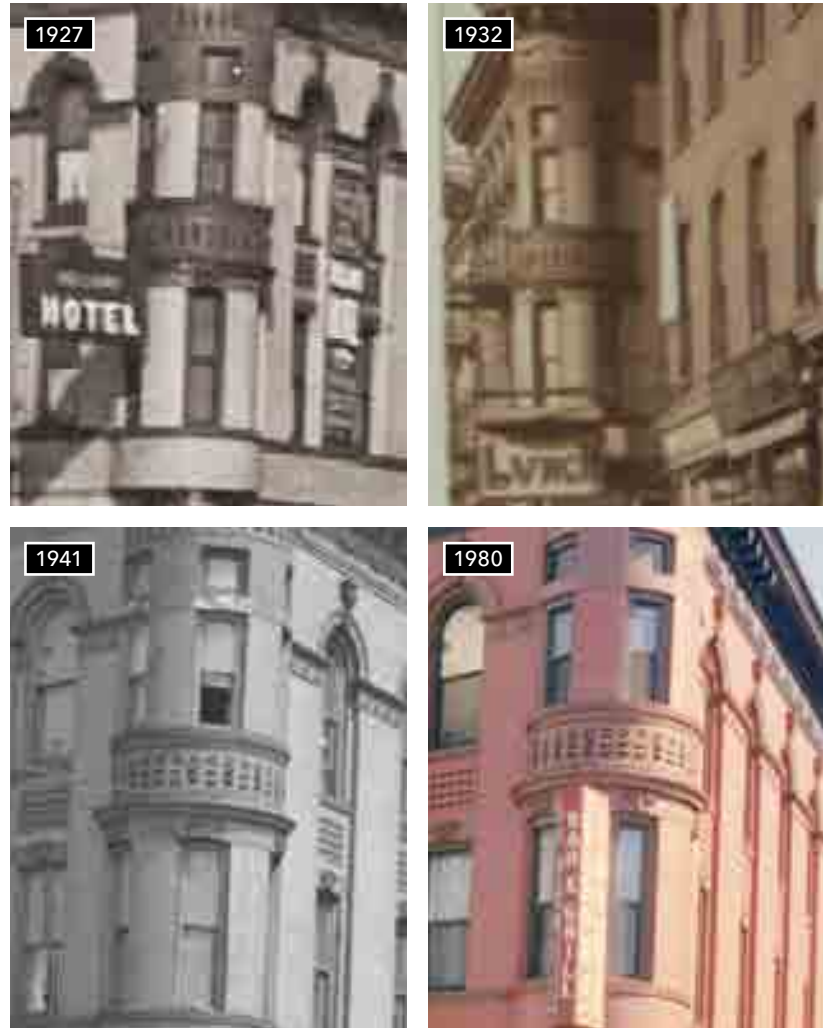
Historic Hung Window: W2-Historic (Photo)
