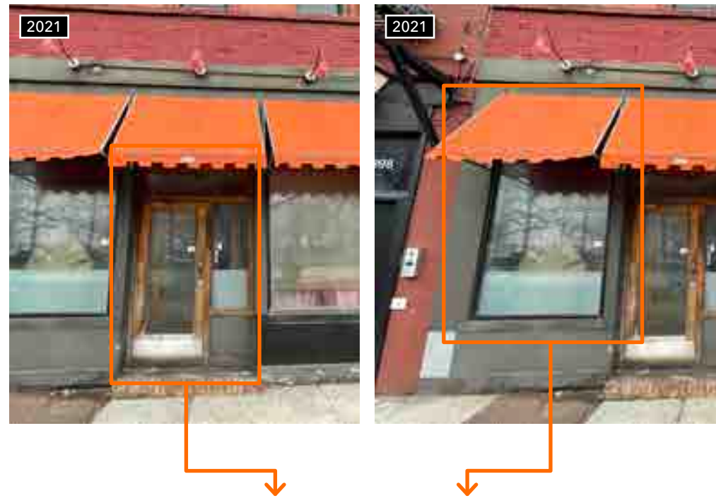
Existing Entrance Existing Storefront
