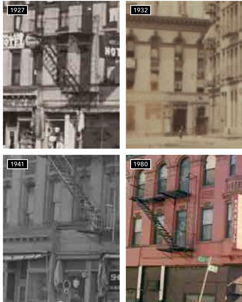
Historic Hung Window: W1-Historic (Photo)
