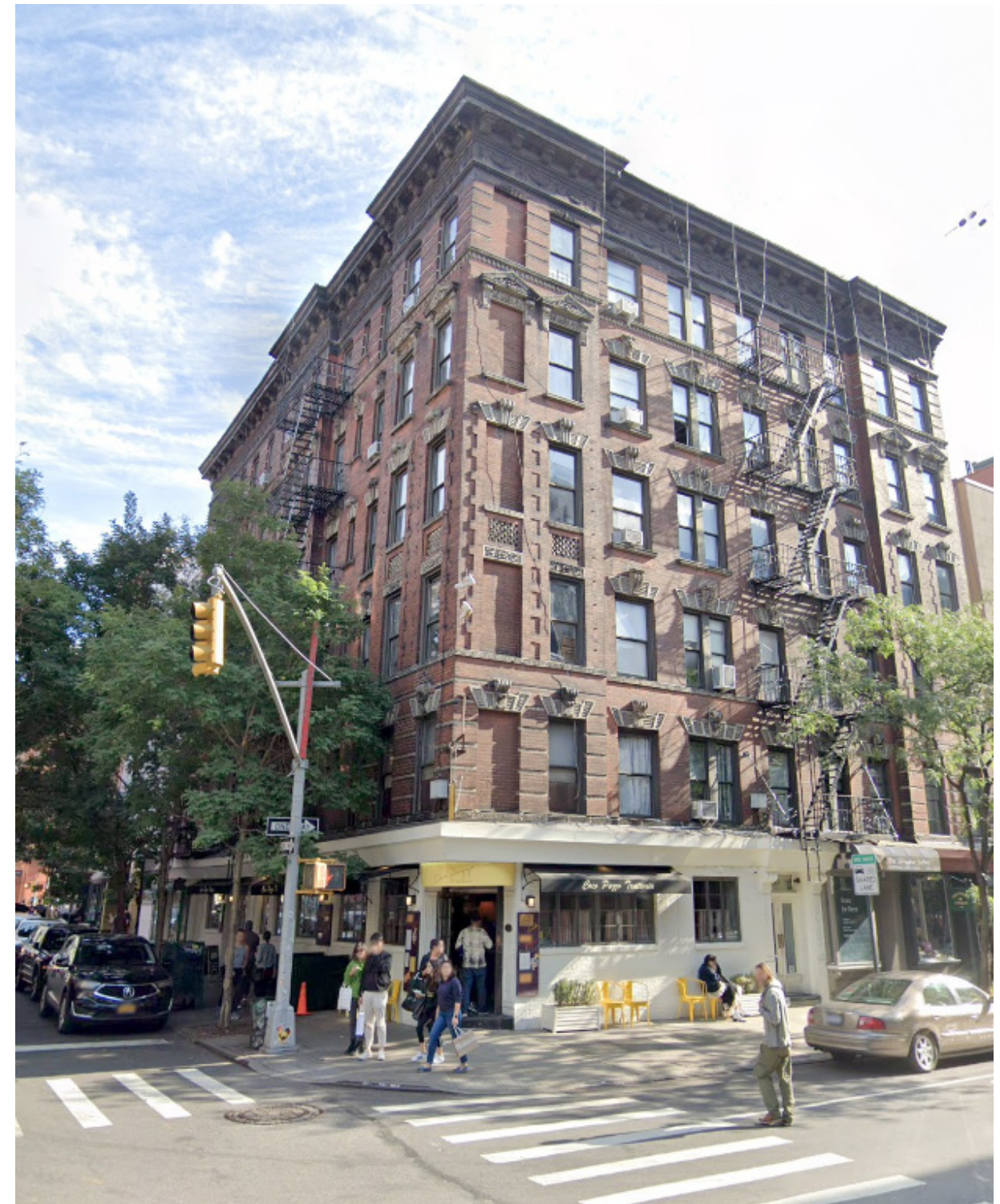
160 PRINCE STREET - SOUTH WEST CORNER AT INTERSECTION OF THOMPSON ST AND PRINCE ST
