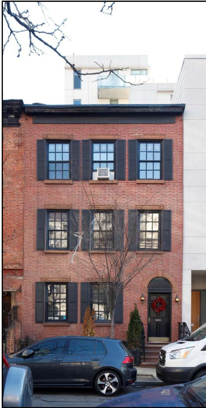
ROW HOUSES 57 SULLIVAN STREET
