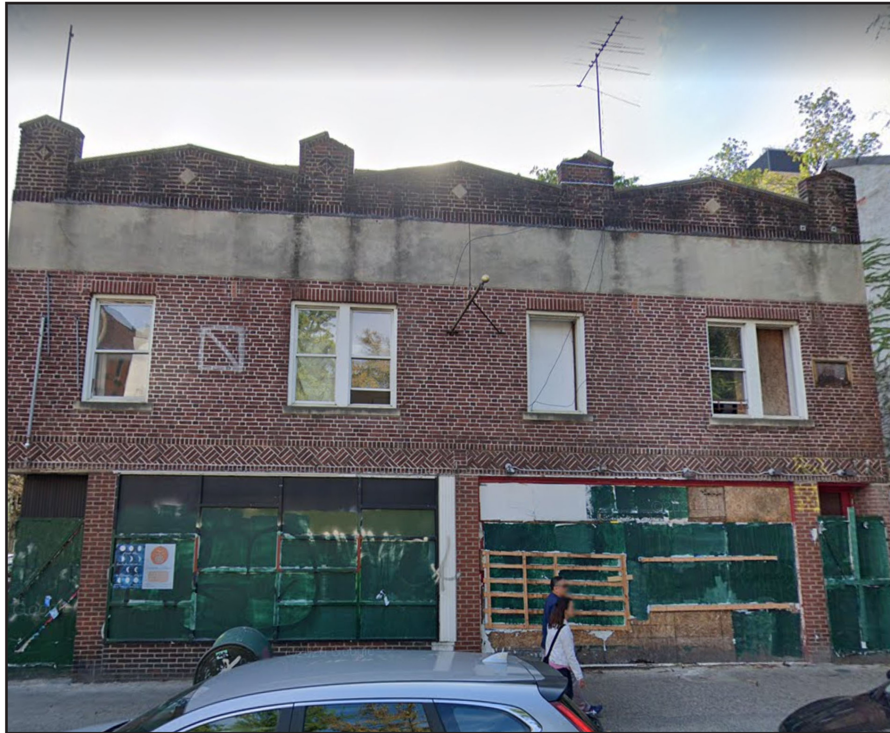
CURRENT: NORTH FACADE
