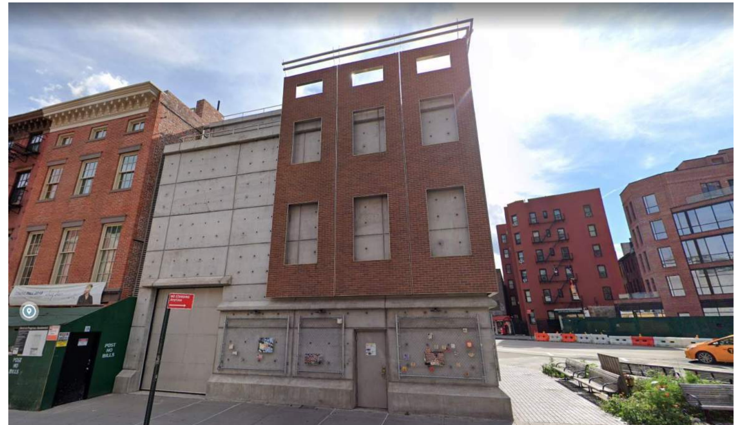
61 Greenwich Ave - Completed 2014
