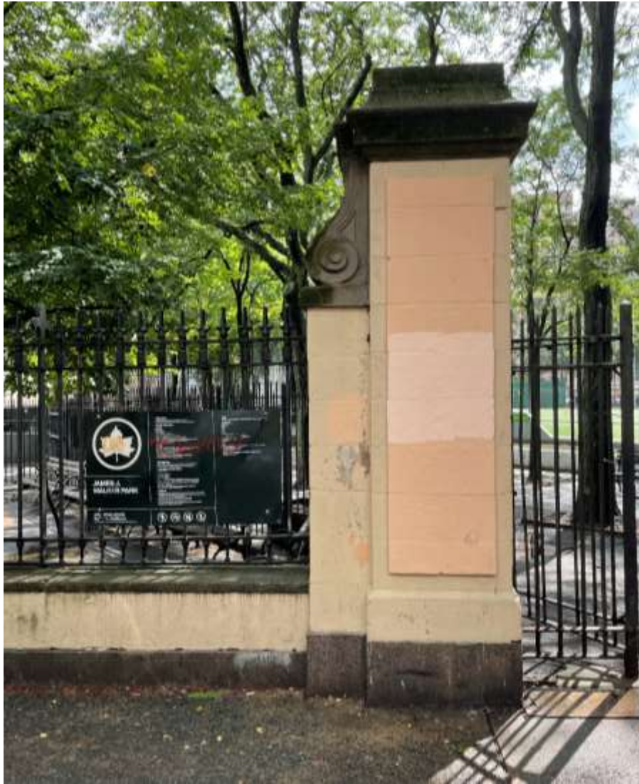
1 – Gate pier at JJ Walker Park– painted/ material unknown, granite base, limestone cap, historic iron fence, modern iron gate
