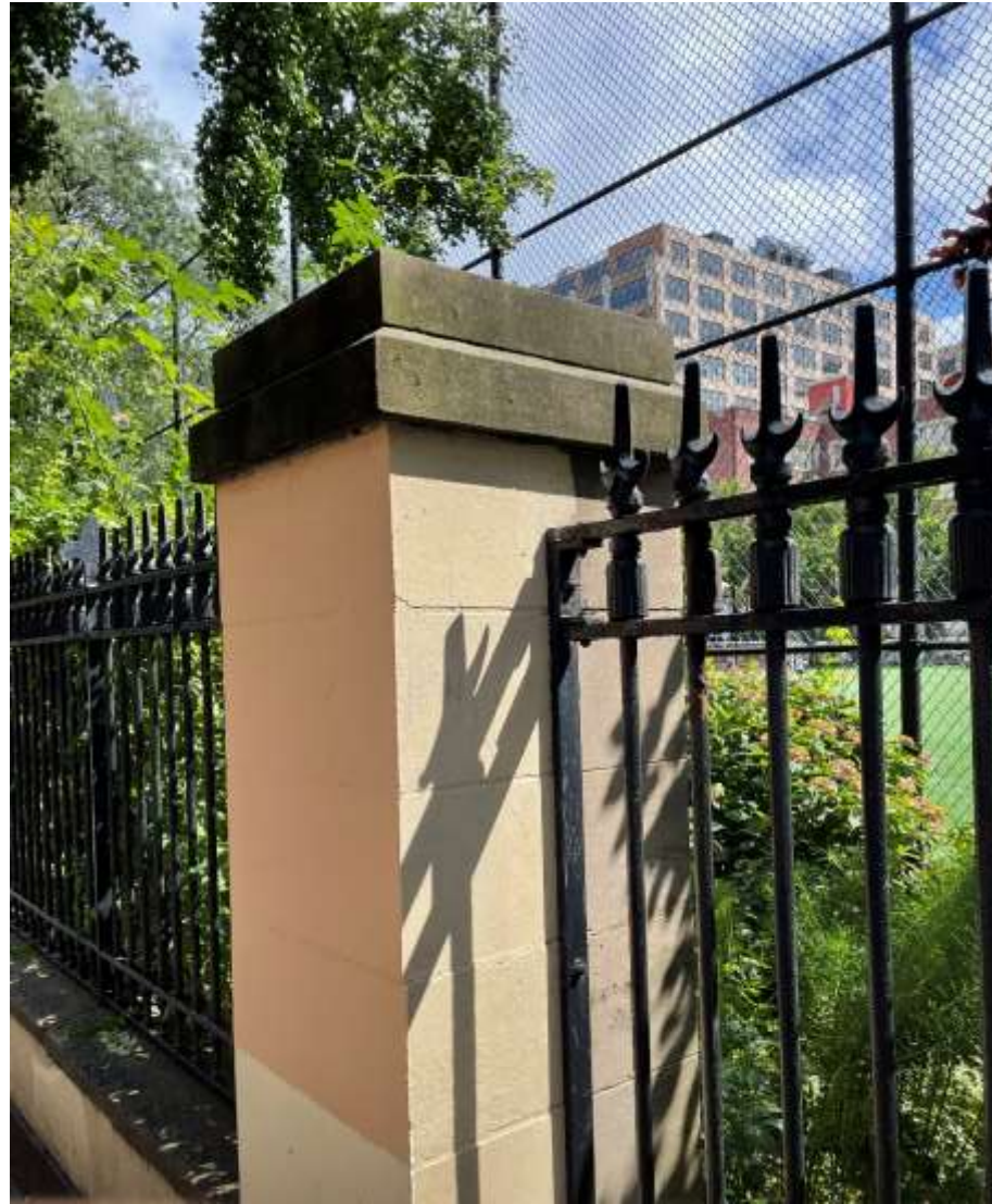
2 – Secondary pier at JJ Walker Park fence – painted/ material unknown, granite base, limestone cap, skirted ranseur fence pickets
