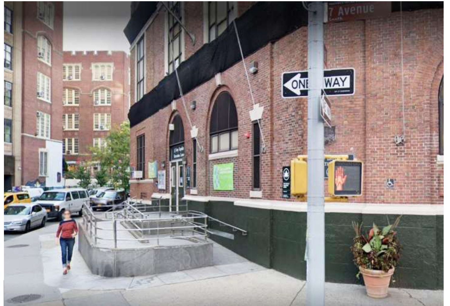
Existing Stair & Ramp - 1982
