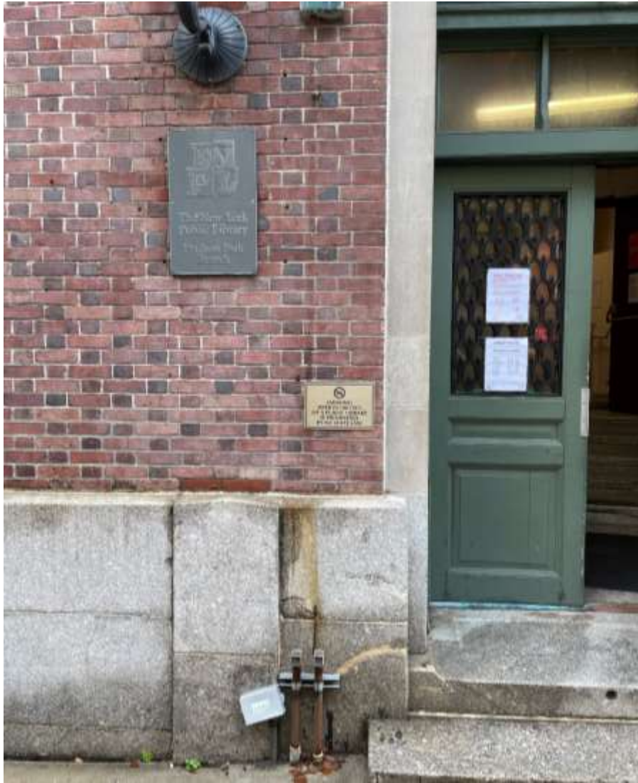
1 – Leroy St. library entrance – granite skirt and steps, limestone banding
