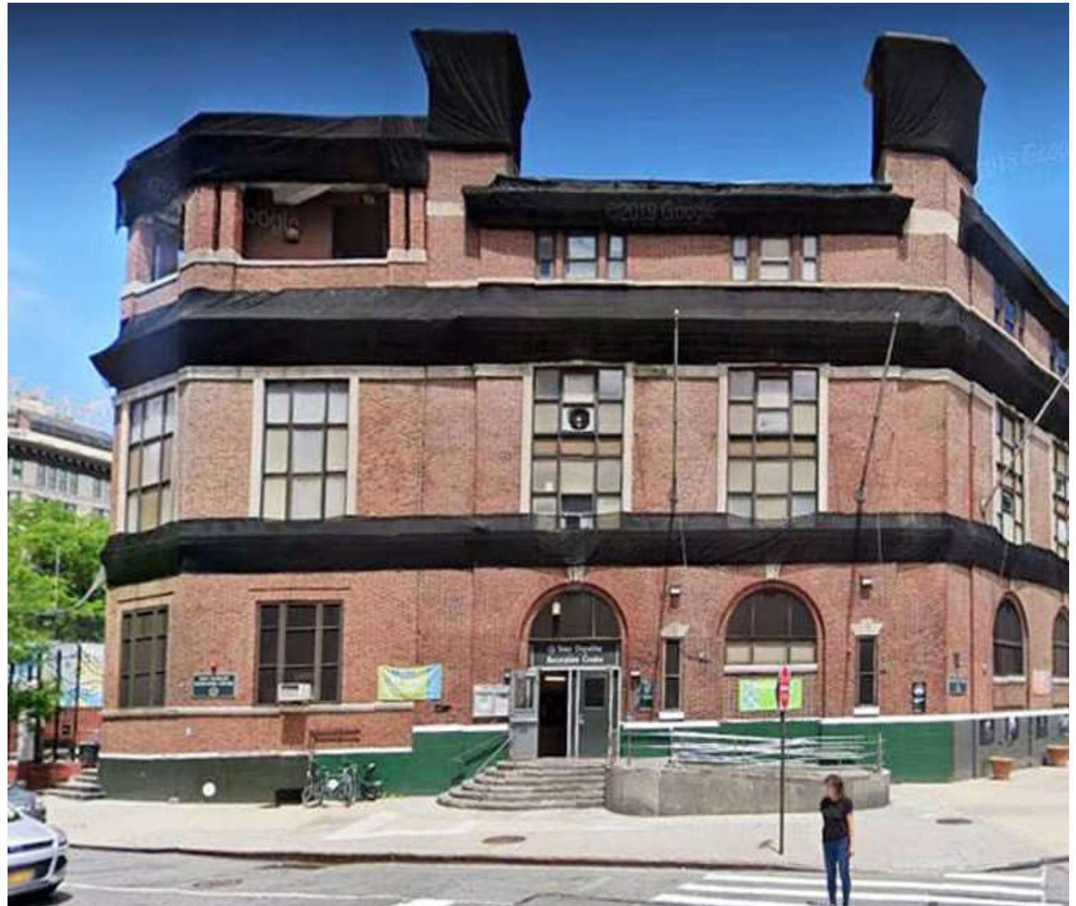
Existing Clarkson Façade
