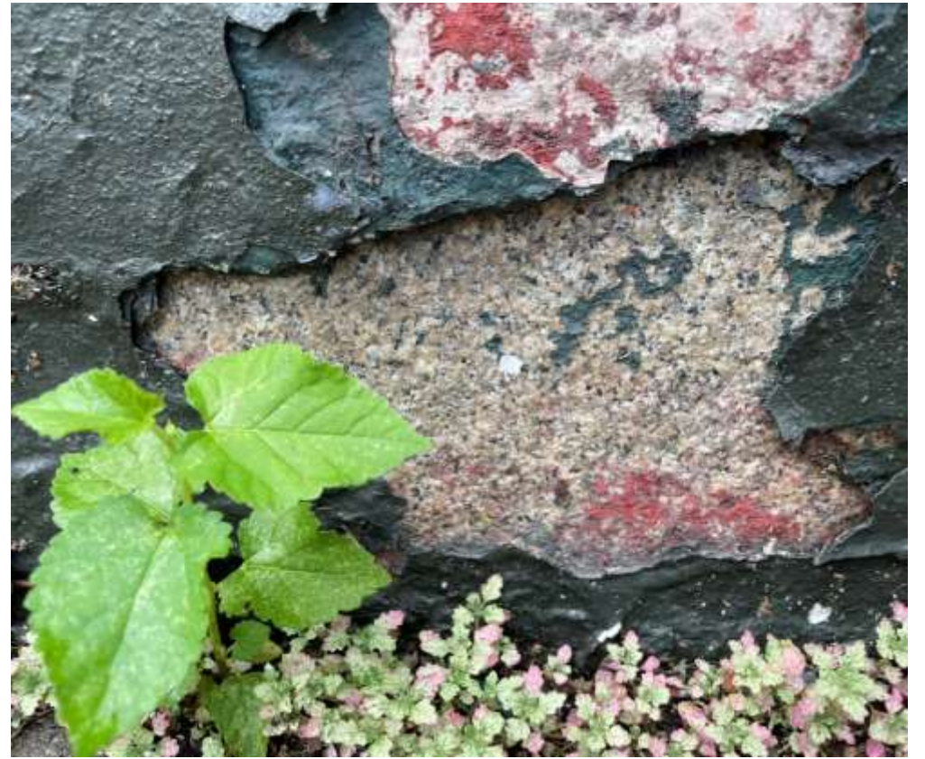
3 – granite building base closeup
