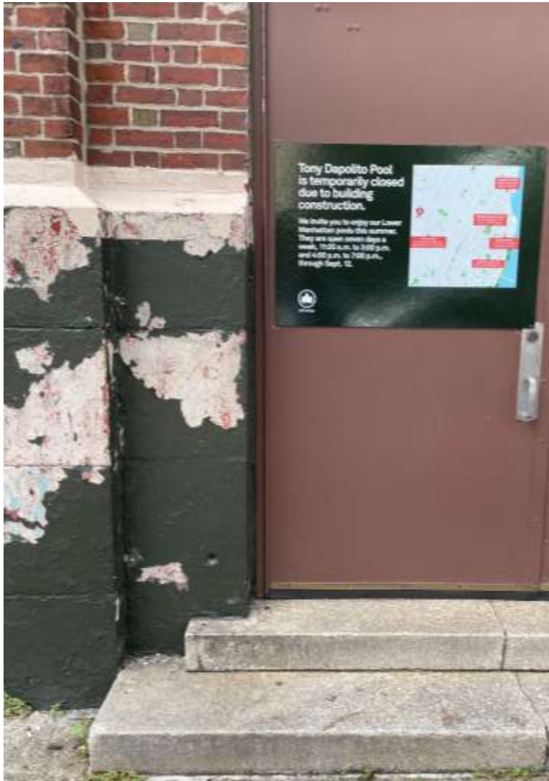
1 – 7 th Avenue egress – granite steps, painted granite skirt
