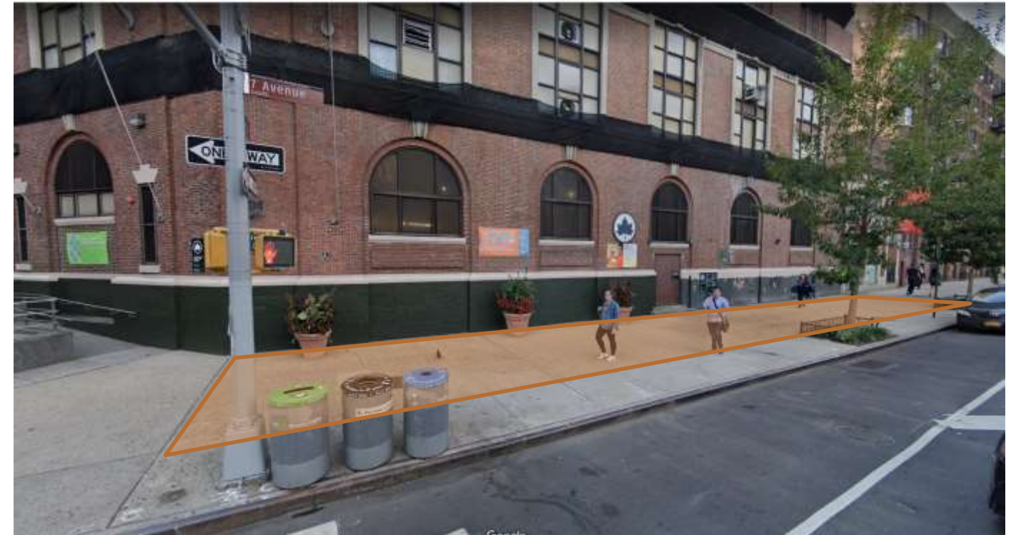
2 – 7 th Ave frontage showing extent of sidewalk vault
