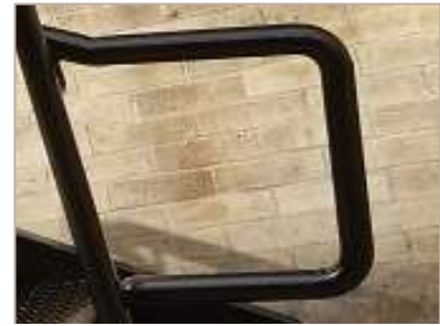
Black steel pipe handrail. Color to match existing fence at Center and adjacent park
