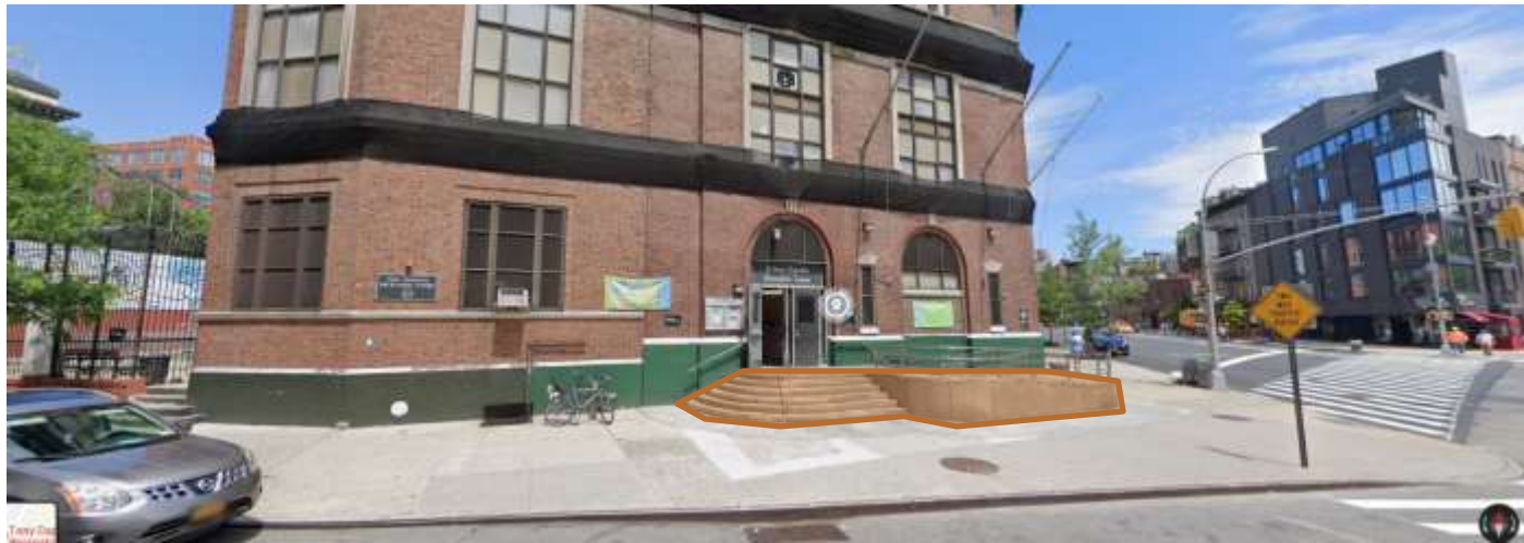
1 – Clarkson frontage showing steps and ramp to be replaced
