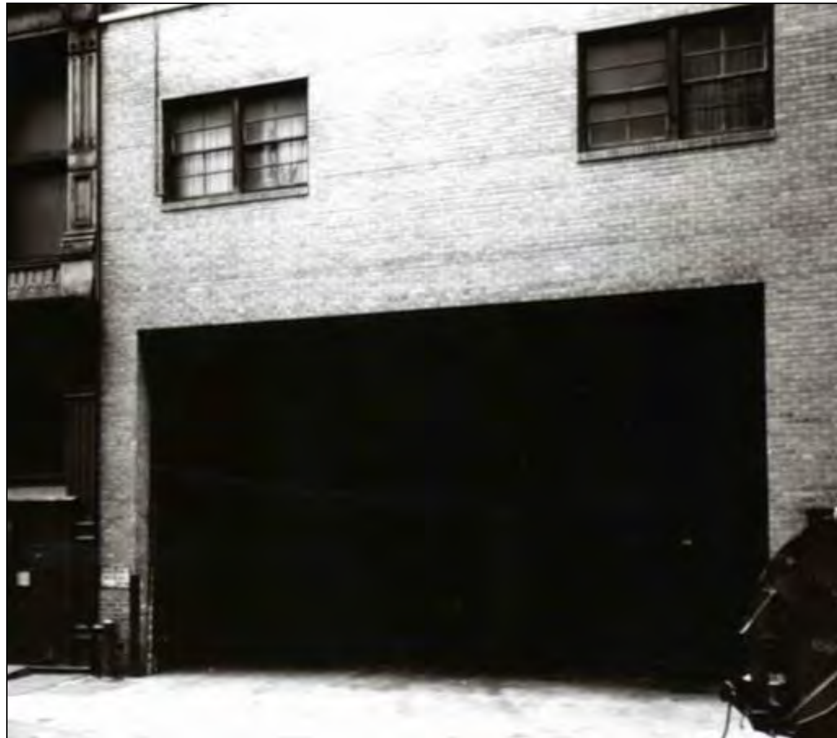
101 Greene Street, c.1971 (LPC Designation Photo)
