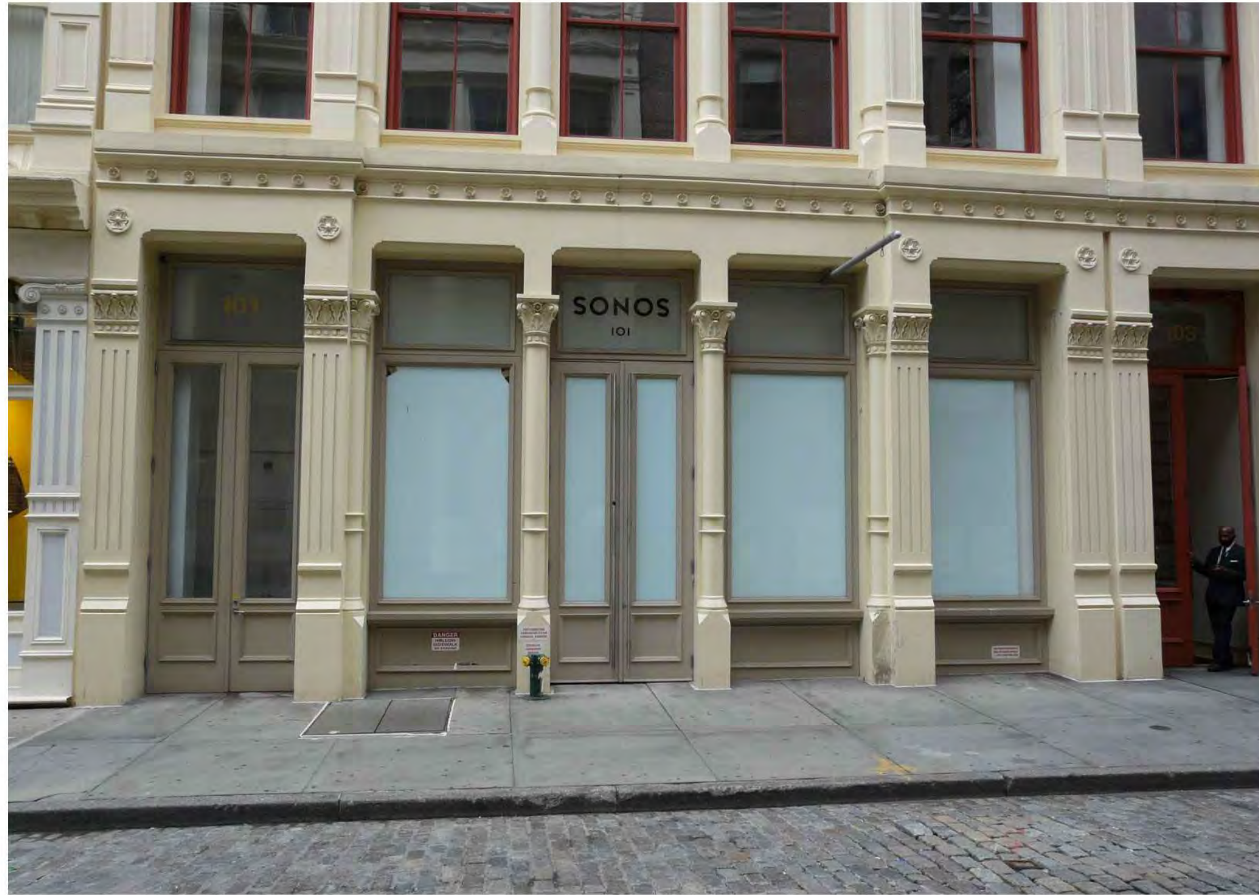
1 EXISTING STOREFRONT CONDITION
