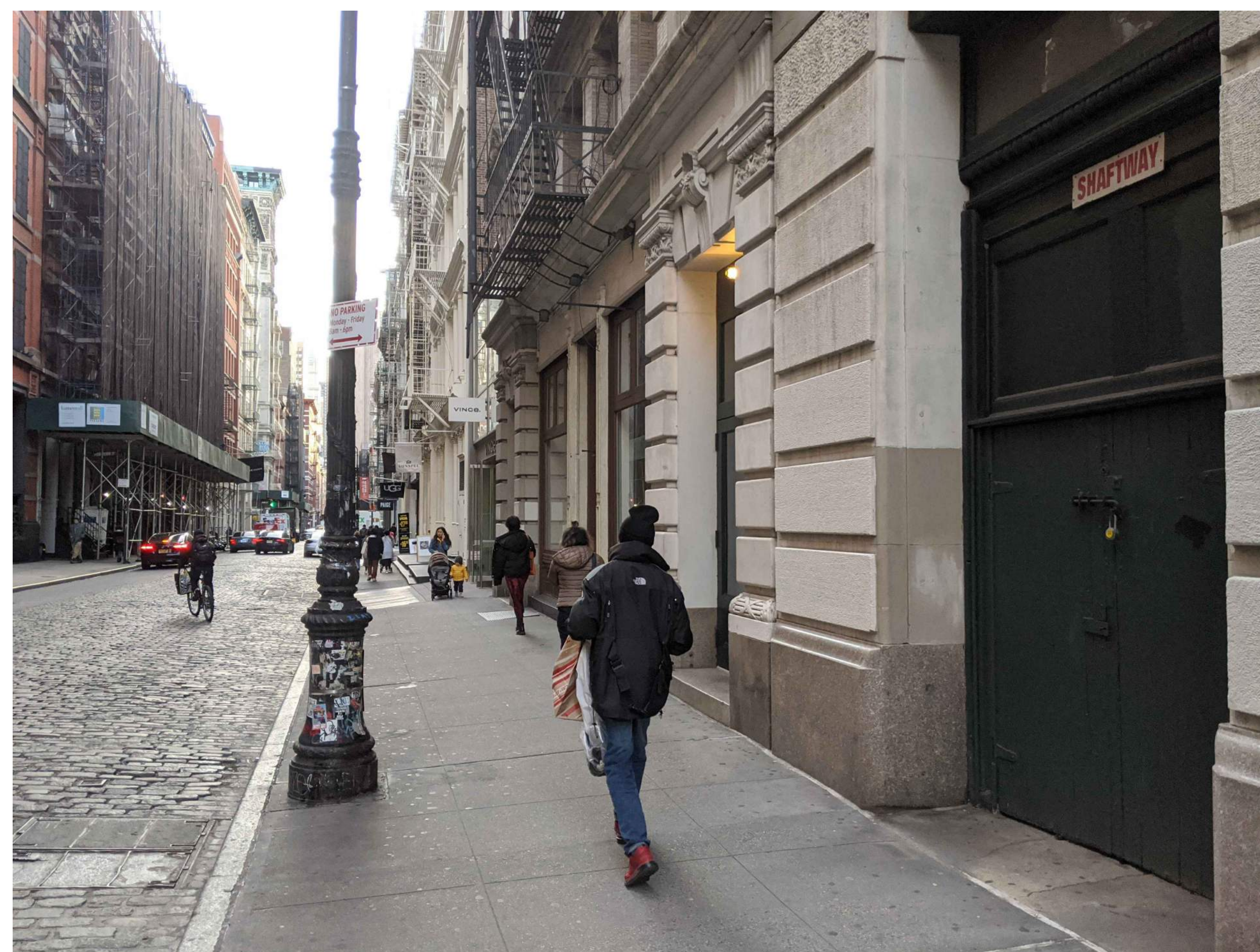
PHOTO 6: CURRENT PHOTO FACING SOUTH OF THE WEST (MERCER STREET) FACING PRIMARY ELEVATION.
