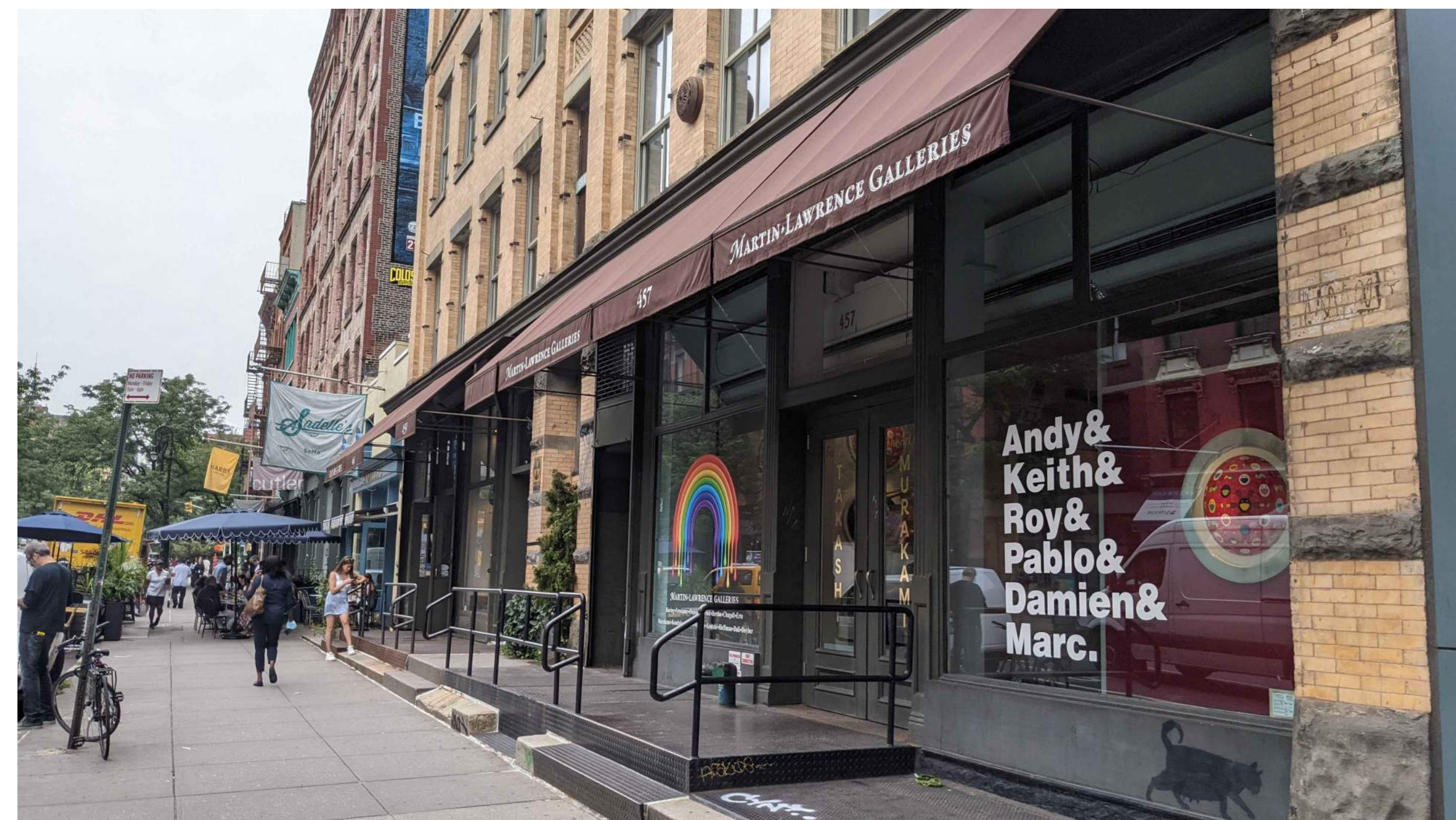
PHOTO 16: CURRENT PHOTO FACING NORTH AT 457 WEST BROADWAY DISPLAYING A LONG STEPPED LANDING WITH RAILINGS .
