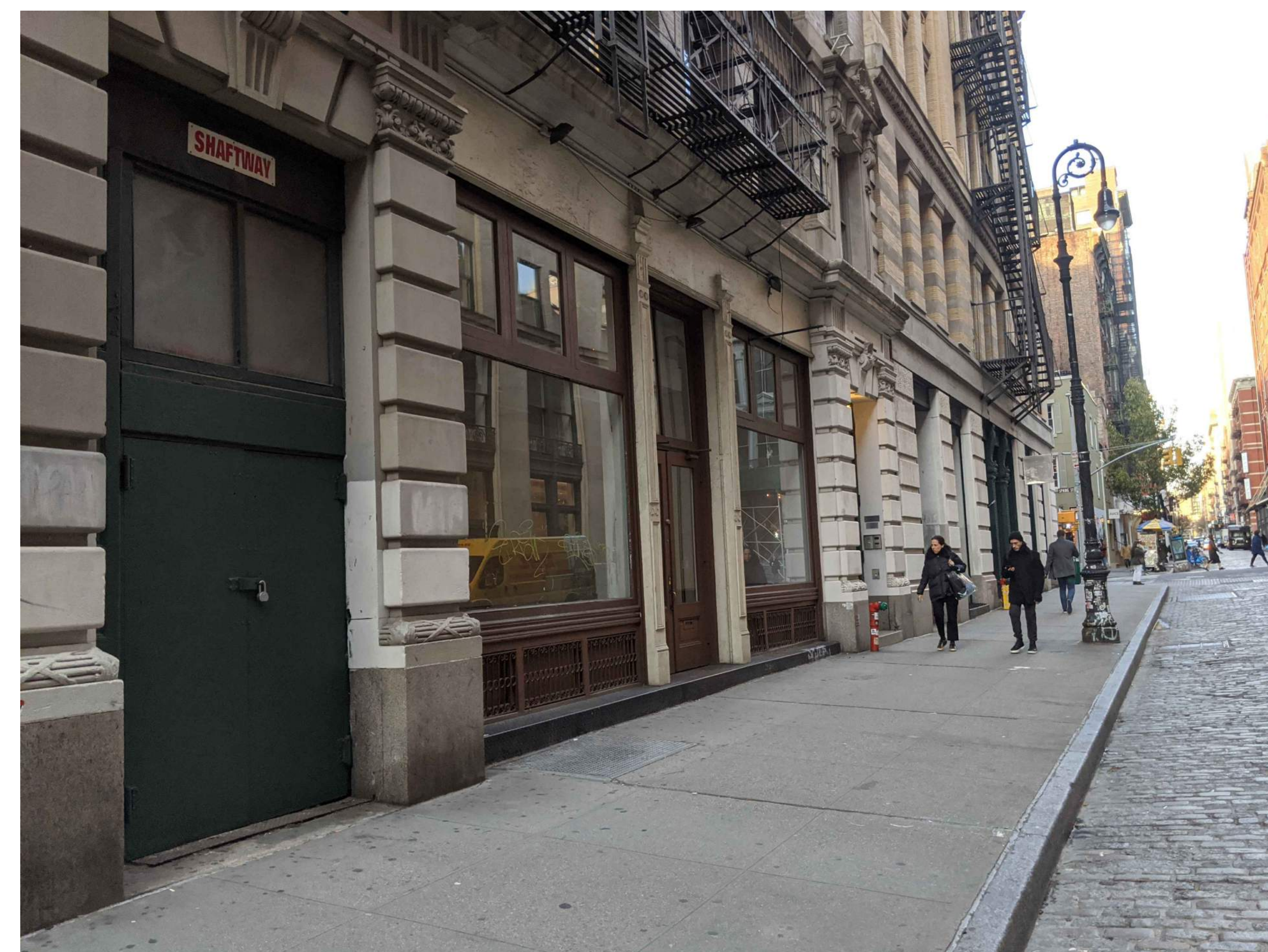
PHOTO 7: CURRENT PHOTO FACING NORTH OF THE WEST (MERCER STREET) FACING PRIMARY ELEVATION.
