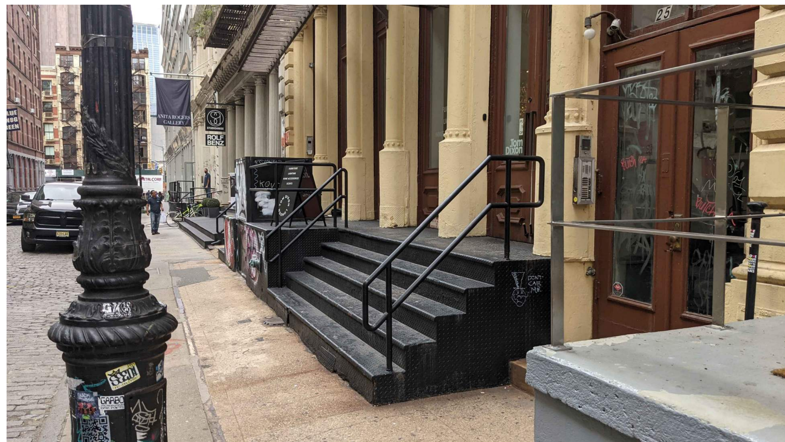
PHOTO 15: CURRENT PHOTO FACING SOUTH AT 25 GREENE STREET DISPLAYING A LONG STEPPED STOOP WITH RAILINGS.
