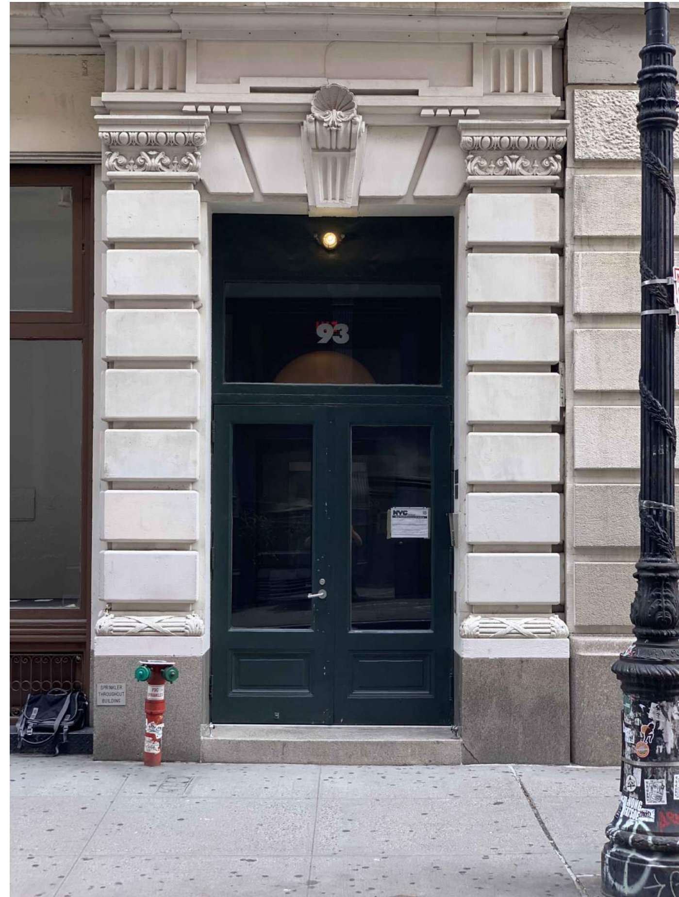
PHOTO 8: CURRENT PHOTO OF THE EXISTING DOUBLE DOOR ASSEMBLY ALONG THE WEST (MERCER STREET) FACING PRIMARY ELEVATION, TO BE REMOVED AND REPLACED WITH A NEW ADA-COMPLIANT DOOR ASSEMBLY DOOR ASSEMBLY TO MATCH DESIGN OF EXISTING DOOR IN STYLE AND FINISH. THE EXISTING STANDPIPE WILL BE RELOCATED AND THE EXISTING STEP WILL REMAIN.
