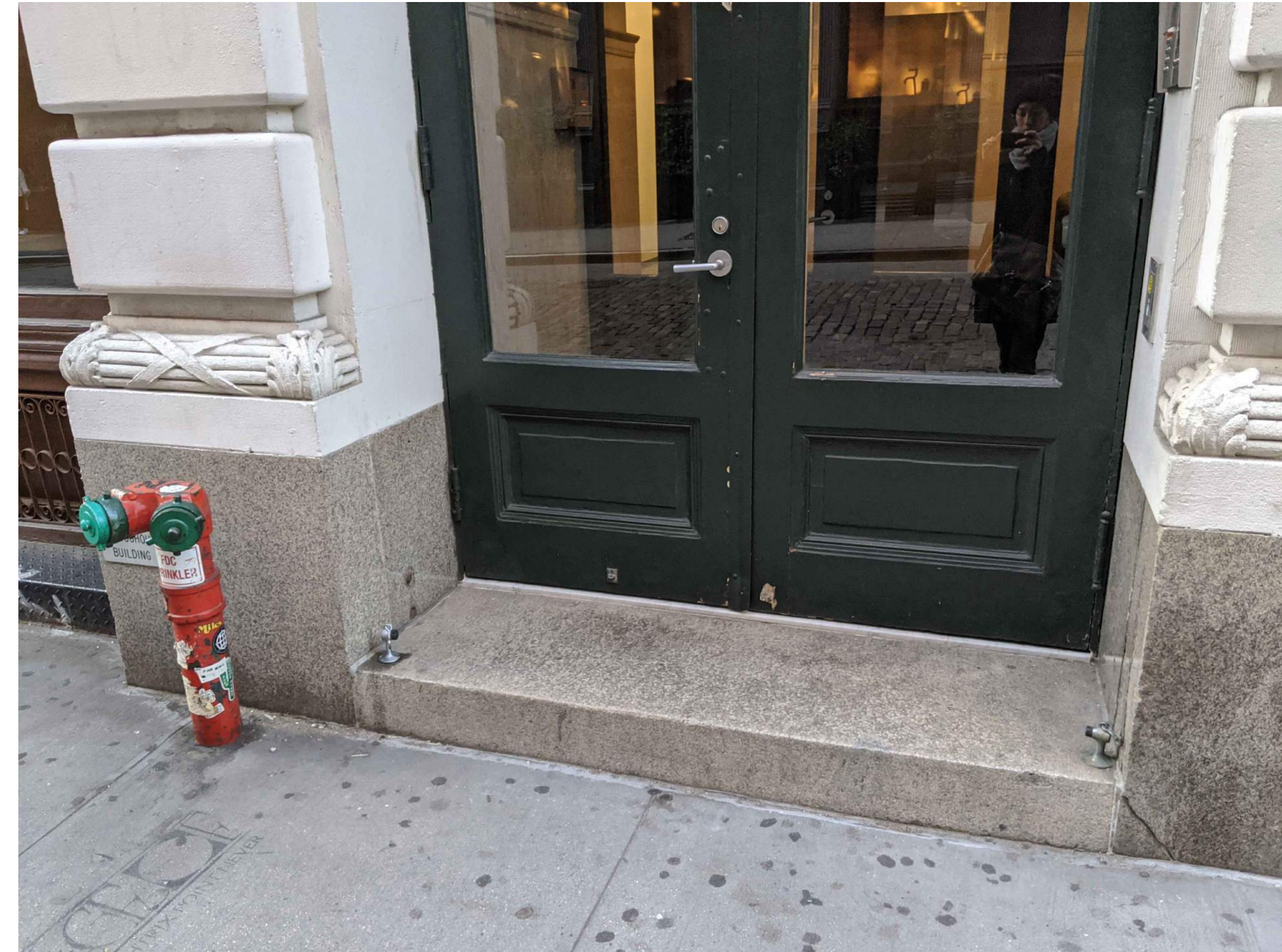
PHOTO 9: CURRENT PHOTO AT THE RESIDENTIAL ENTRANCE ALONG MERCER STREET. THE EXISTING STANDPIPE WILL BE RELOCATED AND THE EXISTING STEP WILL REMAIN.
