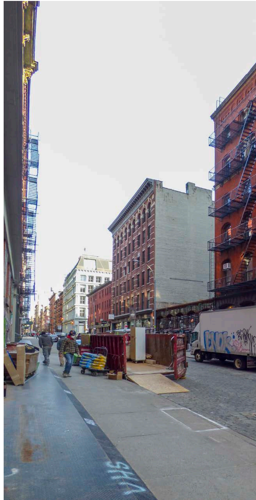
Existing view looking North on Crosby Street, between Grand Street and Howard Street
