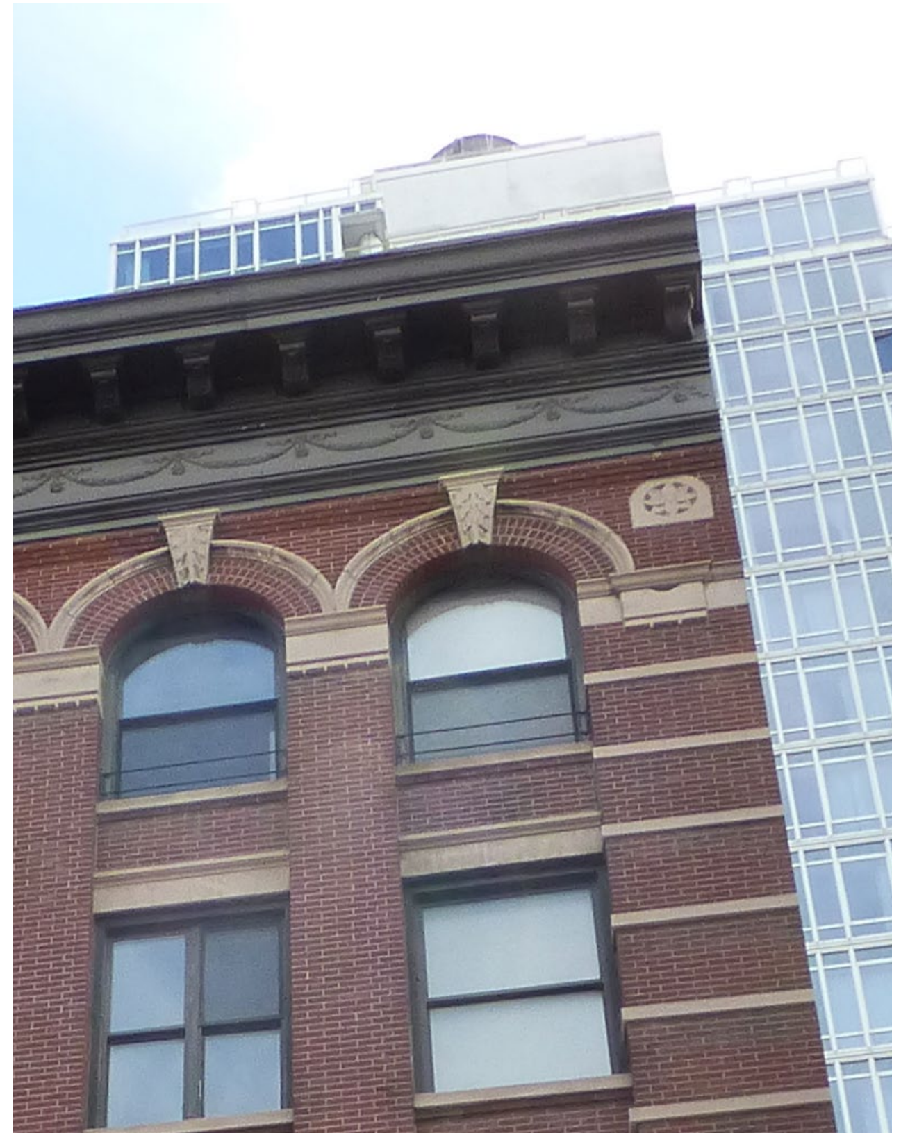
DETAIL VIEW OVER THE PRIMARY FACADE, LOOKING EAST, SHOWING NO VISIBILITY.
