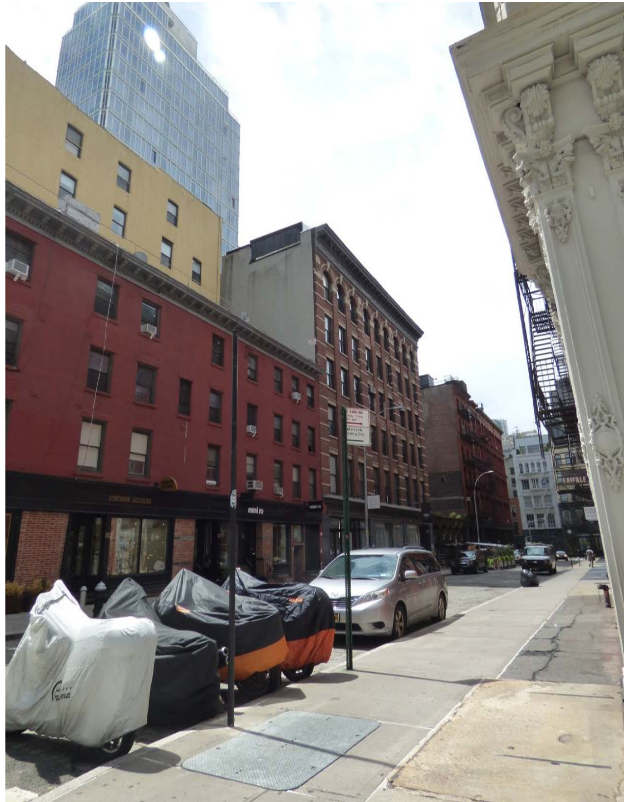
VIEW FROM THE CORNER OF CROSBY AND GRAND, SHOWING NO VISIBILITY.
