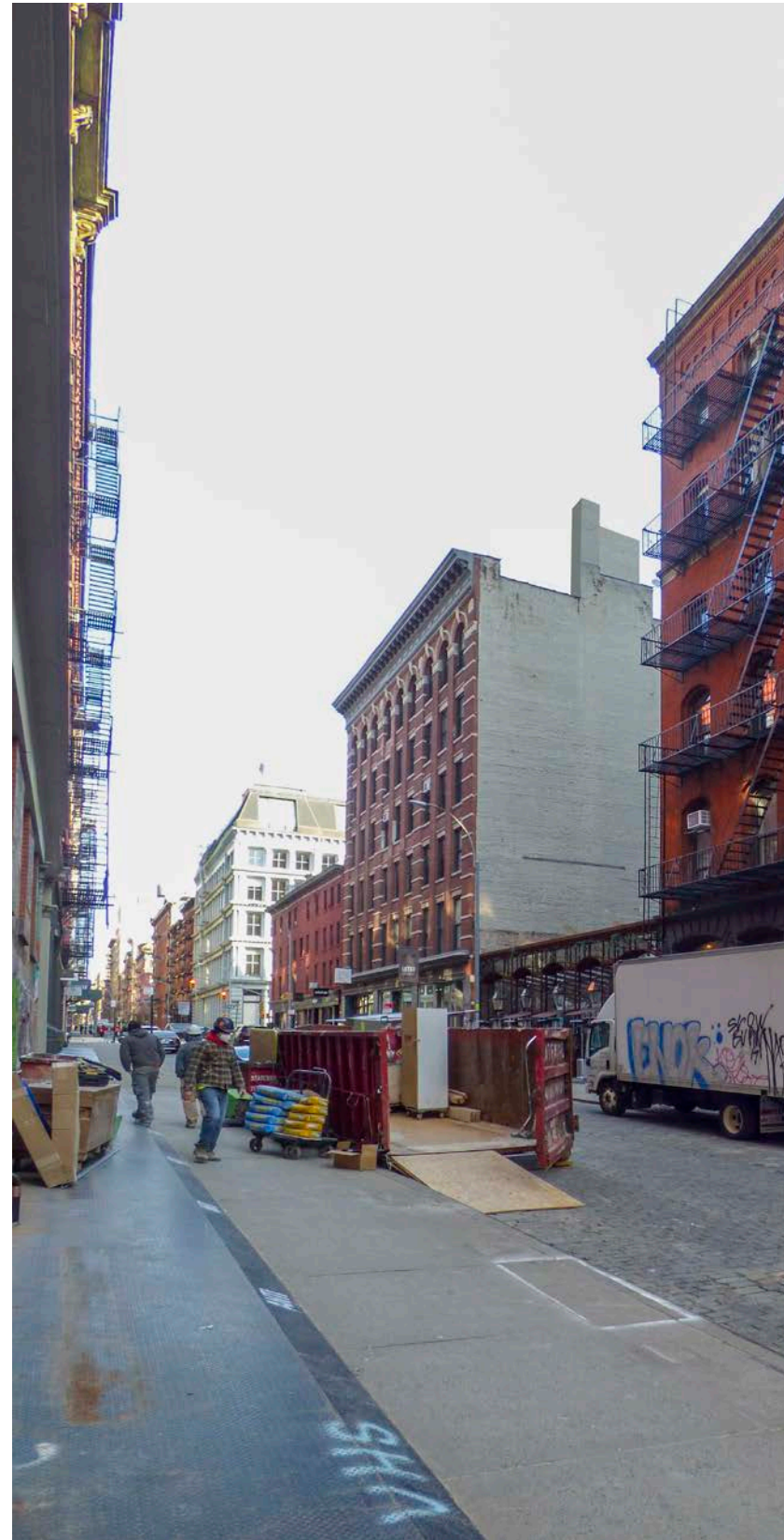
Proposed view looking North on Crosby Street, between Grand Street and Howard Street
