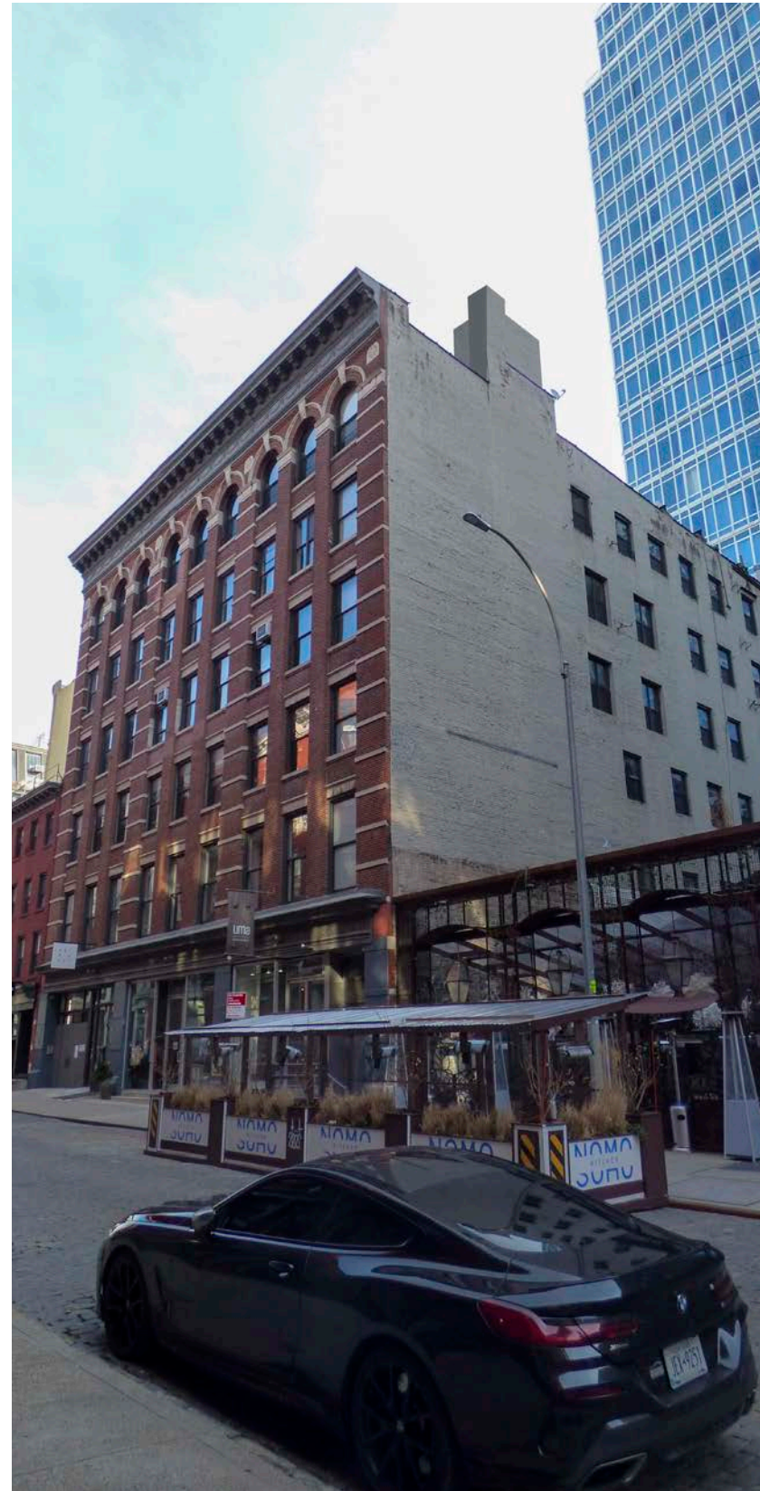
Proposed view looking North on Crosby Street, between Grand Street and Howard Street
