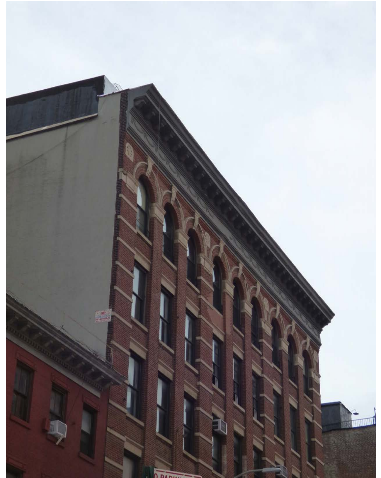
DETAIL VIEW FROM THE CORNER OF CROSBY AND GRAND, SHOWING NO VISIBILITY.
