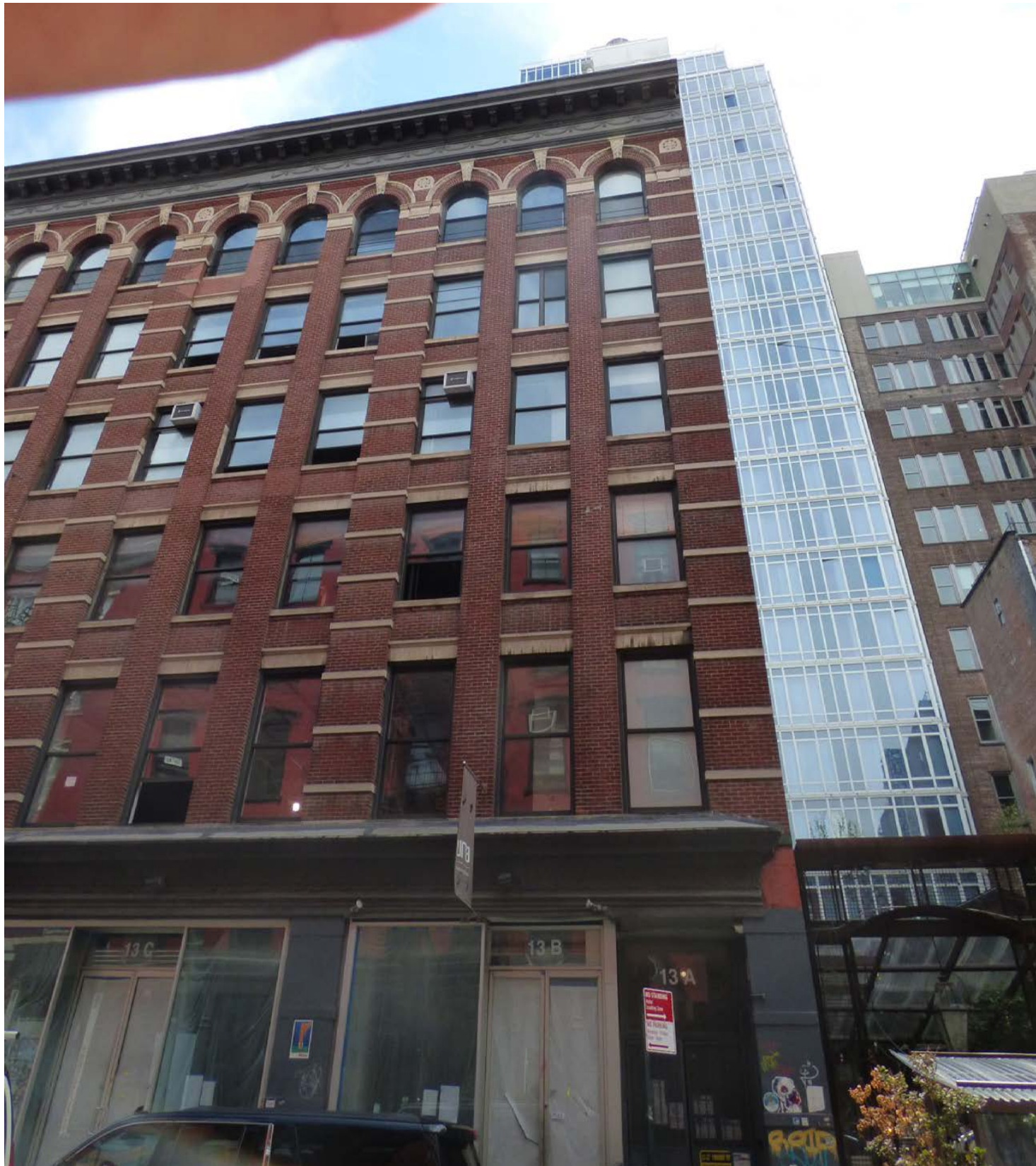
VIEW OVER THE PRIMARY FACADE, LOOKING EAST, SHOWING NO VISIBILITY.
