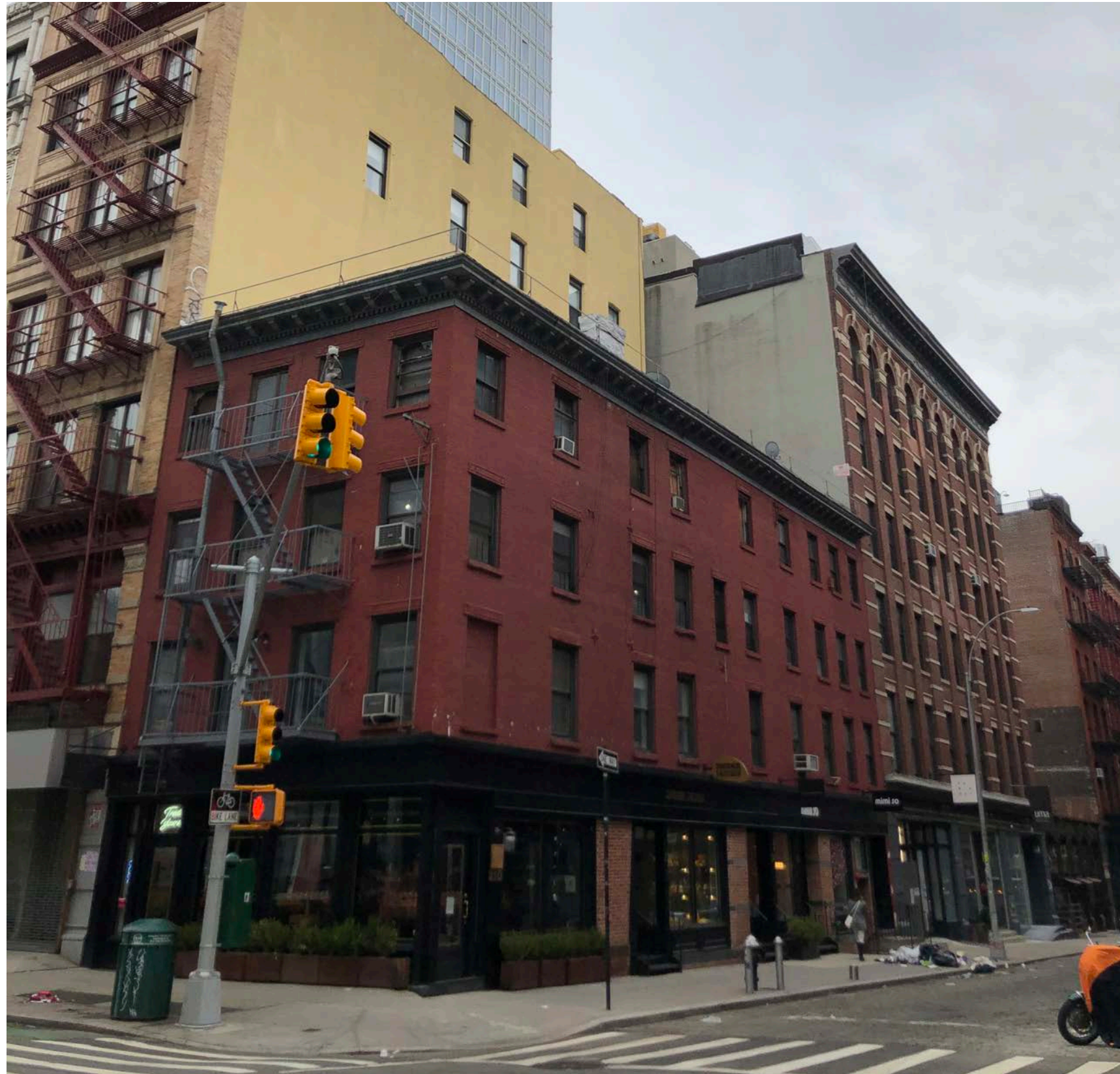
Bulkhead not visible looking south on Crosby Street, between Grand Street and Howard Street
